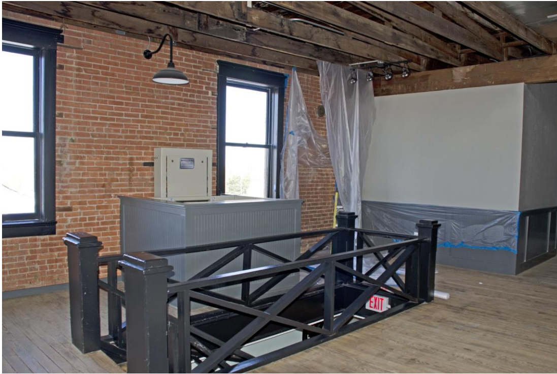
Photo 12 Original Lift, looking northeast
