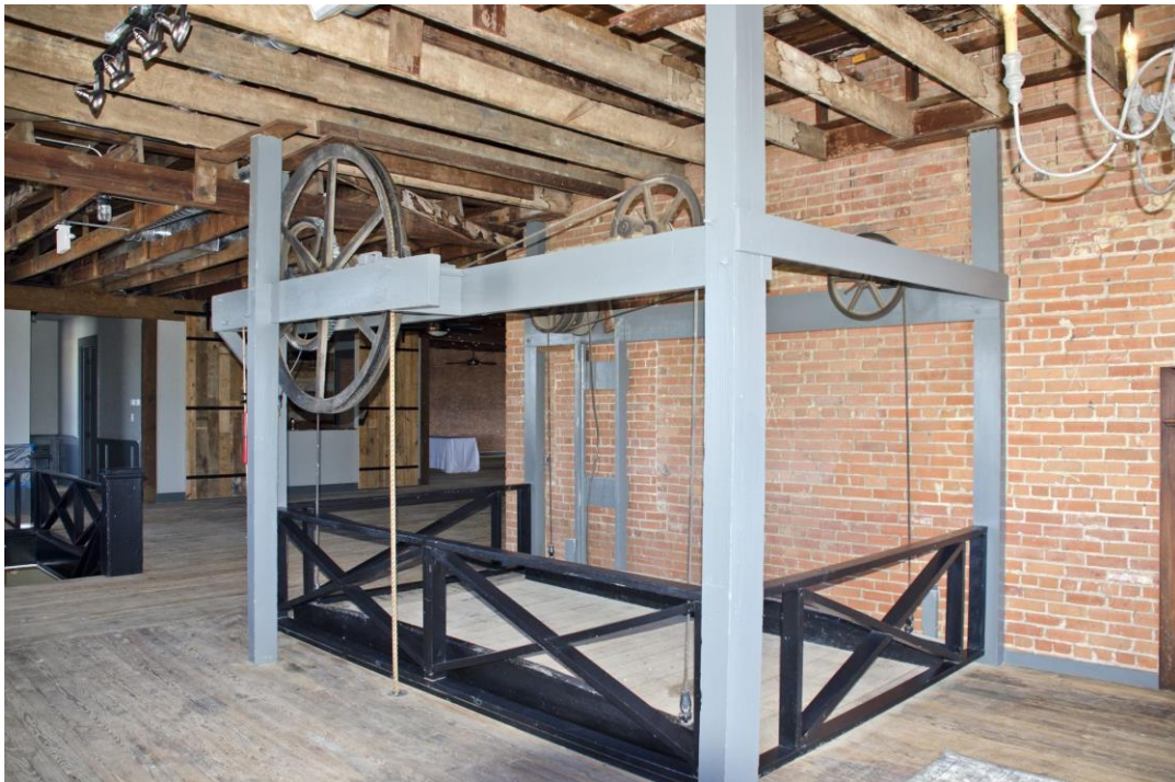
Photo 13 Second Floor Interior, Looking northeast
