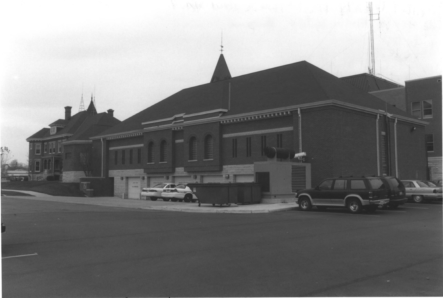
Nicollet County Courthouse and Jail Nicollet County, MN 014241-15A116
