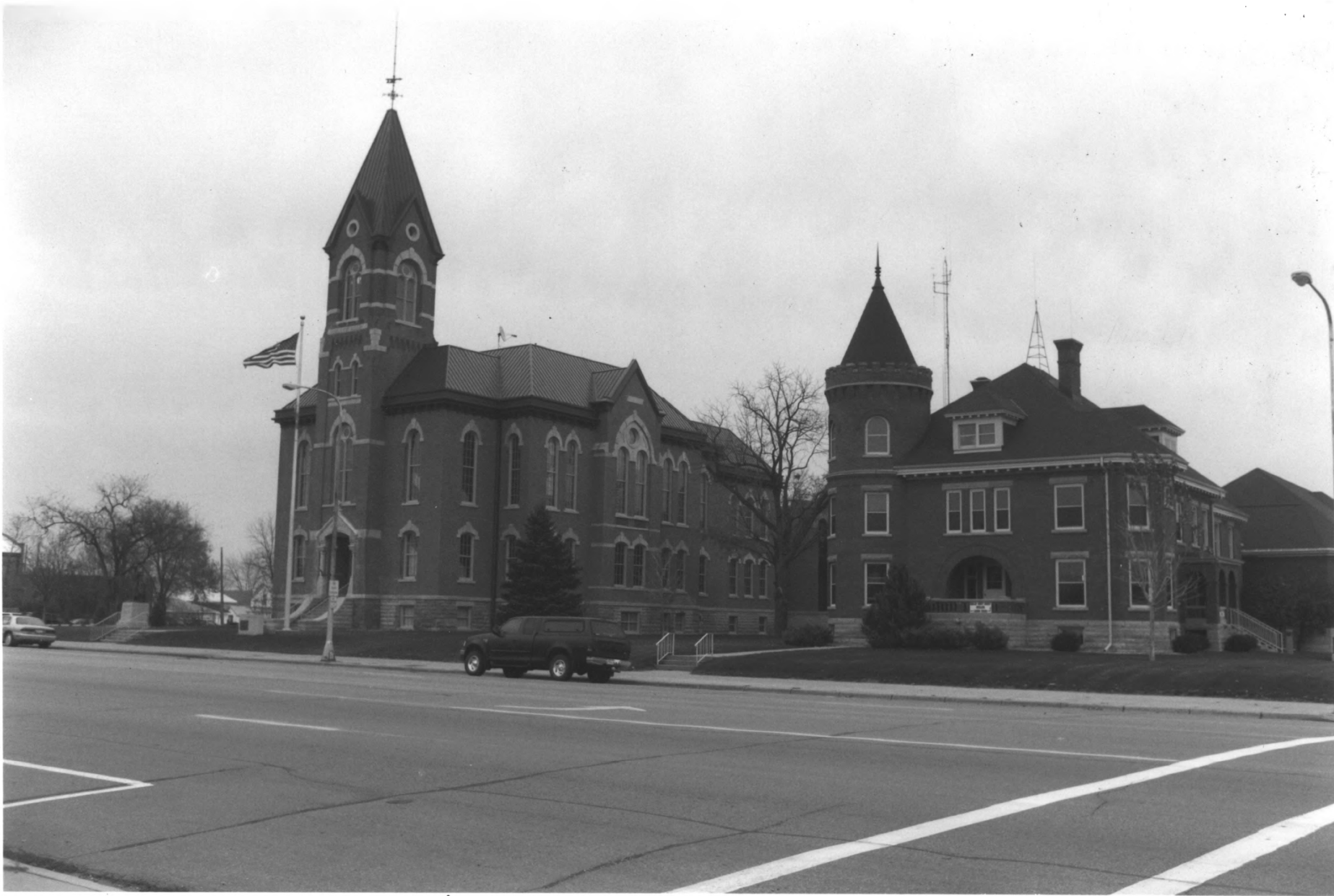
Nicollet County Courthouse and Jail Nicollet County, Mn 014241- 1A/2
