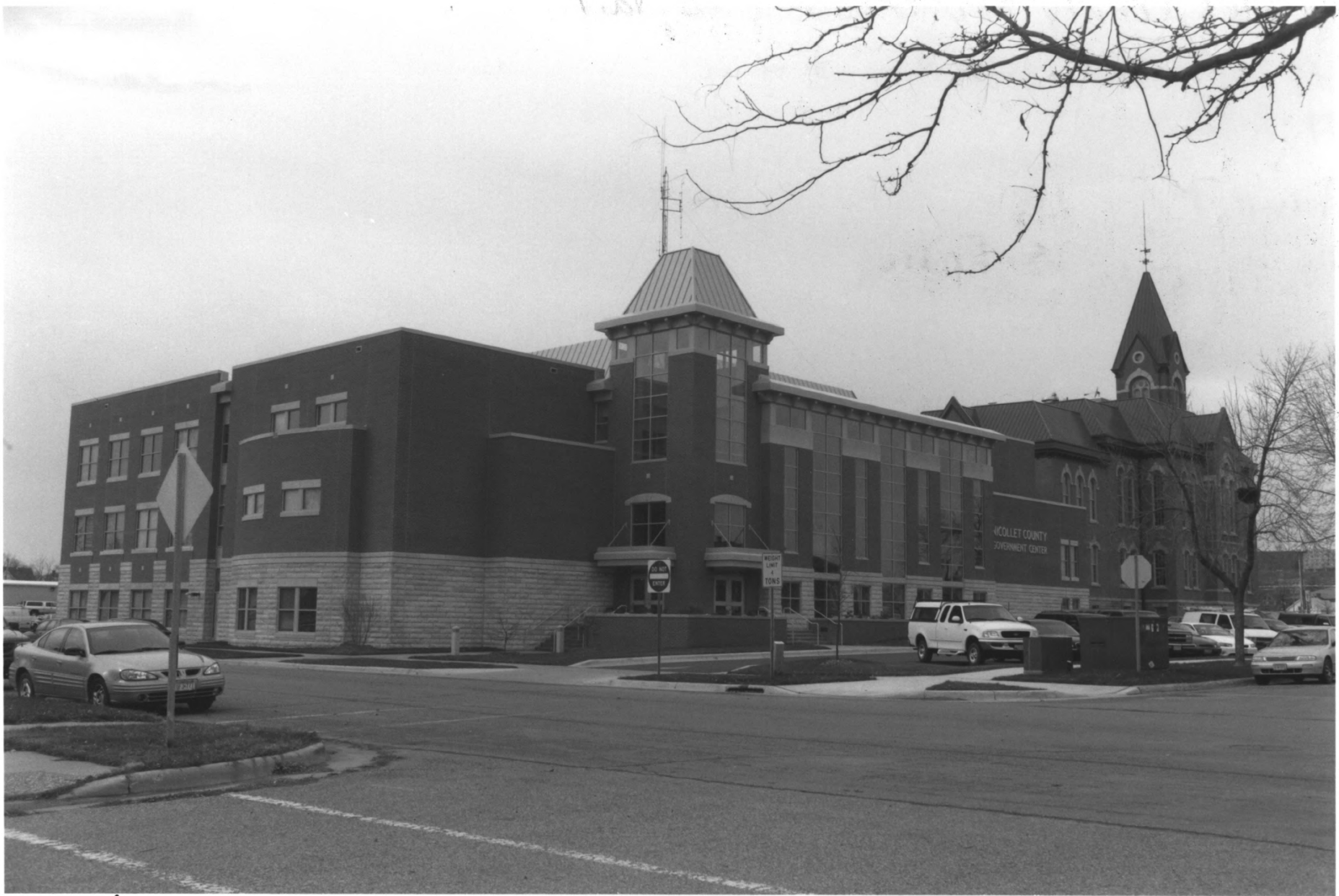
Nicollet County Courthouse and Jail Nicollet County, MN 014241-13A/14
