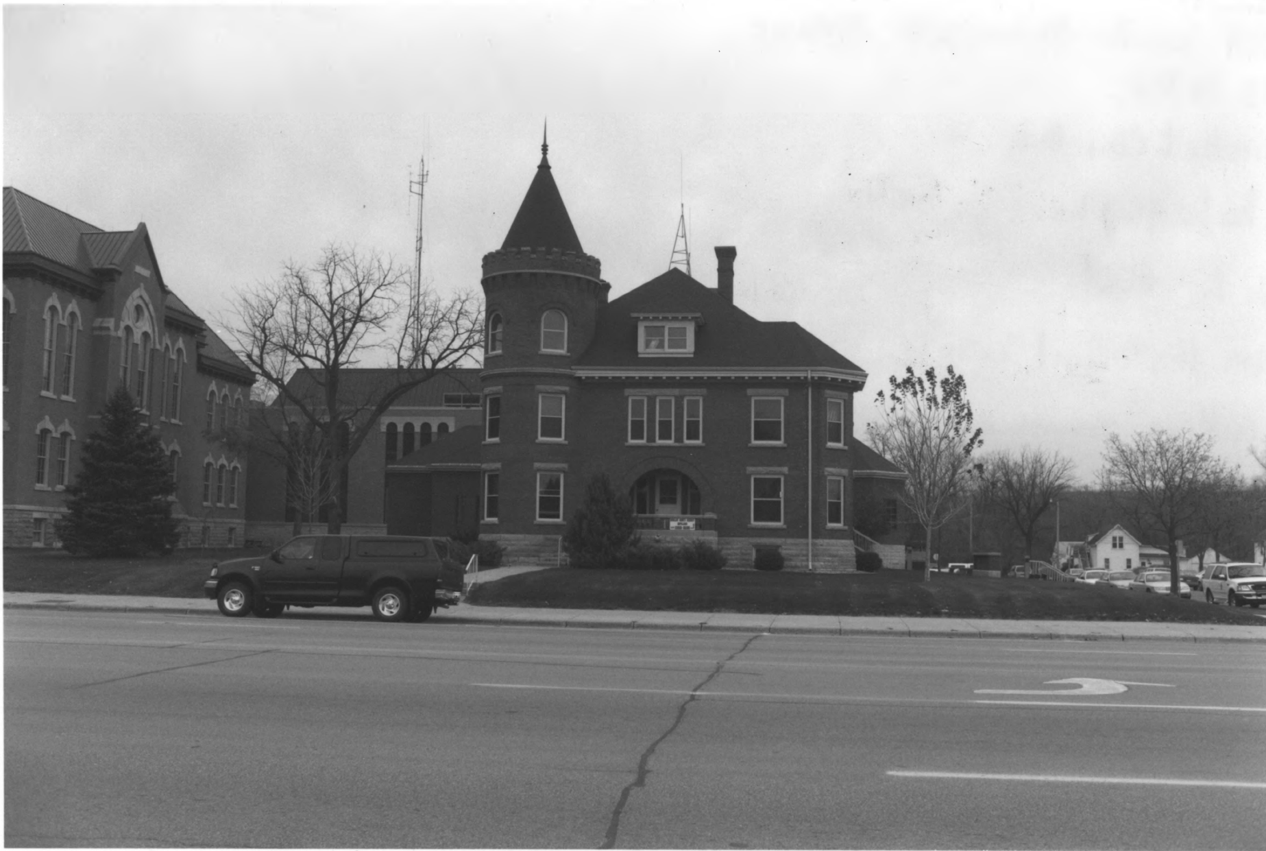
Nicollet County Courthouse and Jail Nicollet County, MN 014241-3A/4
