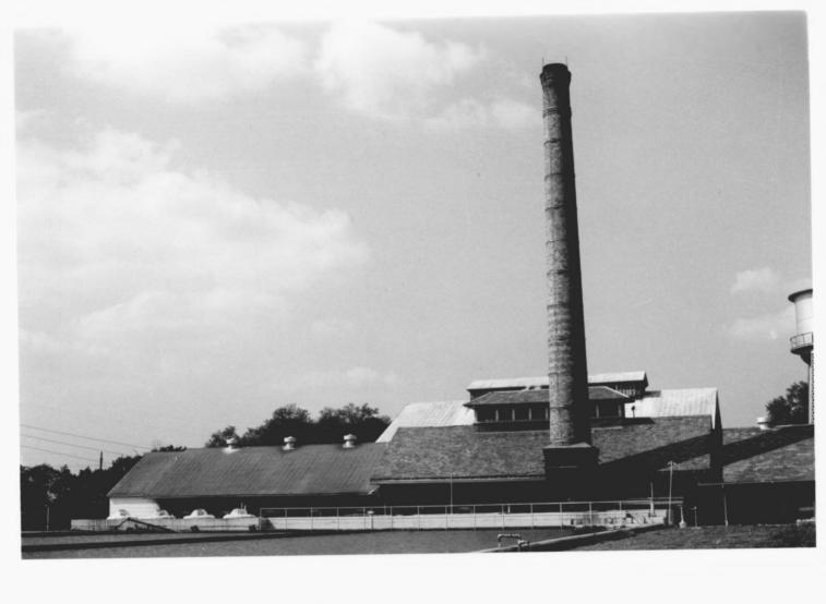
South Elevation over looking settling basins and a view of the 1901 Adophus Custodis stack
