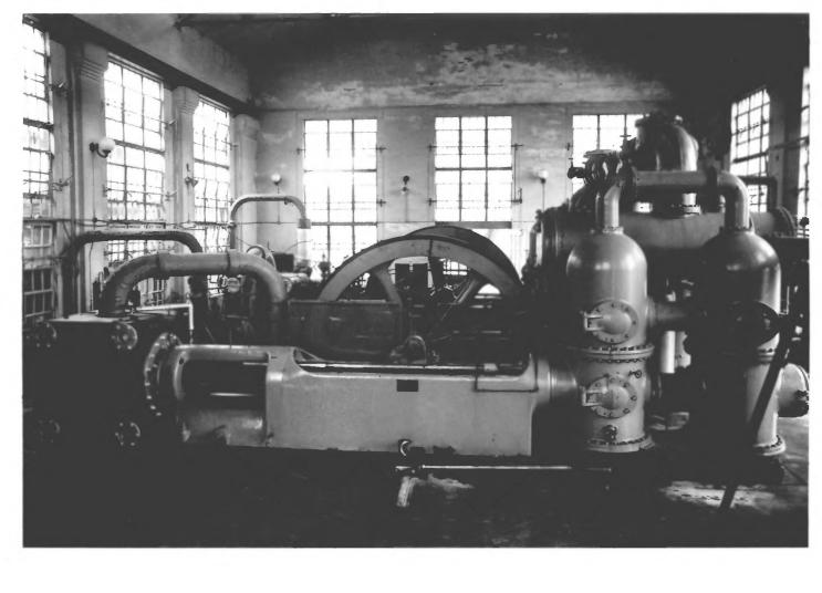
$N\Theta$ -3 &4 High-Service Engines, installed in 1921
