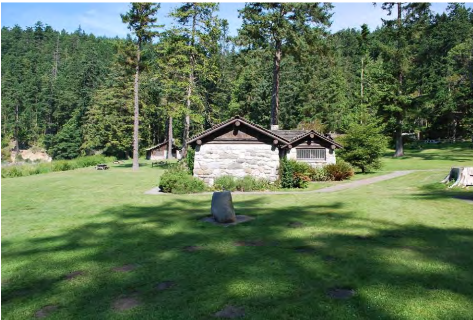
Photo 23 of 28: ID#20, Drinking Fountain. View to north with Bath House (ID#15) and Community Kitchen (ID#16) in background, taken 8/1/2012.
