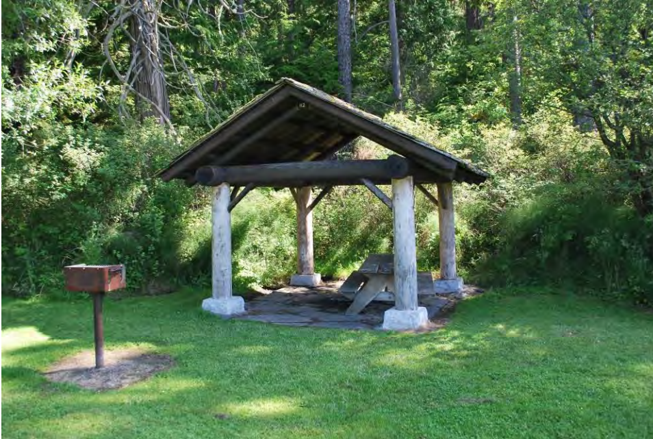
Photo 22 of 28: ID#19, Bowman Bay Campstove Shelter. View to east taken 8/1/2012.
