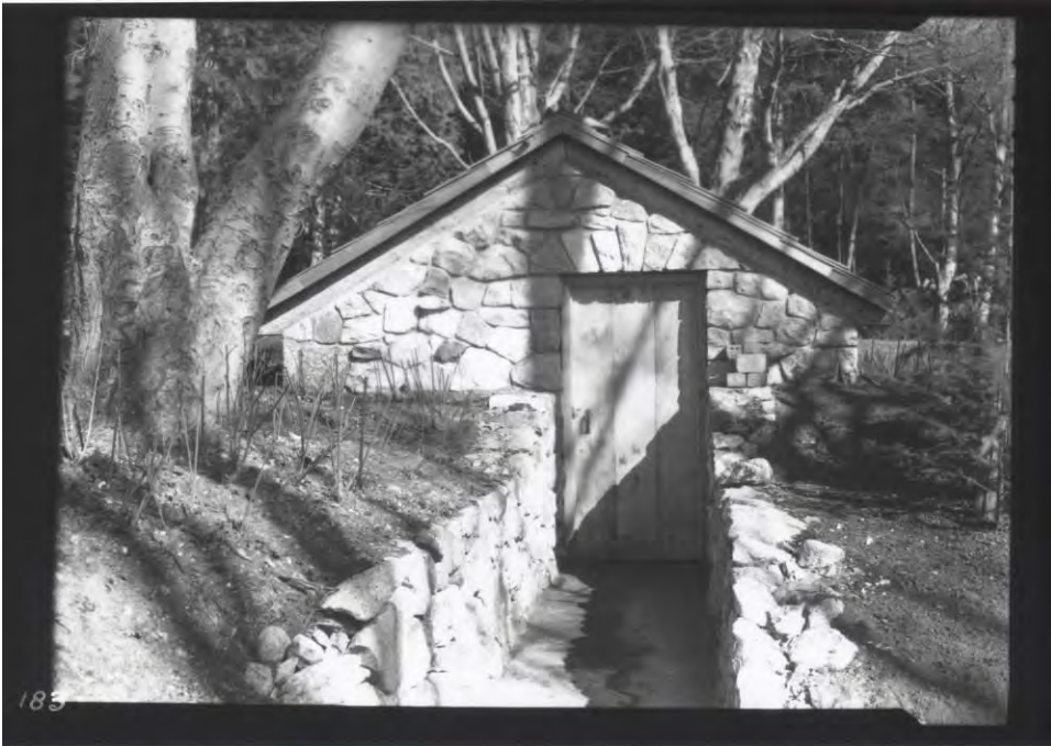
Rosario Pump House (ID#2) completed, view to east.
