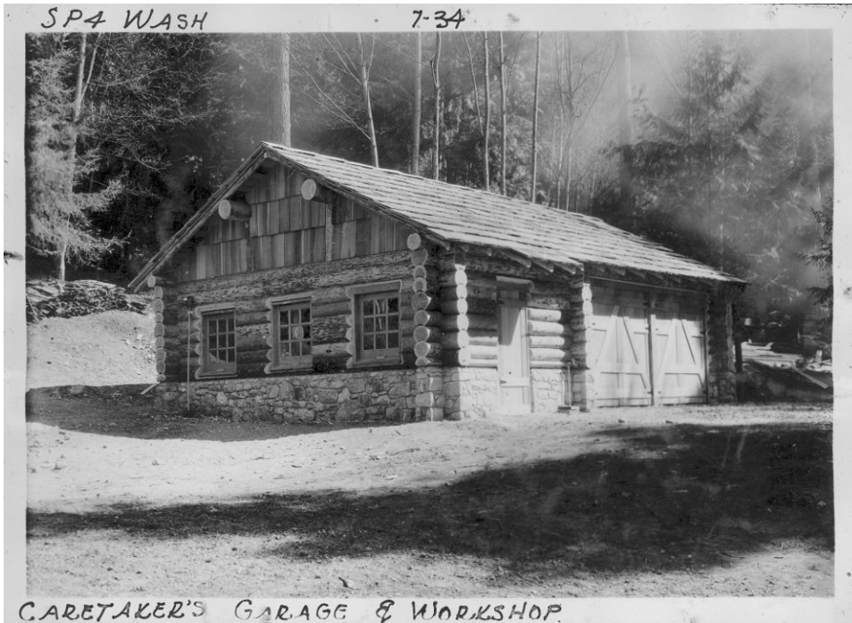
Bowman Bay Caretaker's Shop and Garage (ID#13), view to east.
