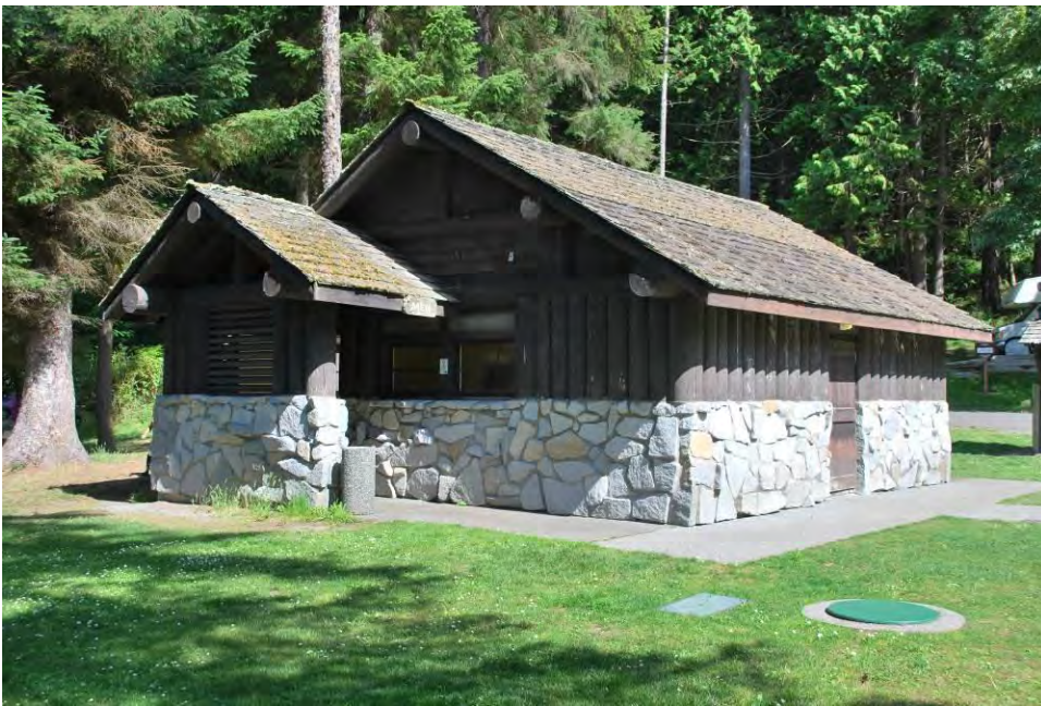
Photo 21 of 28: ID#18, Bowman Bay Comfort Station. View to northeast taken 8/1/2012.
