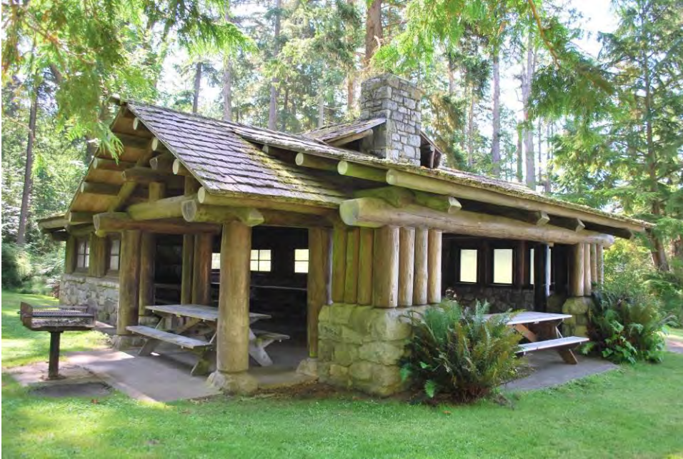
Photo 20 of 28: ID#17, Bowman Bay Combination Building. View to southwest taken 8/1/2012.
