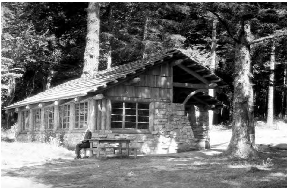
Completed Bowman Bay Community Kitchen (ID#16), view to northwest.
