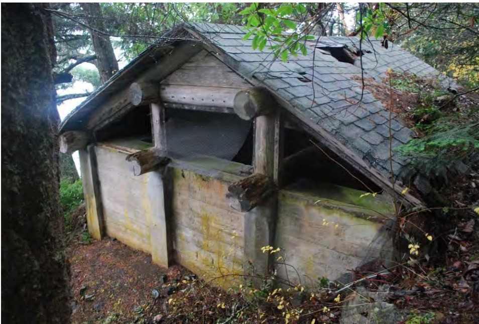
Photo 11 of 28: ID#10, Water Storage Reservoir. View to southwest taken 11/18/2014.
