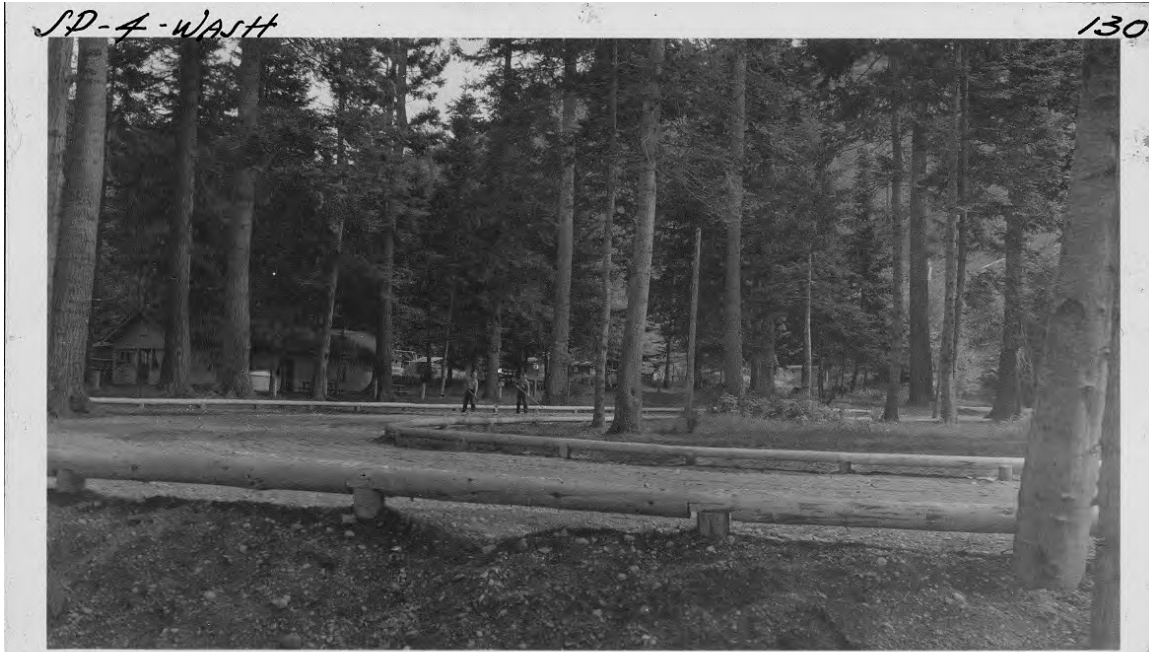
62 FINISHING PARKING AREA AT ROSARIO BEACH. Completed Parking Area (ID#6), view to east.
