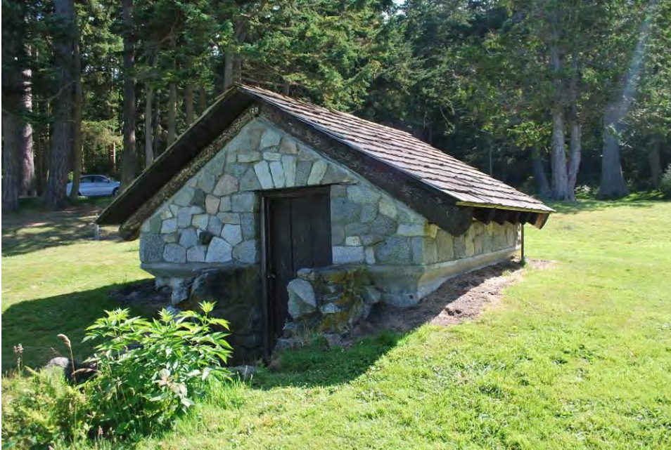
Photo 2 of 28: ID#2, Rosario Pump House. View to east taken 8/1/2012.
