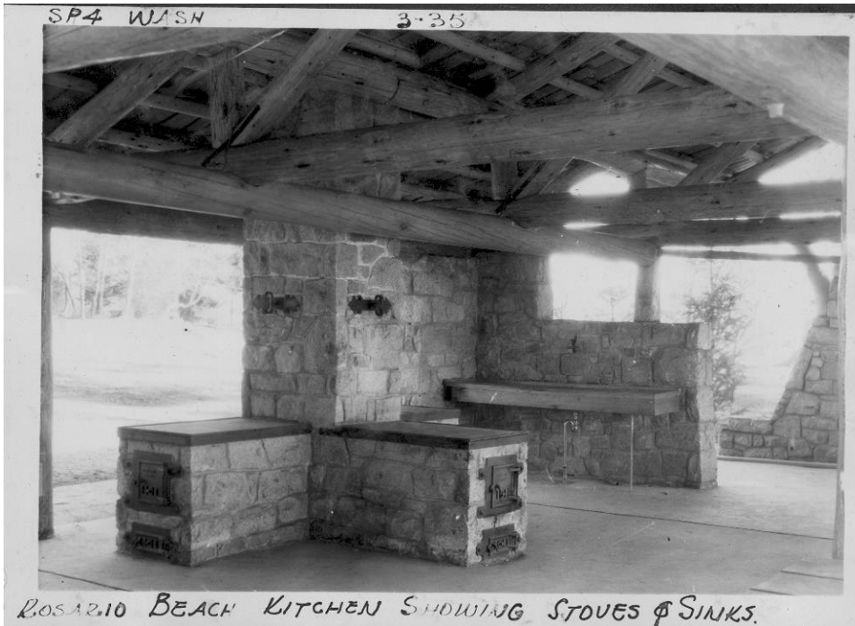
Interior view of completed Community Kitchen.
