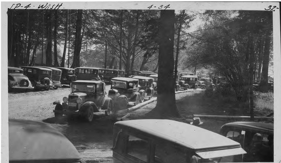
63 PARKING AREA FILLED BY VISITORS ON SUNDAY Completed Parking Area (ID#6), view to southwest.
