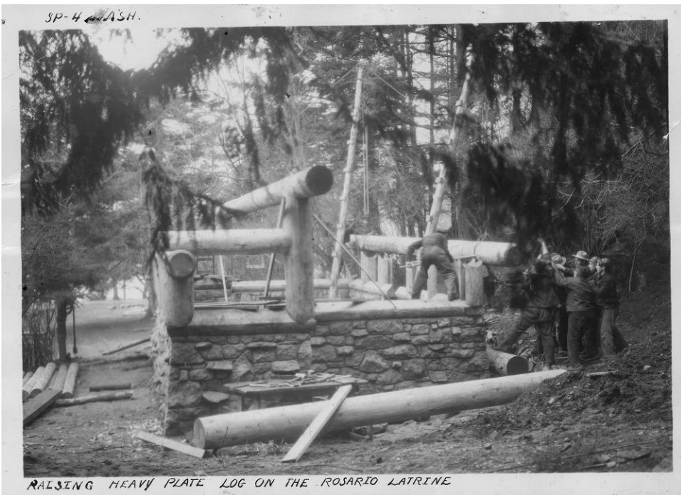
Rosario Latrine (ID#3) under construction, view to west.
