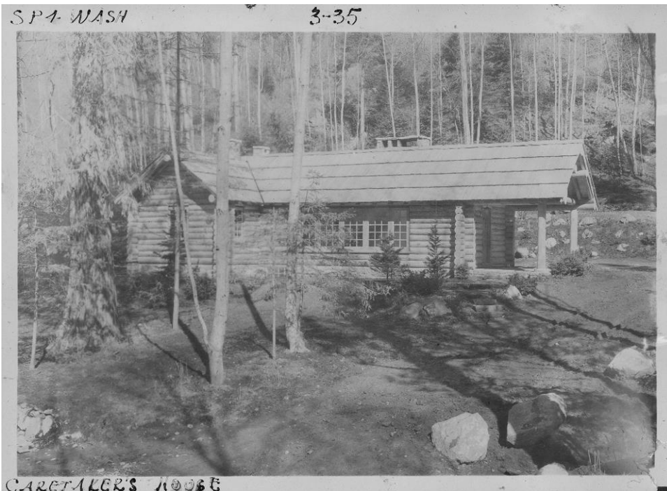
Completed Caretaker's Residence (ID#12), view to north.
