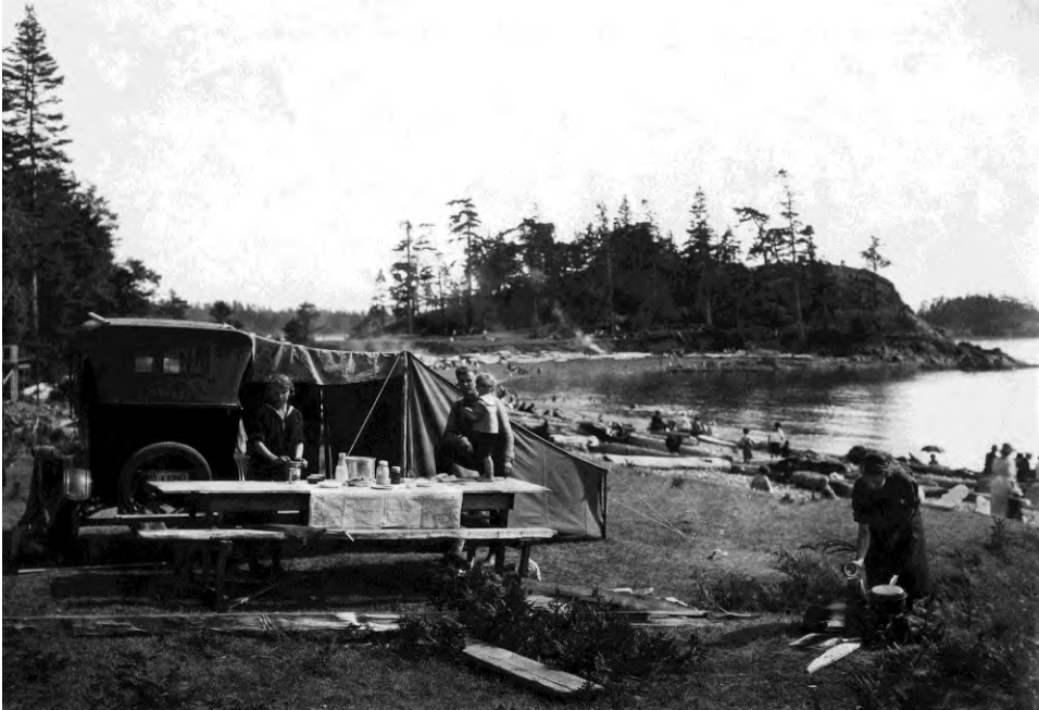
Pre-Depression view of park users at Rosario, view to south.
