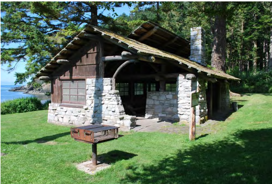
Photo 19 of 28: ID#16, Bowman Bay Community Kitchen. View to northwest taken 8/1/2012.
