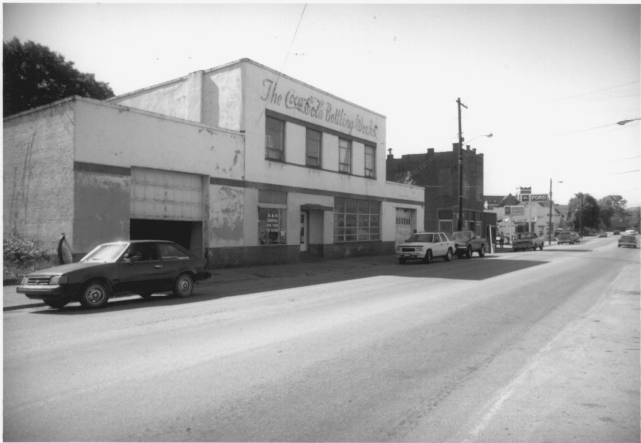
Jellico Commercial Historic District, Campbell County, TN
