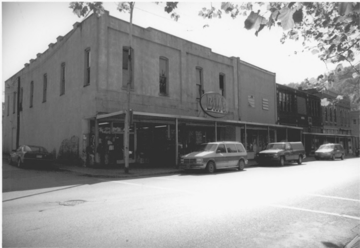
Jellico Commercial Historic District, Campbell County, TN
