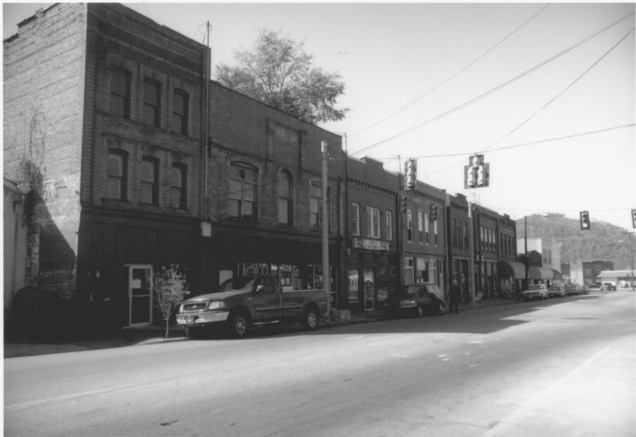
Jellico Commercial Historic District, Campbell County, TN
