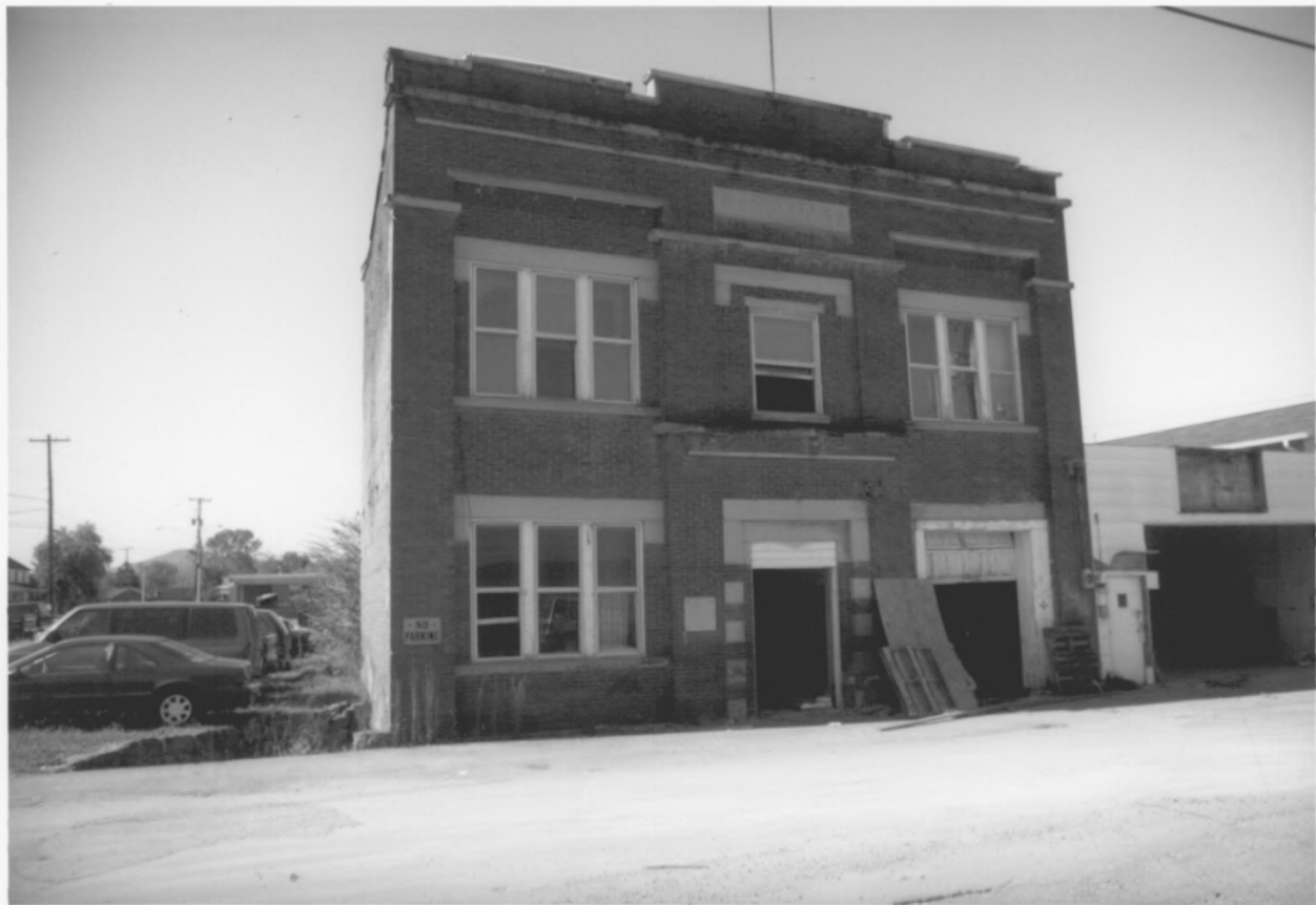
Jellico Commercial Historic District, Campbell County, TN
