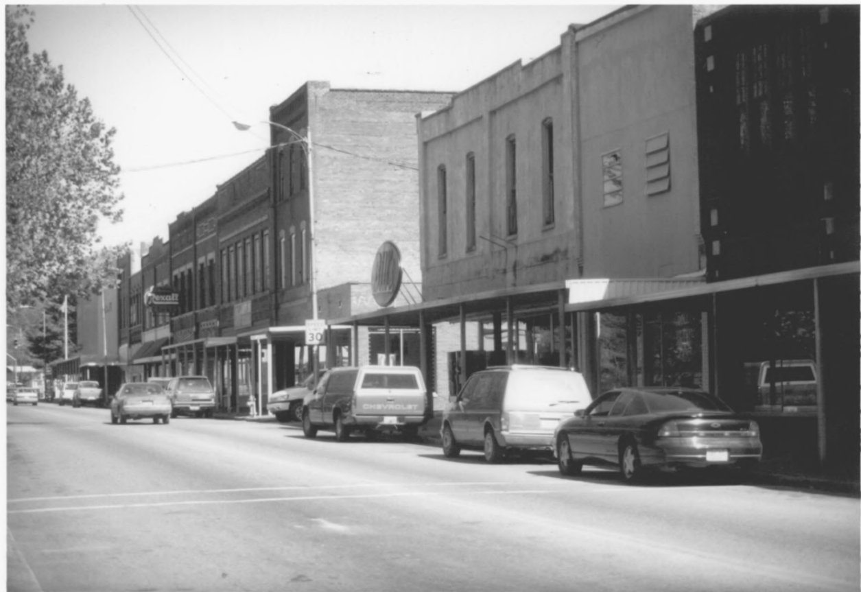
Jellico Commercial Historic District, Campbell County, TN
