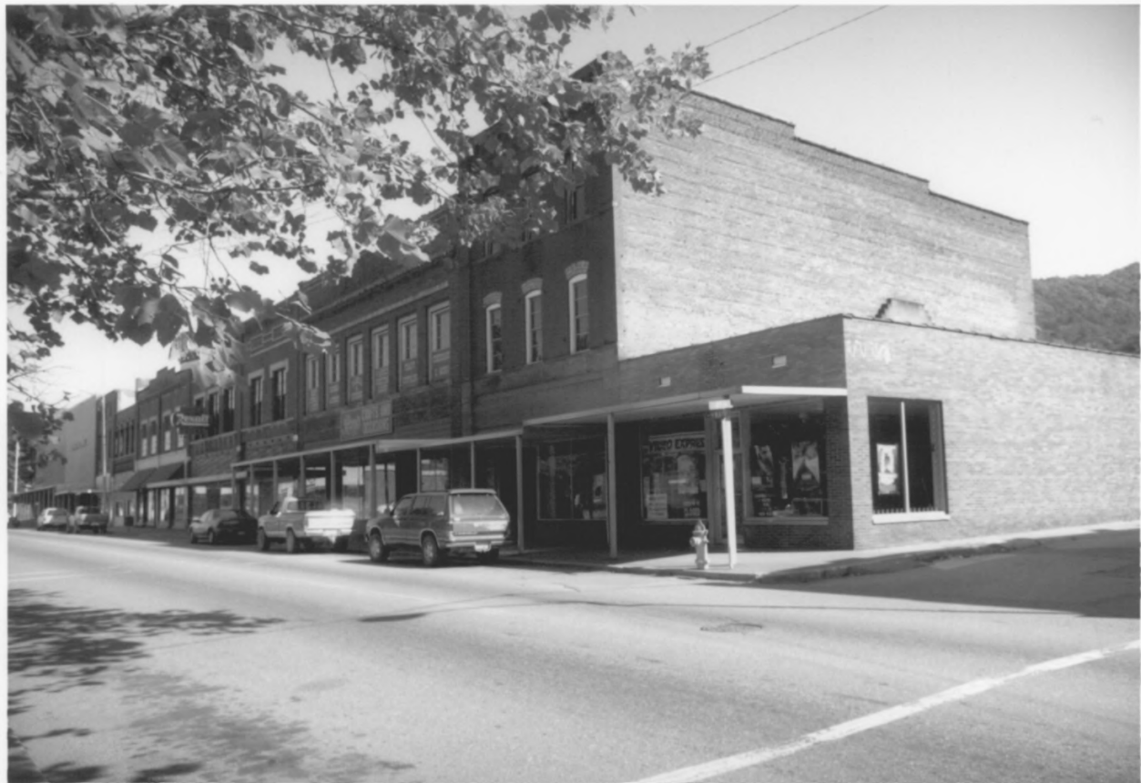
Jellico Commercial Historic District, Campbell County, TN
