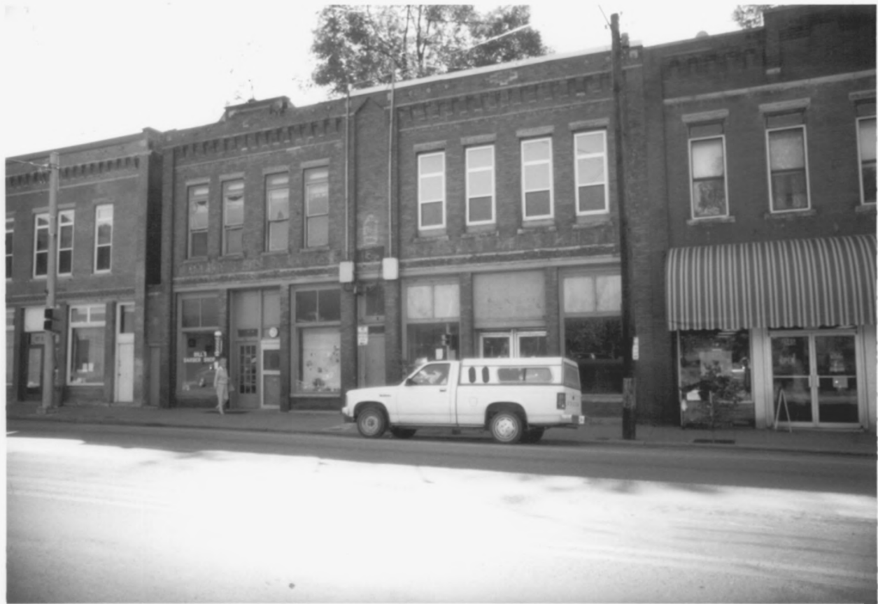
Jellico Commercial Historic District, Campbell County, TN
