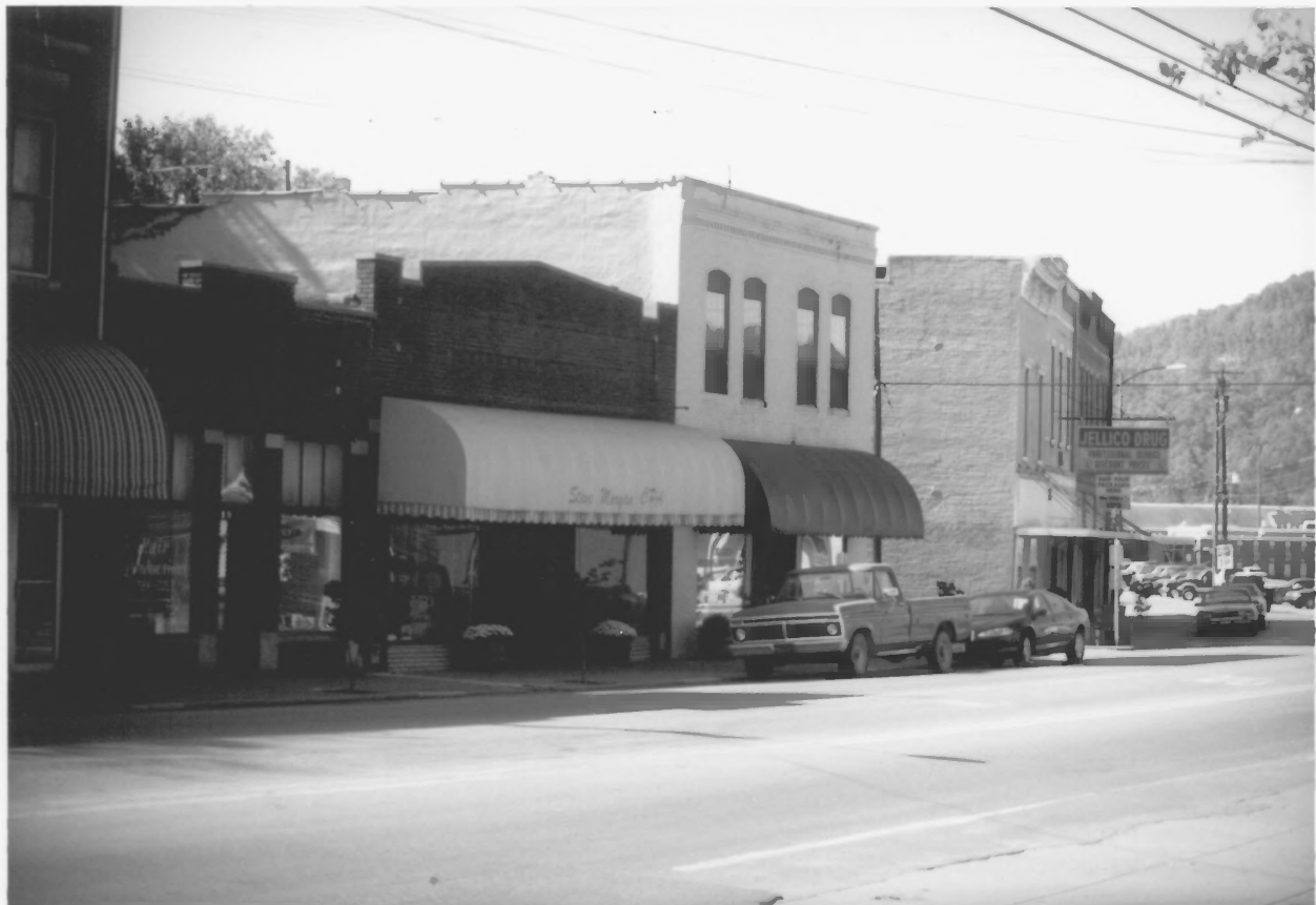
Jellico Commercial Historic District, Campbell County, TN
