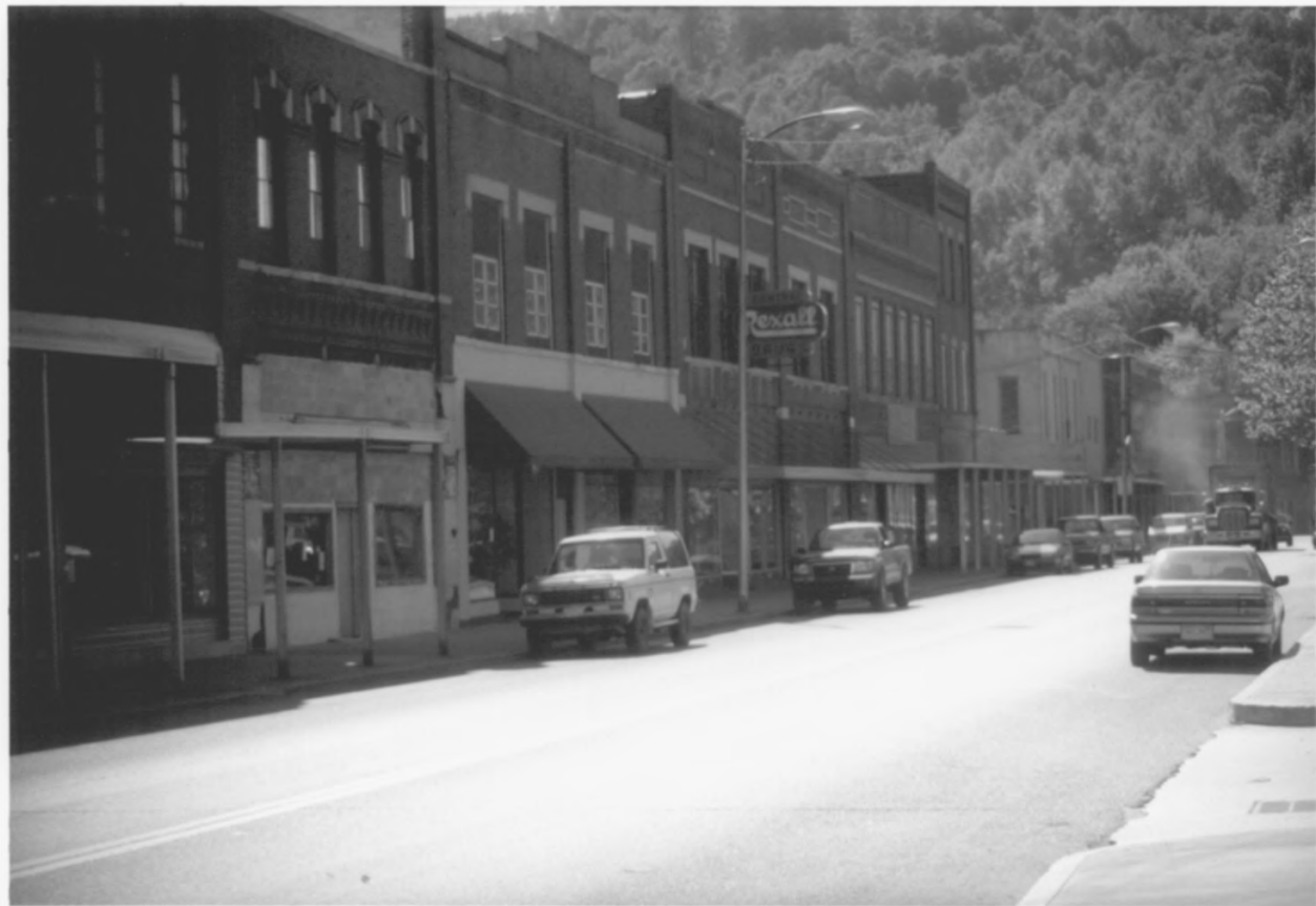
Jellico Commercial Historic District, Campbell County, TN
