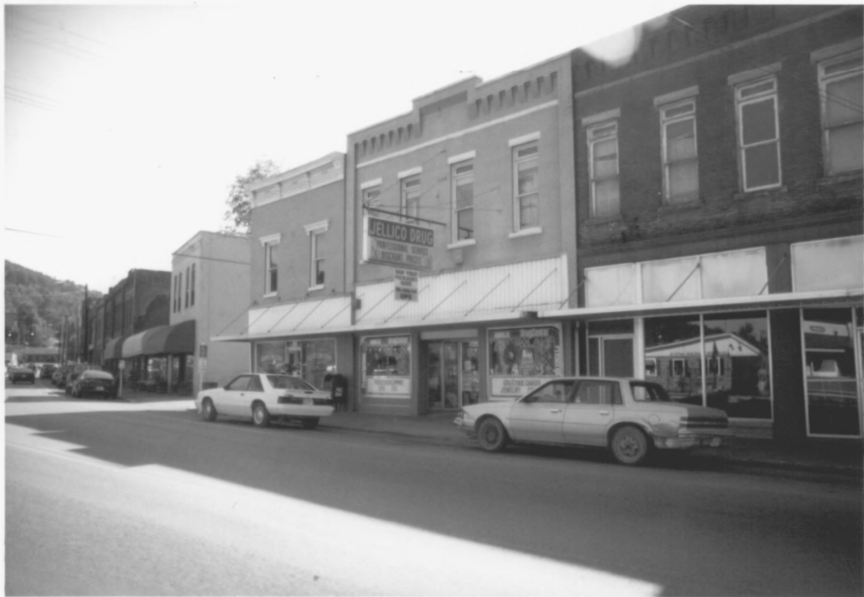
Jellico Commercial Historic District, Campbell County, TN
