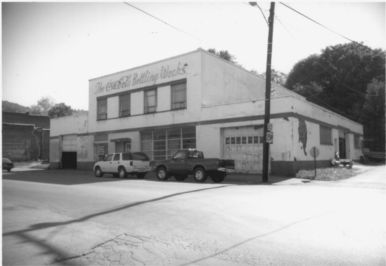
Jellico Commercial Historic District, Campbell County, TN
