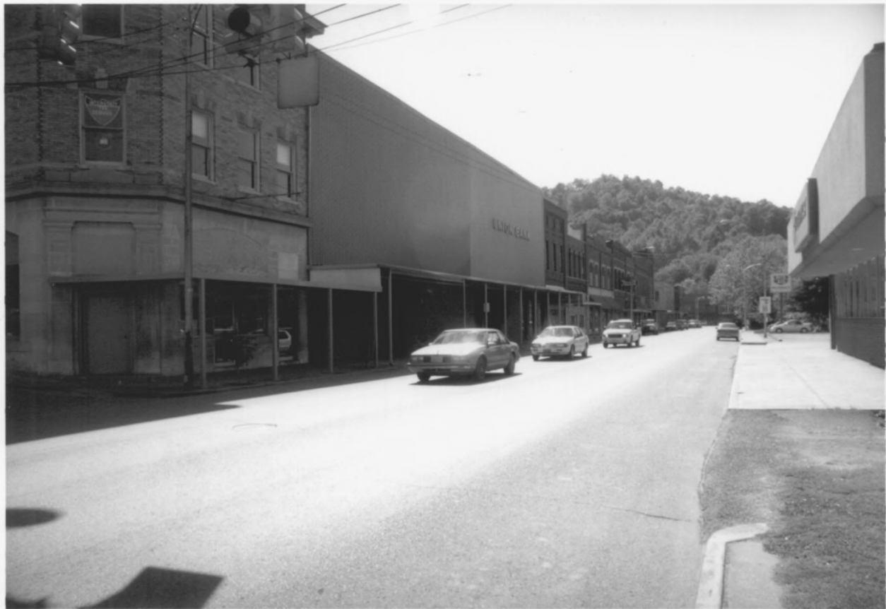
Jellico Commercial Historic District, Campbell County, TN
