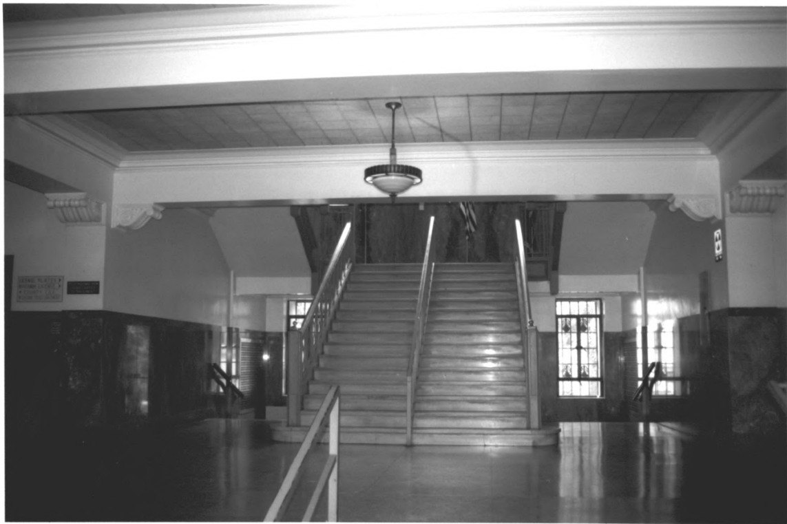
MADISON COUNTY COURTHOUSE MADISON COUNTY TN
