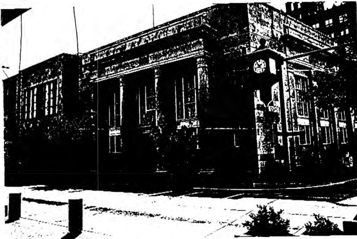
Photograph No. 1: Main Building looking southeast on DeSiard/Jackson Streets, Annex 1 plus partial Annex 2 indicated
