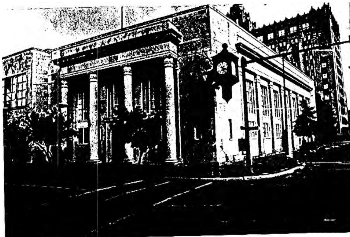
Photograph No. 19: Main Building, facing south, corner DeSiard/Jackson Streets
