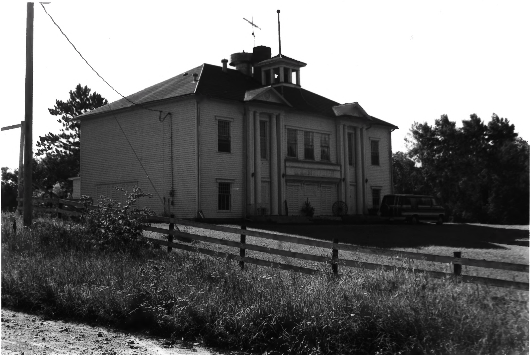
District School No. 132 Beltrami, Co., MN. #08487-16A
