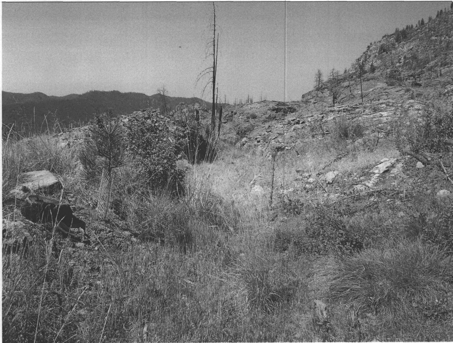
Photo 0011. Section 2. Mullan Road rock cut built in 1860. View to the west.
