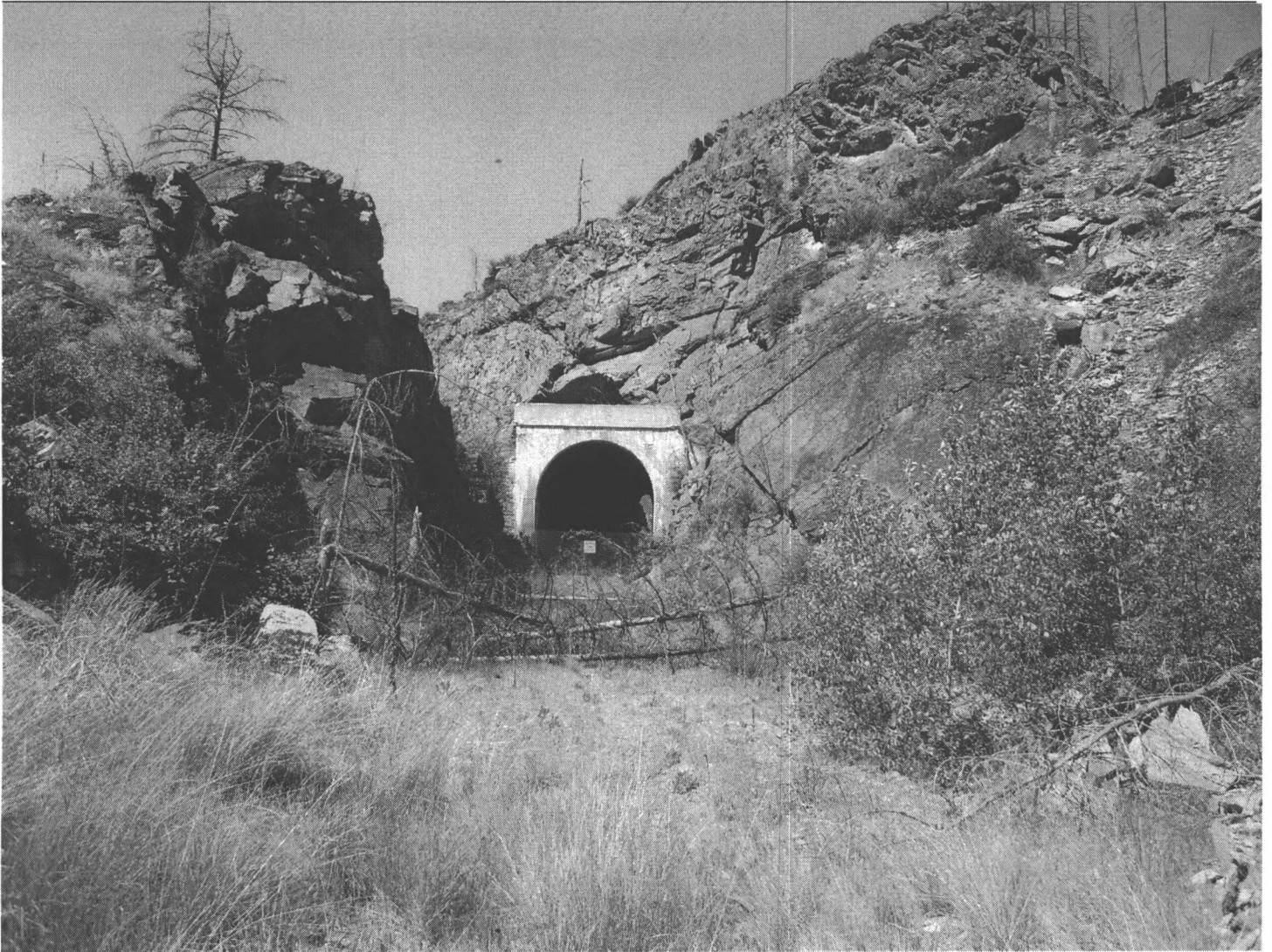
Photo 0040. Section 5. Tunnel 18. East portal. View to southwest.
