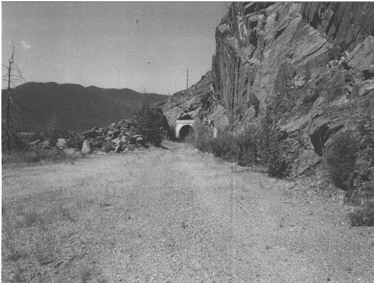
Photo 0029. Section 5. Milwaukee Road Railroad grade. View to southwest toward east portal of Tunnel 18.
