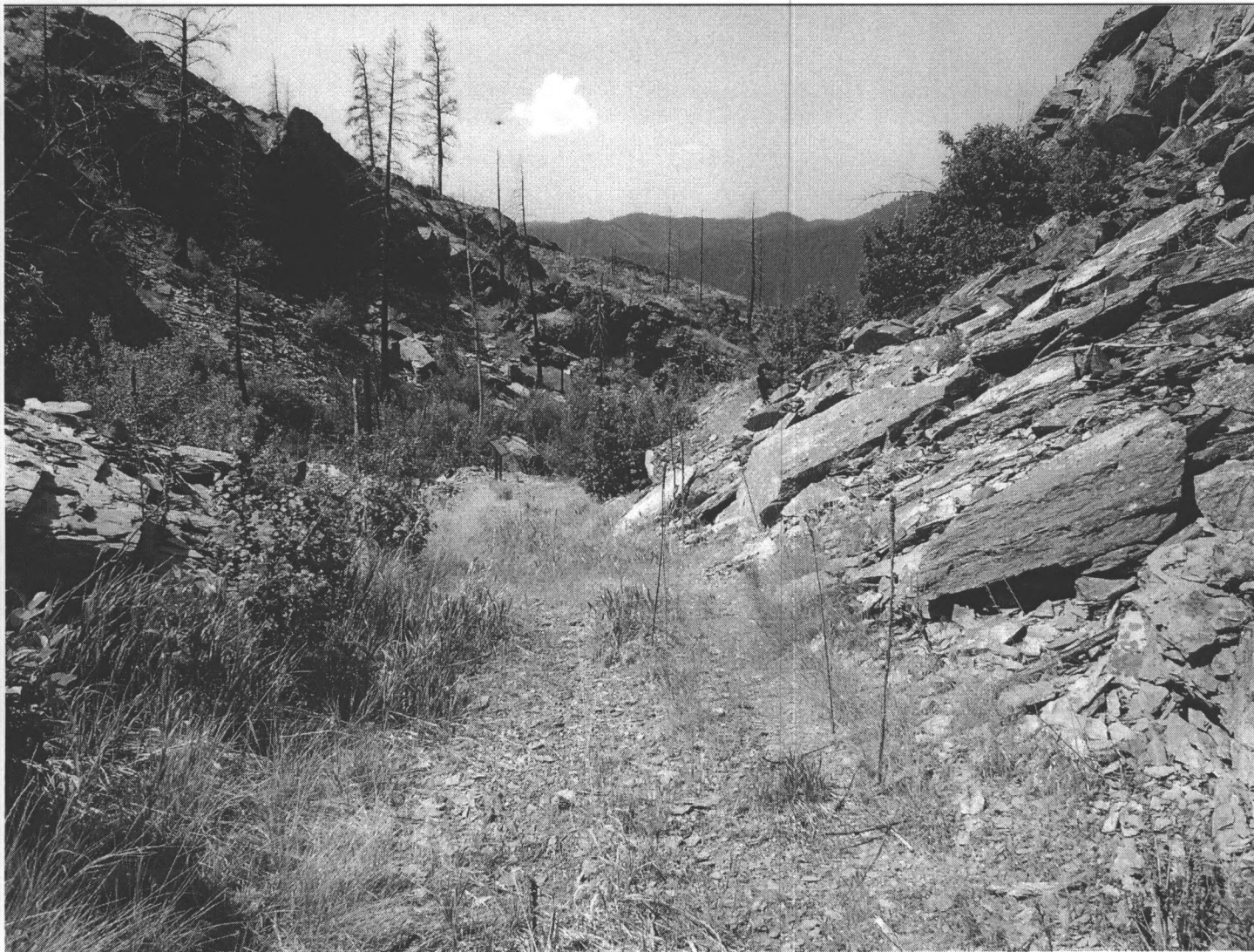
Photo 0024. Section 4. Mullan Road segment; Point of Rocks geologic feature on left. View to the southwest.
