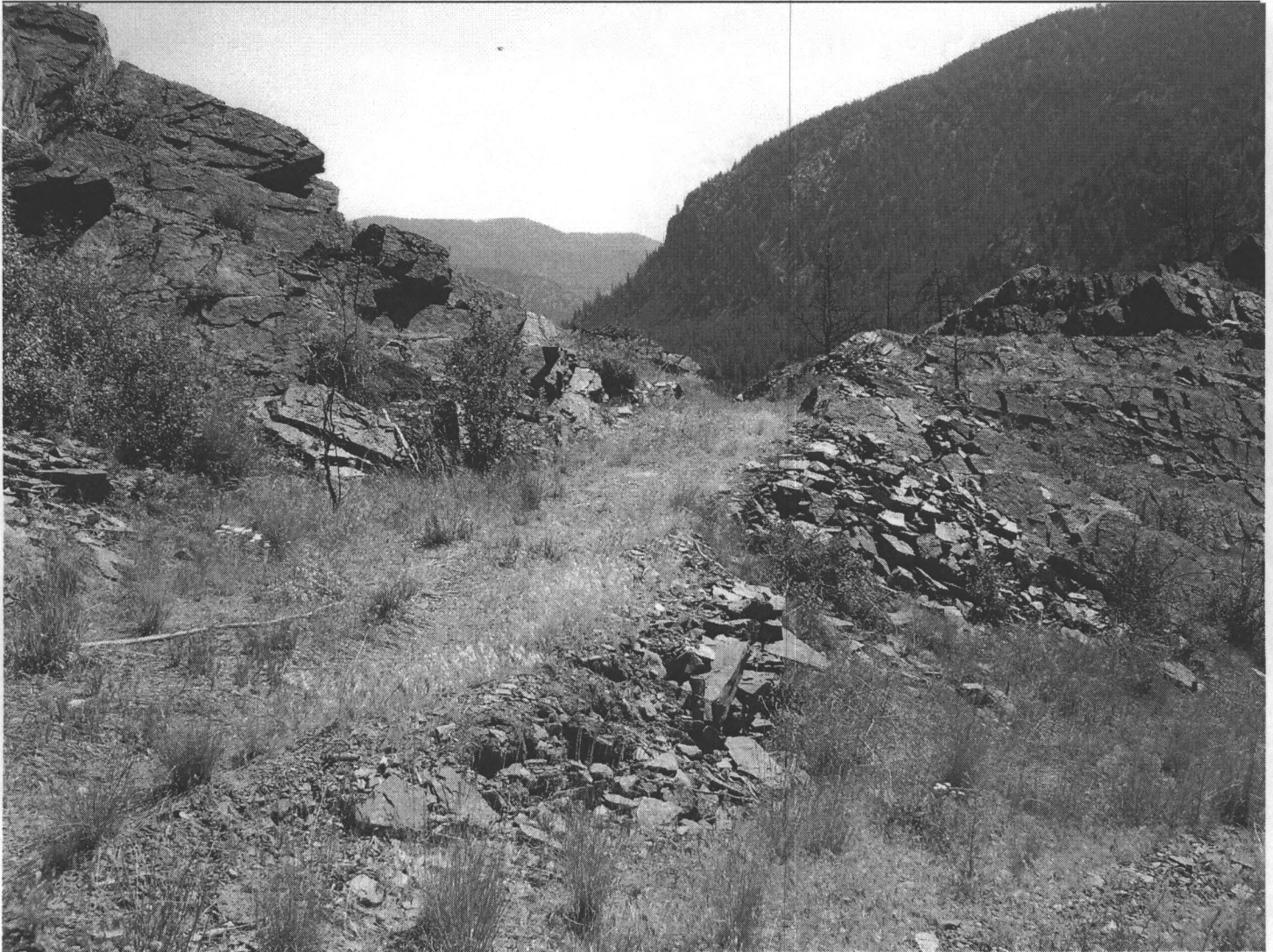
Photo 0023. Section 4. Mullan Road retaining walls. View to southeast.
