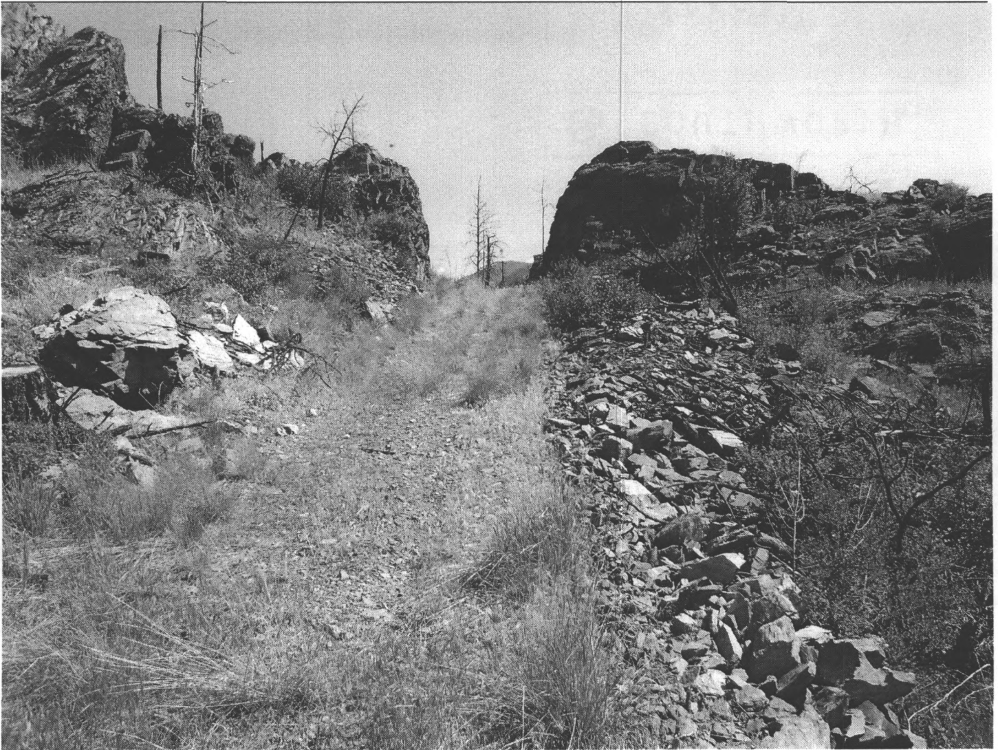
Photo 0034. Section 3. Milwaukee Road Railroad retaining wall (foreground). View to northeast.
