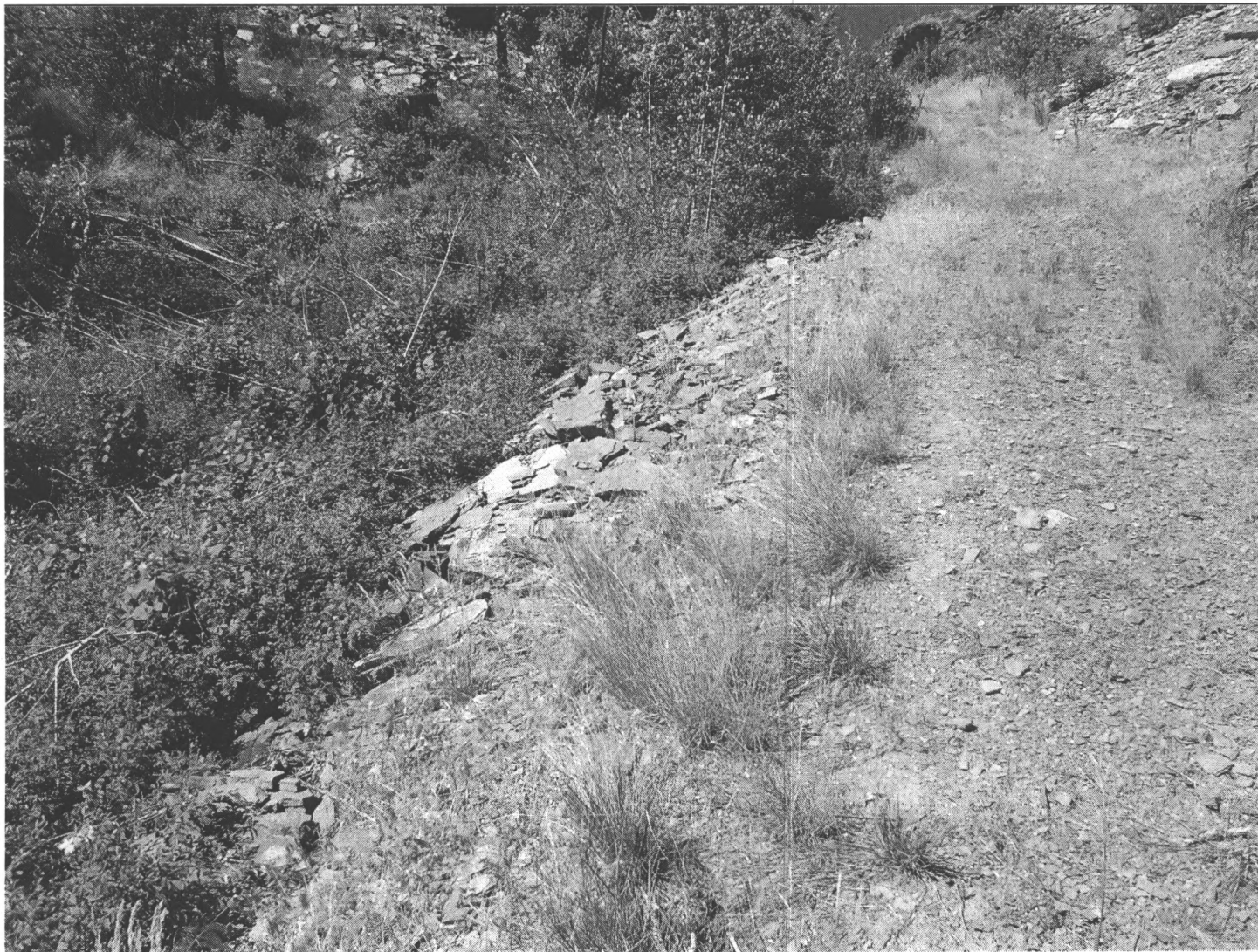
Photo 0037. Section 4. Mullan Road retaining wall. View to southwest.
