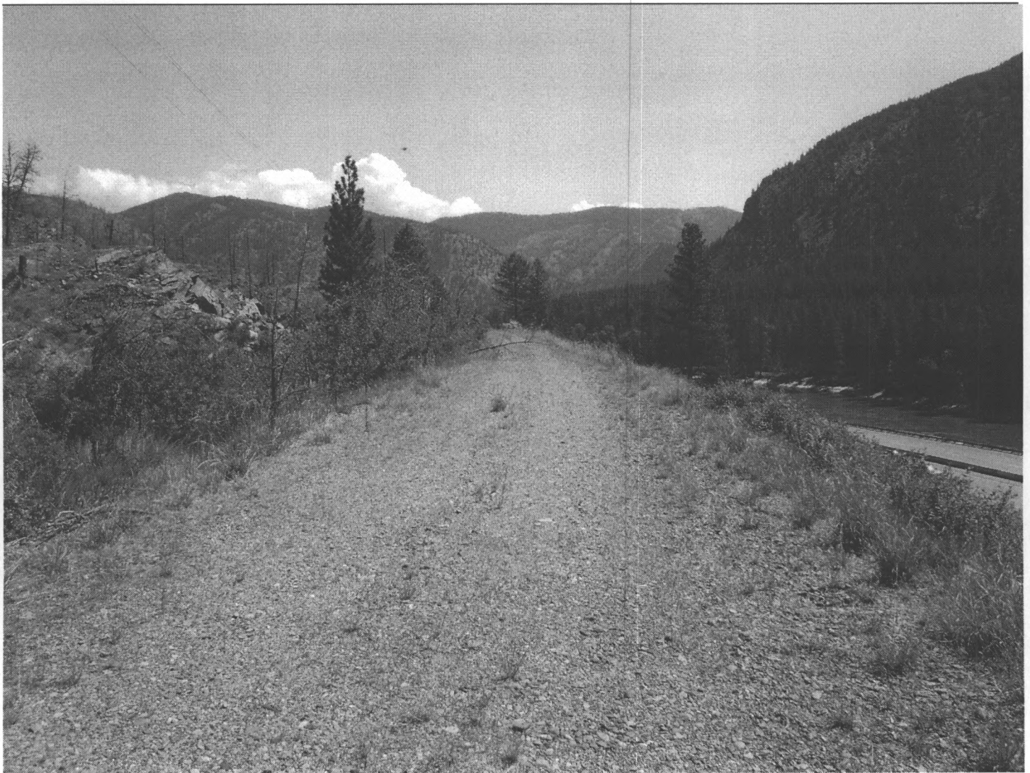
Photo 0030. Section 5. Milwaukee Road Railroad grade. View to northeast.
