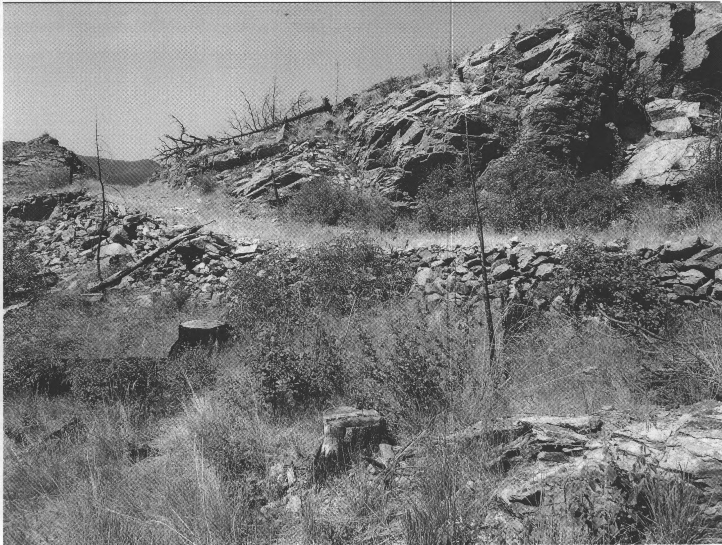
Photo 0035. Section 3. Milwaukee Road Railroad retaining wall. View to northwest.
