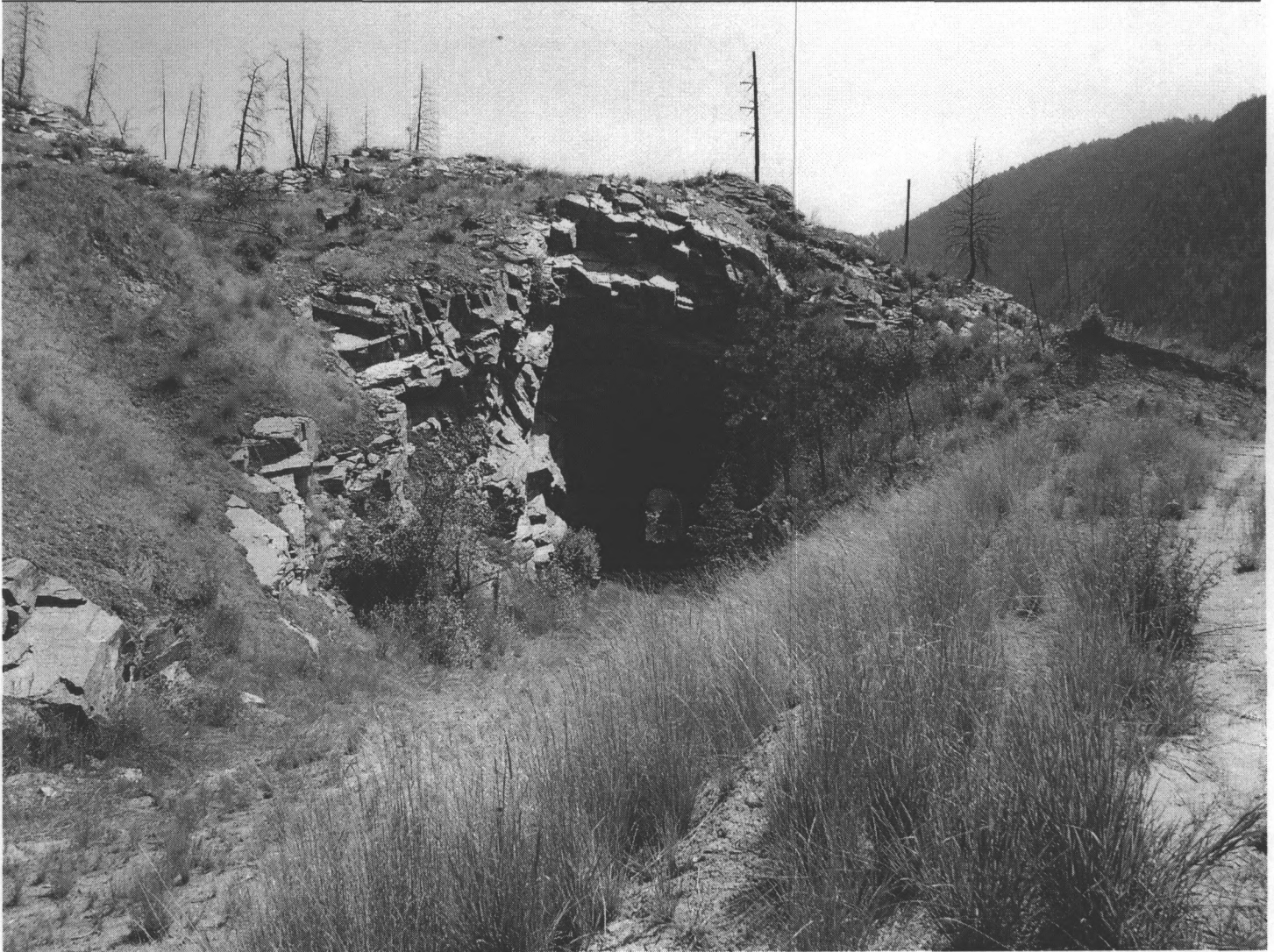
Photo 0039. Section 5. Tunnel 18. West portal. View to northeast.
