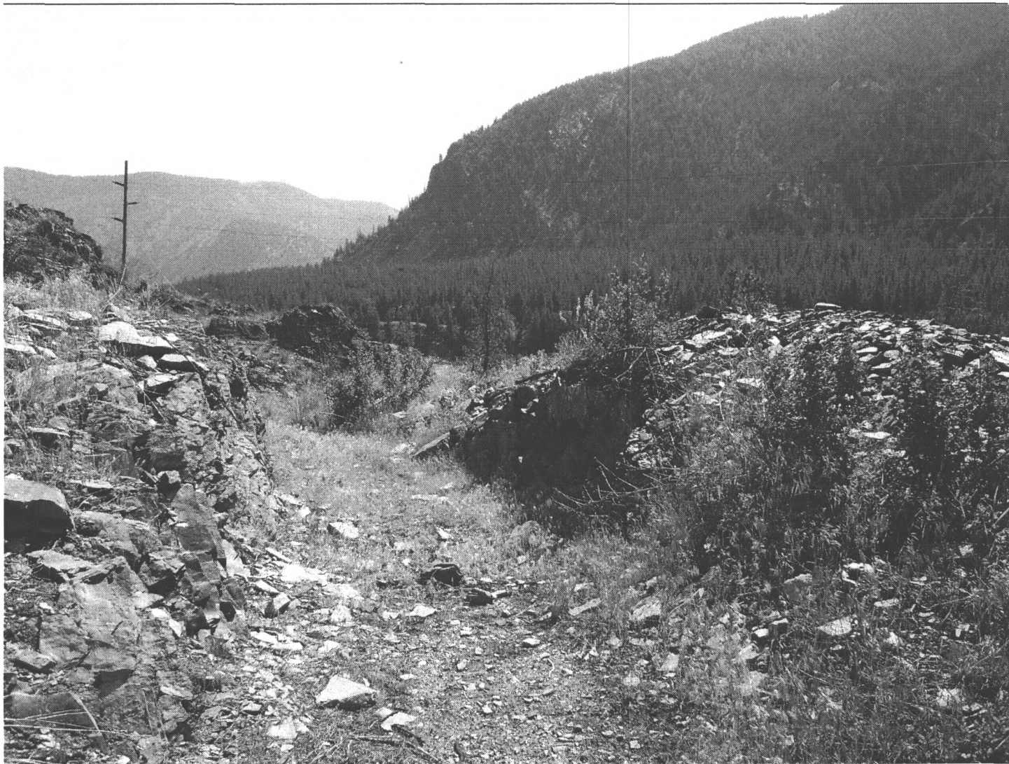
Photo 0010. Section 2. Mullan Road rock cut built in 1860. View to the east.
