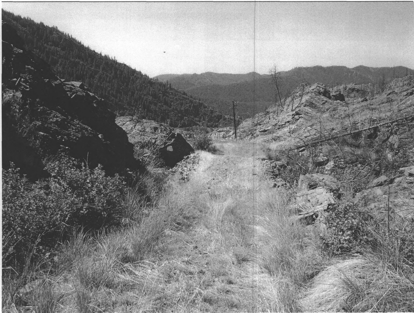
Photo 0020. Section 4. Mullan Road segment View to the southwest.
