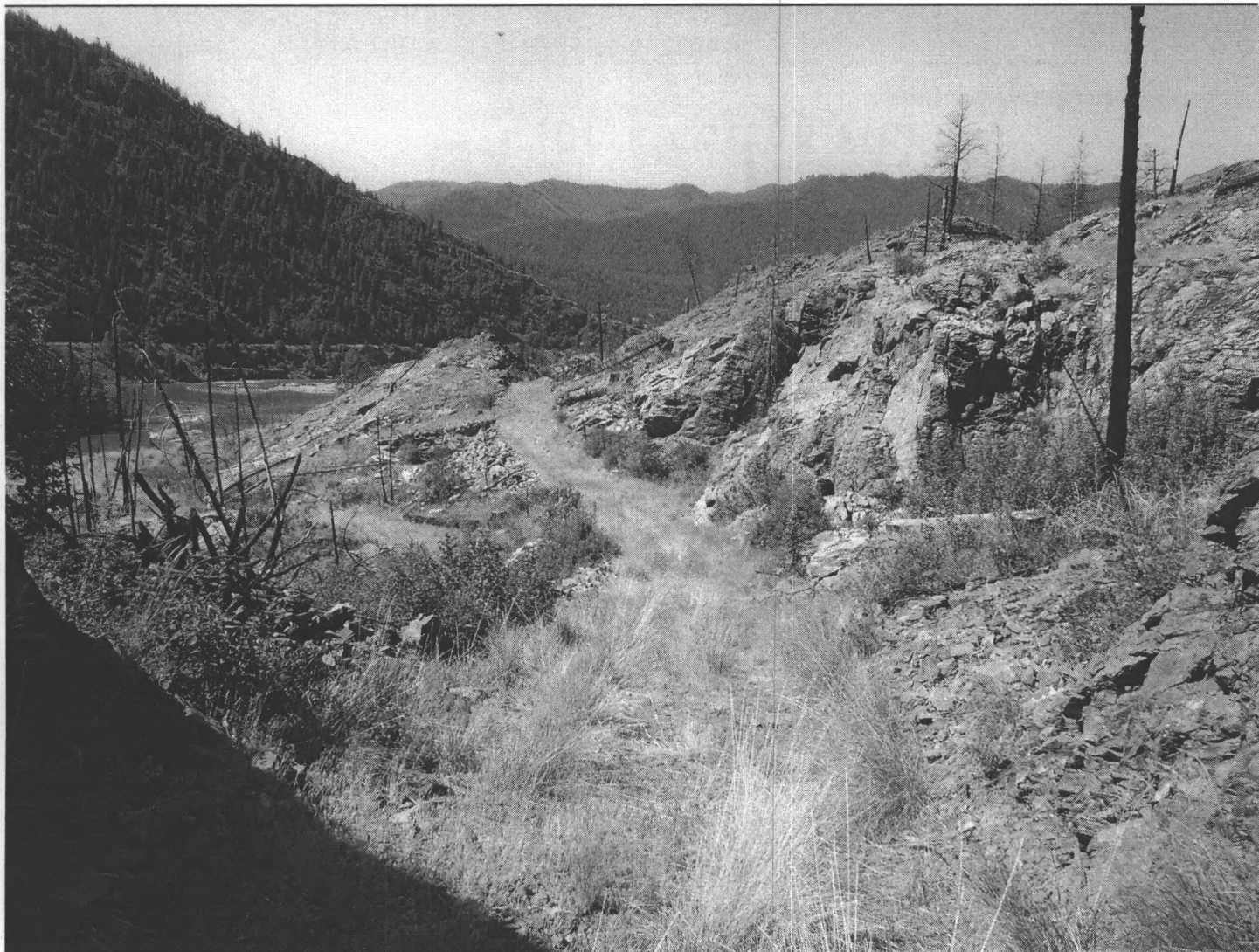
Photo 0017. Section 3. Milwaukee Road RR-built segment looking southwest toward Point C.
