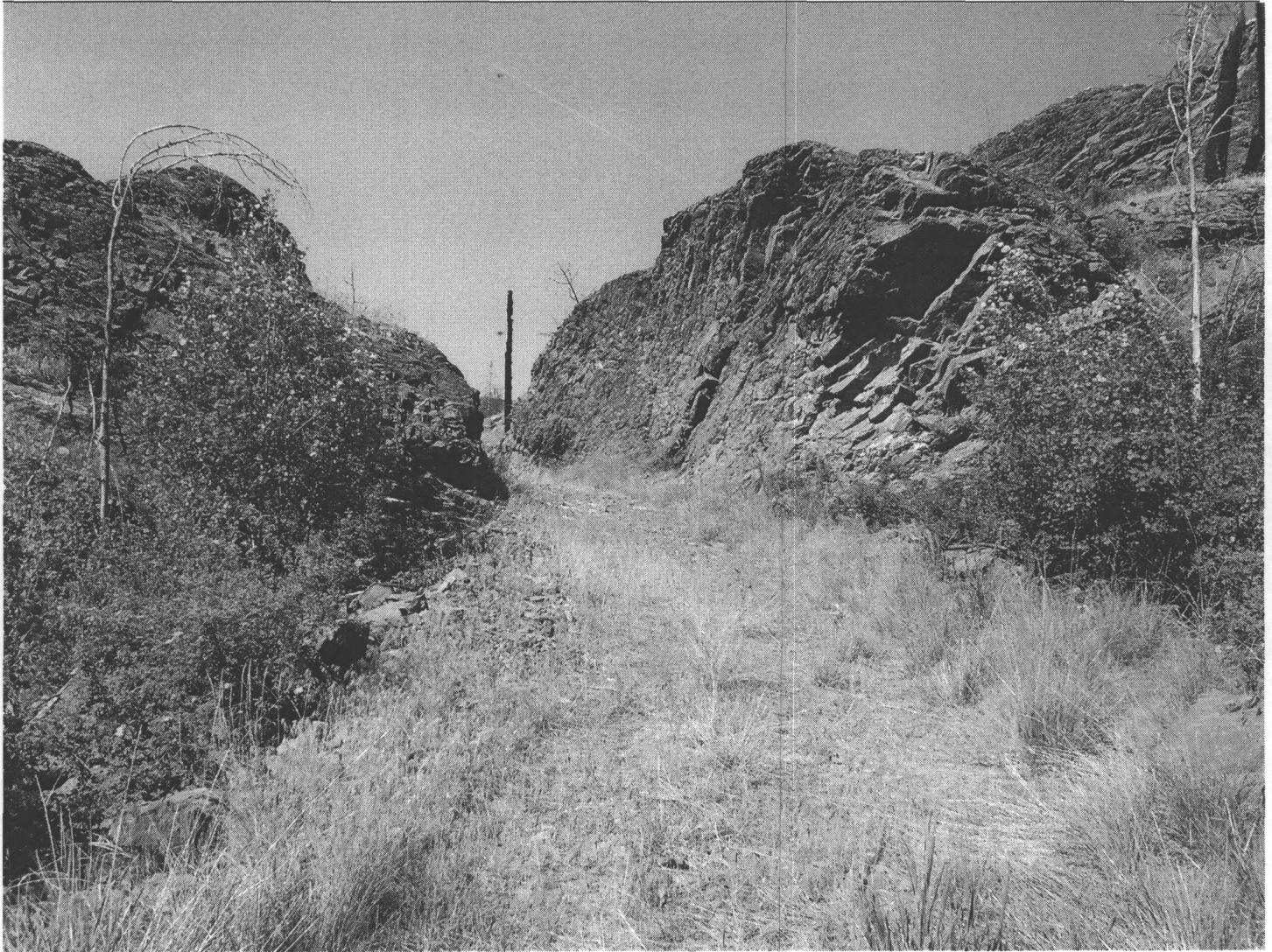
Photo 0015. Section 3. Milwaukee Road RR-built rock cut. View to west.
