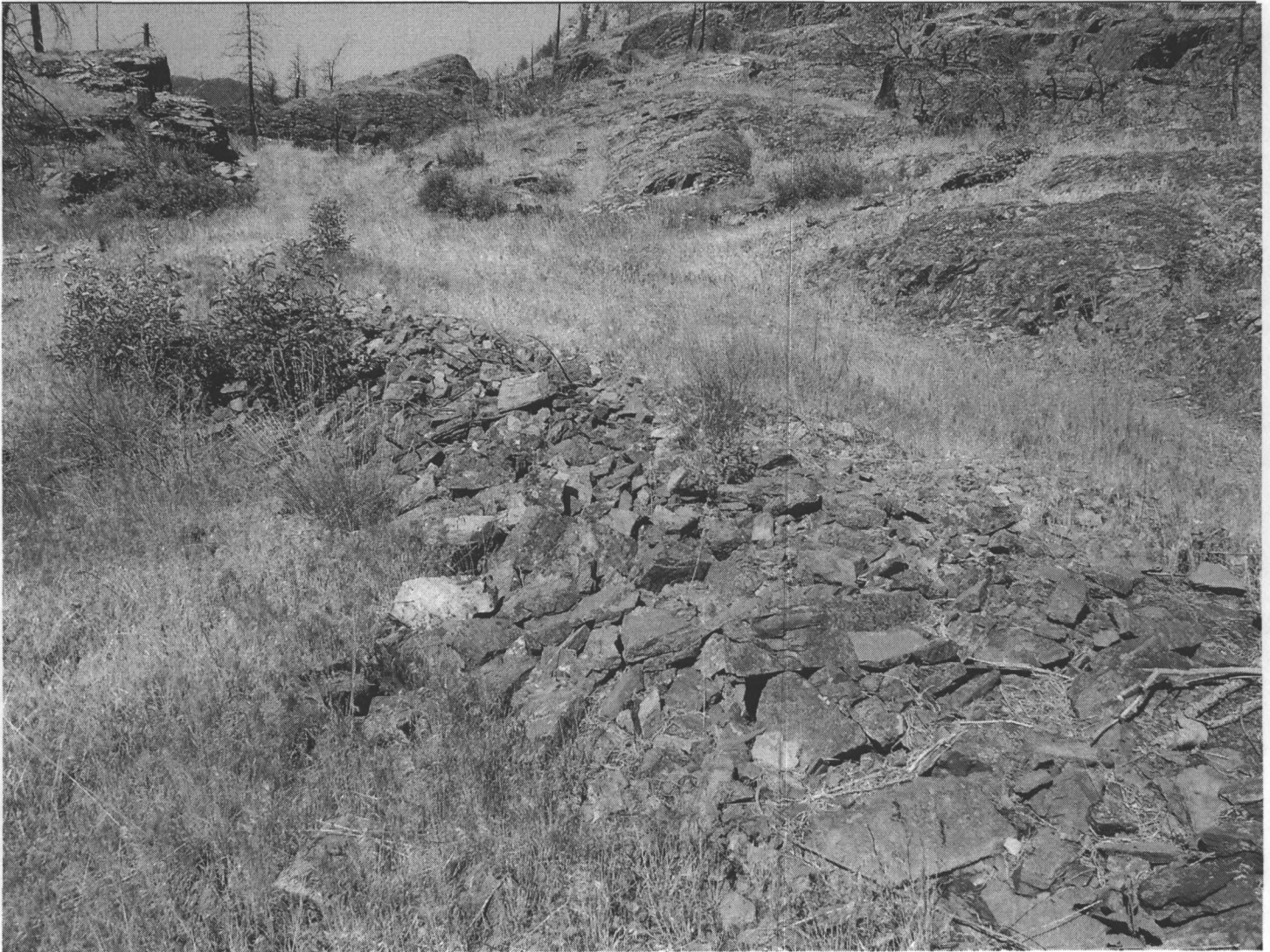
Photo 0036. Section 2. Mullan Road retaining wall. View to west-northwest.
