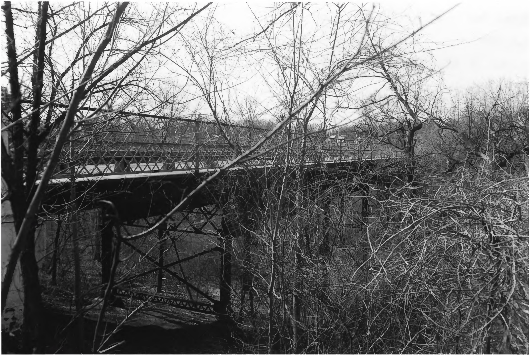
Bridge, MN Soldiers' Home Historic District Hennepin Co, MN 09548/21
