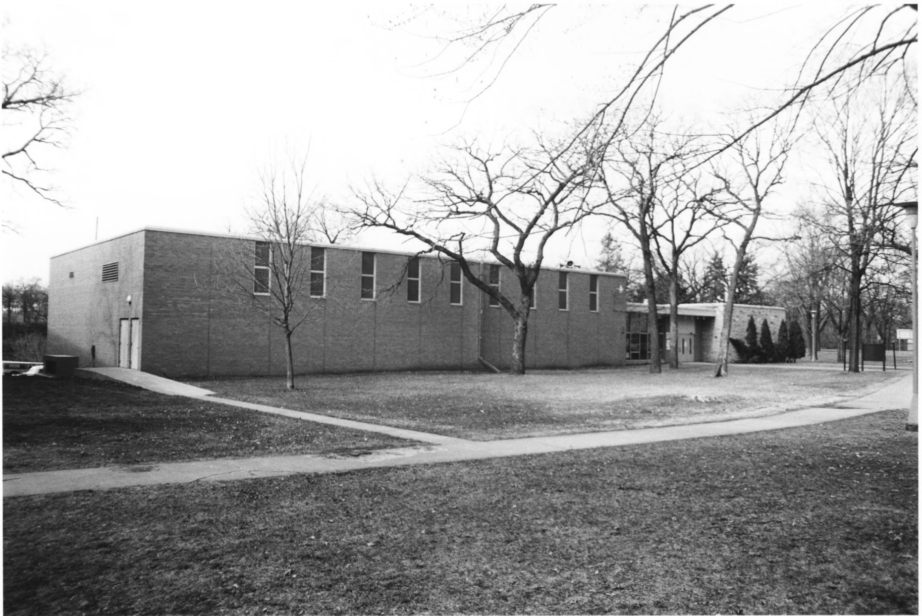
Chapel/Auditorium, MN Soldiers' Home Historic District Hennepin Co, MN 09548/15
