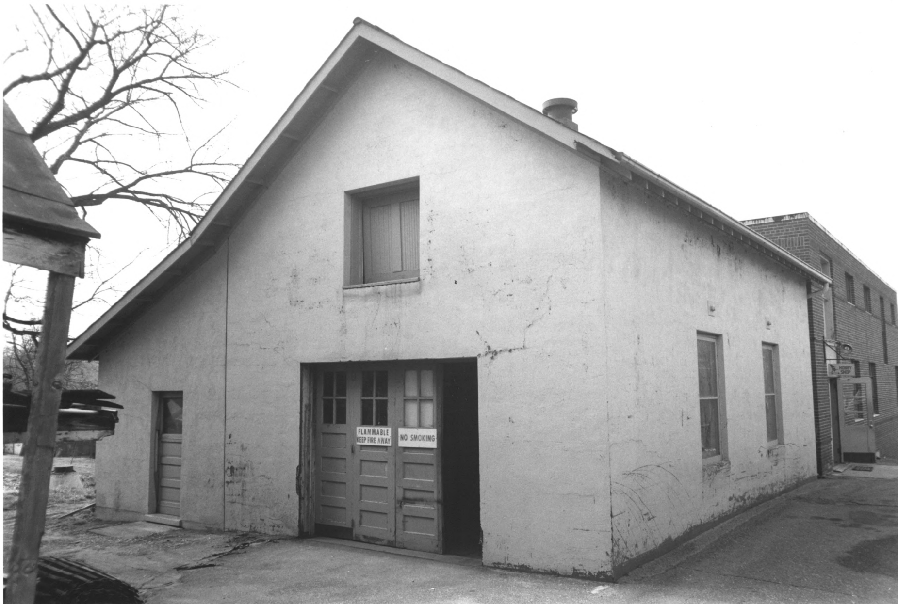
Storage Building, MN Soldiers' Home Historic District Hennepin Co, MN 09548/5
