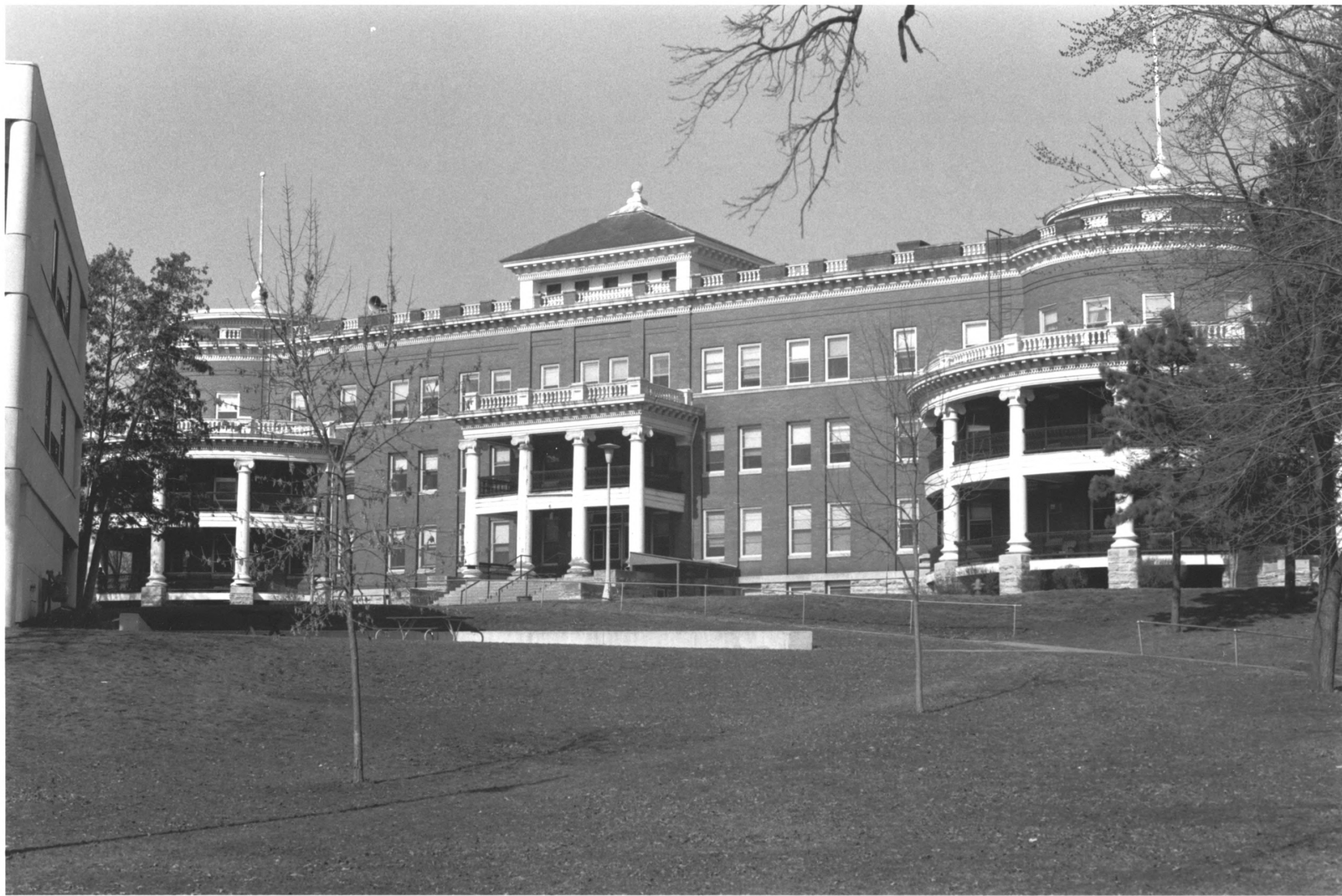
Women's Residence, MN Soldiers' Home Historic District Hennepin Co, MN 09561/8
