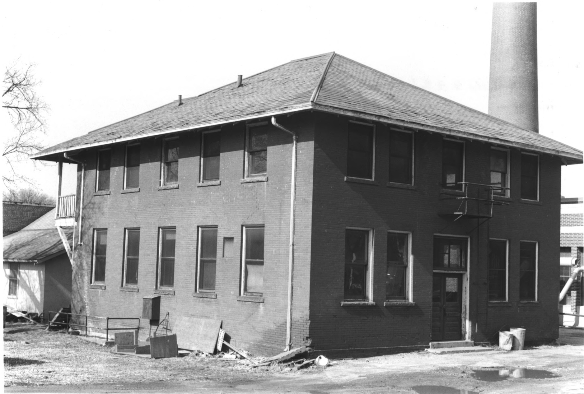
Laundry and Heating Plant, MN Soldiers' Home Historic District Hennepin County, MN 09561/24A
