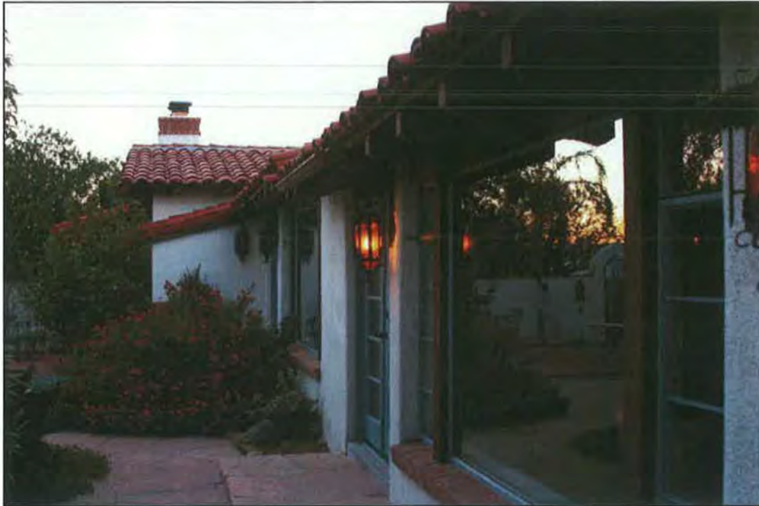
Photograph 3 of 13. Looking northwest, south elevation, elevation details.
