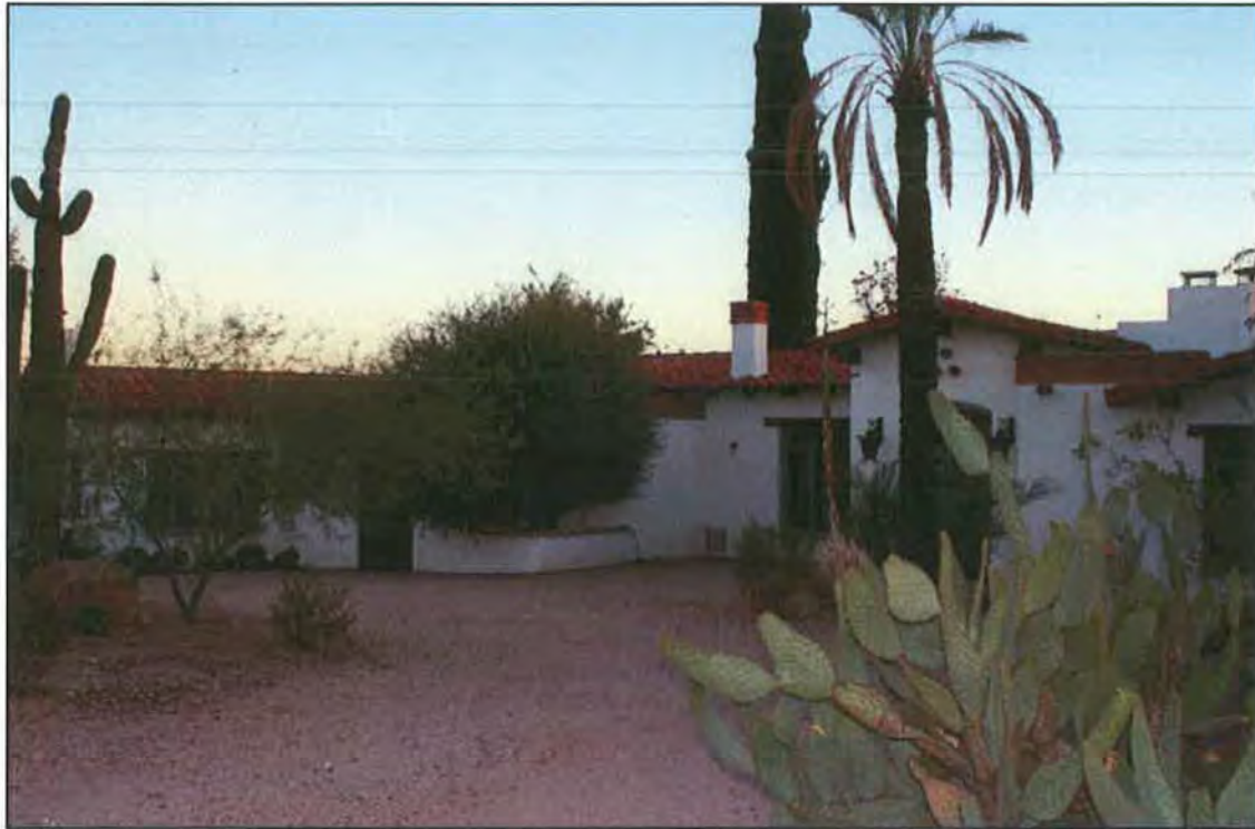
Photograph 1 of 13. Looking south, north elevation.
