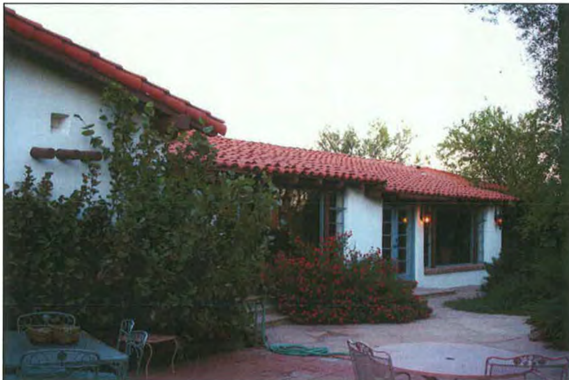
Photograph 2 of 13. Looking northeast, south elevation, enclosed porch
