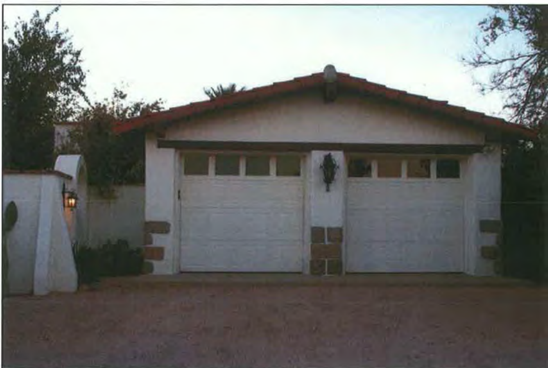
Photograph 6 of 13. Looking west, east elevation, garage details.
