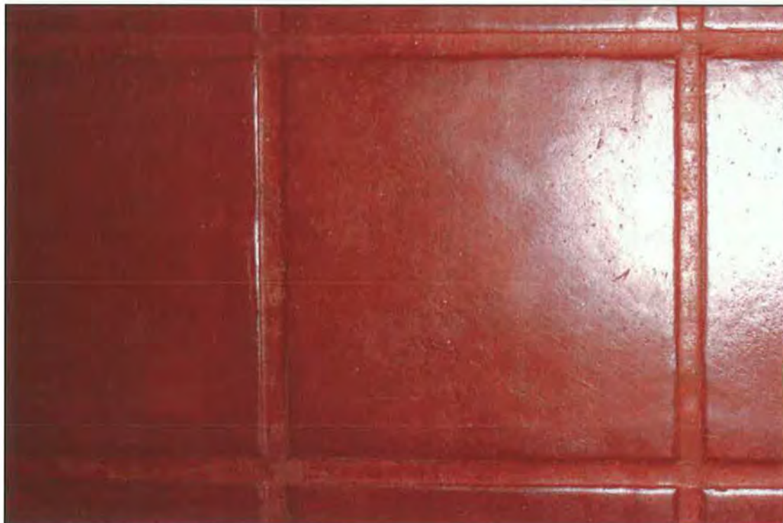
Photograph 13 of 13. Red concrete floor detail.
