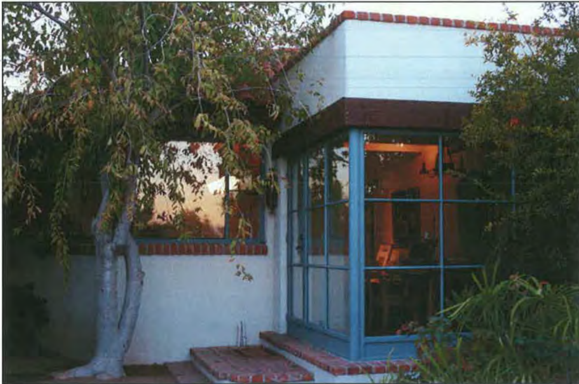
Photograph 8 of 13. Looking northwest, kitchen addition.
