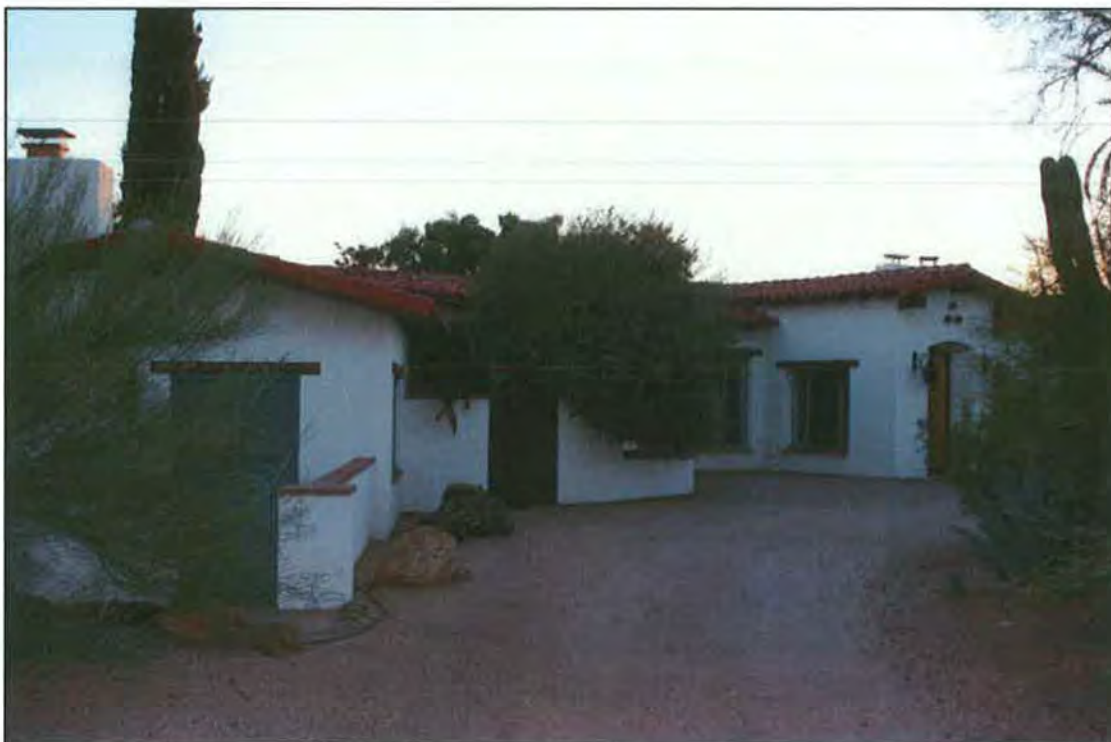
Photograph 5 of 13. Looking southwest, north elevation, elevation details.
