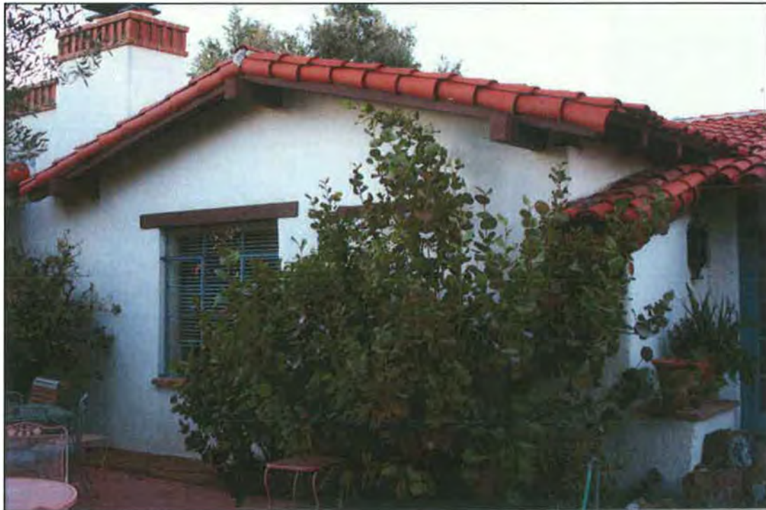
Photograph 4 of 13. Looking north, south elevation, elevation details.
