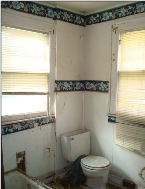
Photo 23. Second Floor bathroom, facing southwest
