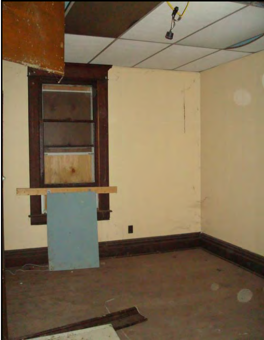
Photo 21. Bedroom in first floor addition, facing south
