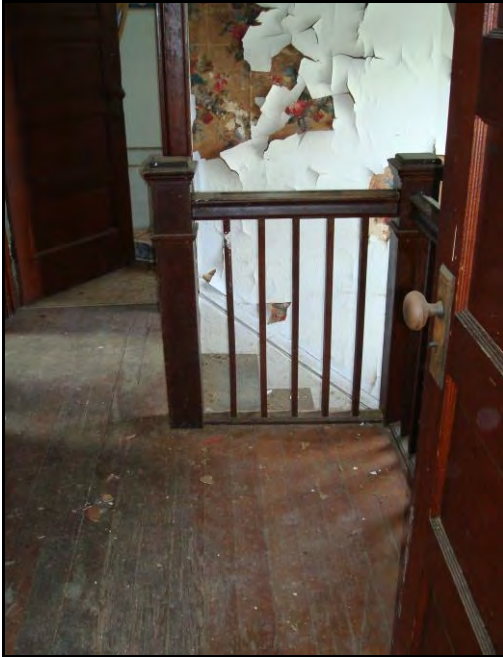
Photo 25. Facing north out of the second floor west/front bedroom. Staircase and landing, facing bath
