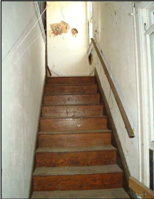
Photo 11. Staircase from first floor entry to second floor.
