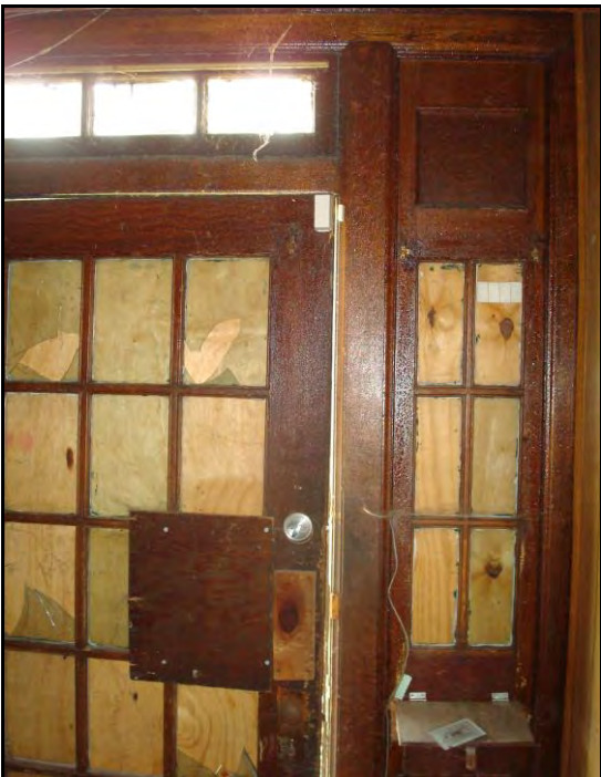
Photo 8. Entry door with sidelight and transom, first floor interior.
