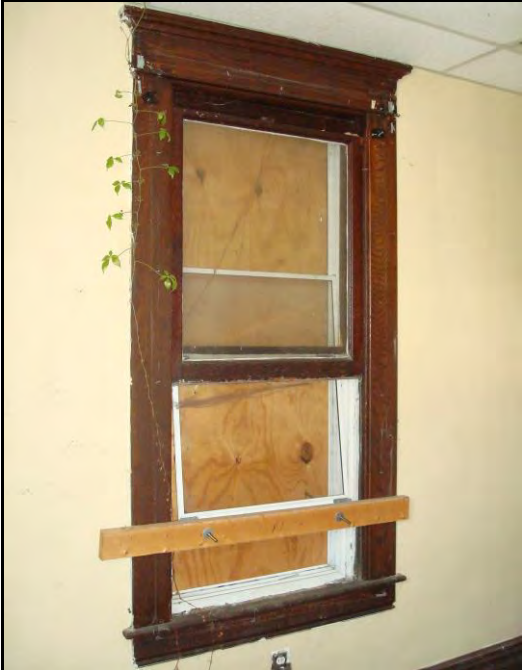
Photo 14. Living room window with original molding, first floor interior, facing east
