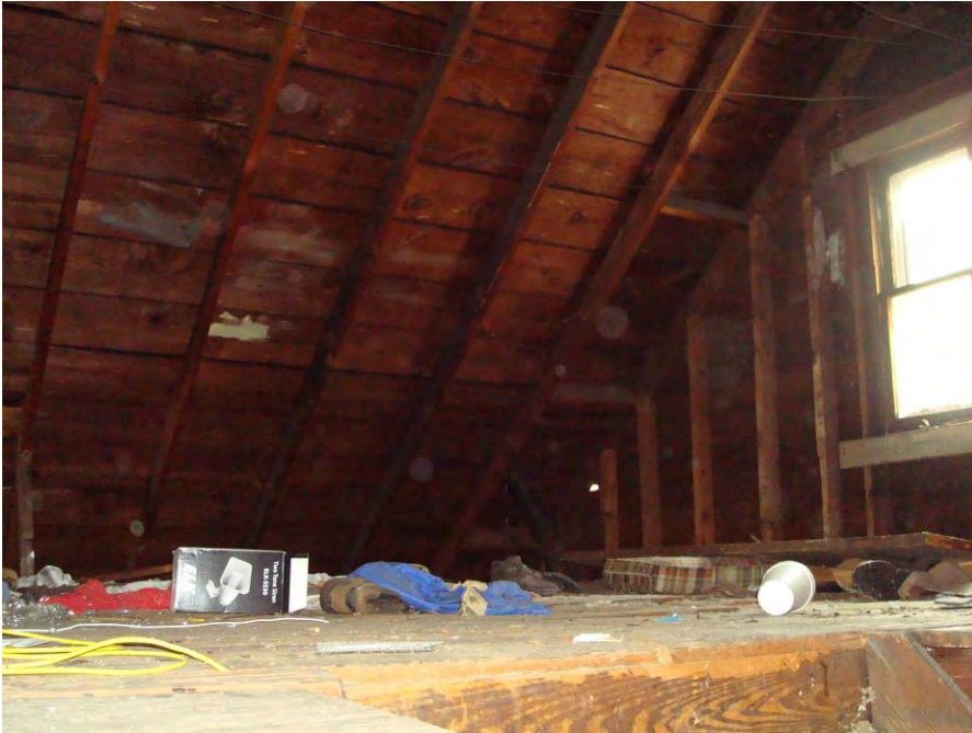
Photo 27. Attic, facing northeast.
