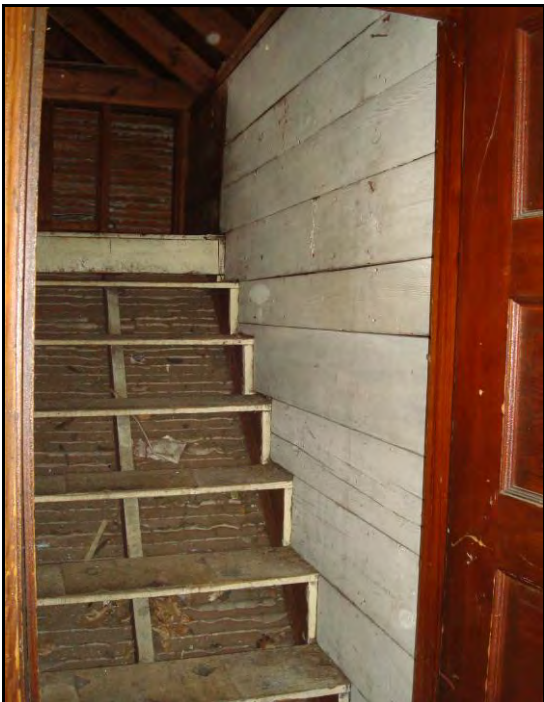
Photo 26. Attic Stair in western front bedroom, facing north
