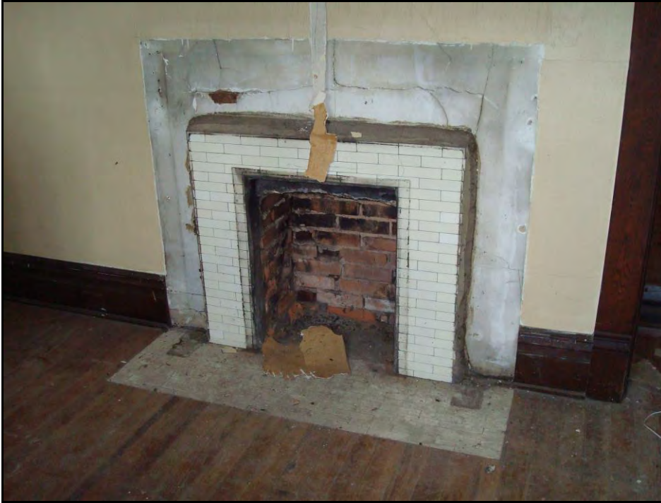
Photo 15: Tile-clad fireplace in living room, first floor interior, facing south
