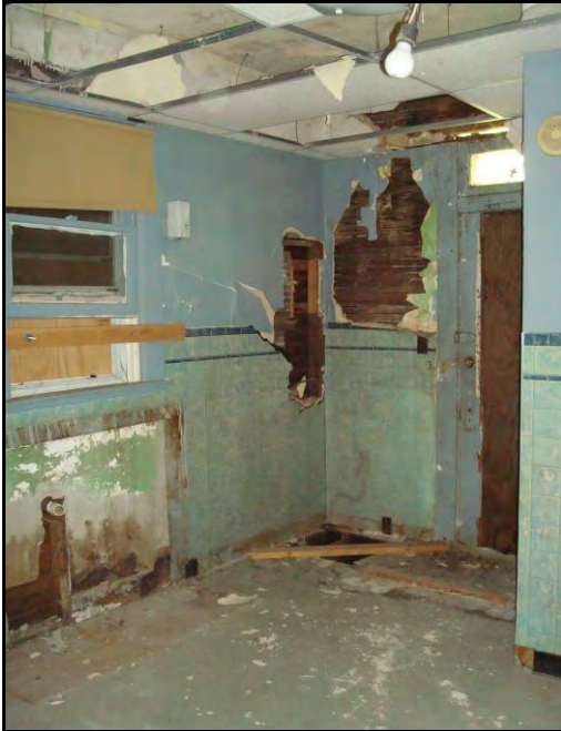
Photo 19. First floor kitchen addition, facing southeast
