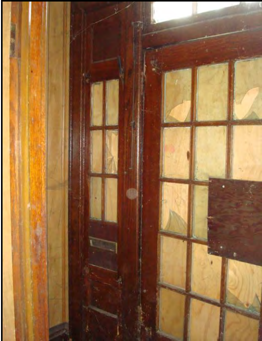
Photo 9. Western side of entry door with sidelight and transom, first floor interior.
