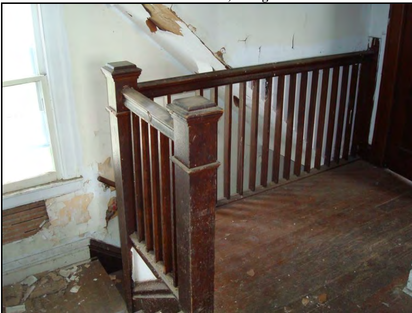
Photo 22. Original staircase balustrade, second floor, facing west
