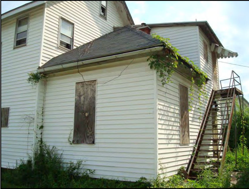
Photo 7. Back of dwelling, facing Southwest on 17 th Street
