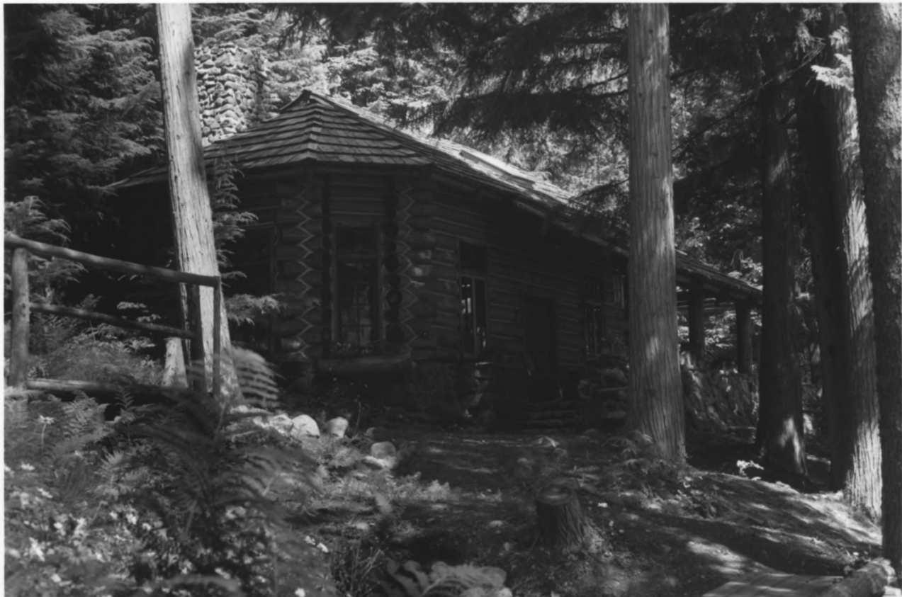
Sherwood Lodge (main cabin) Glacier National Park, Flathead County, Montana Photograph No. 2
