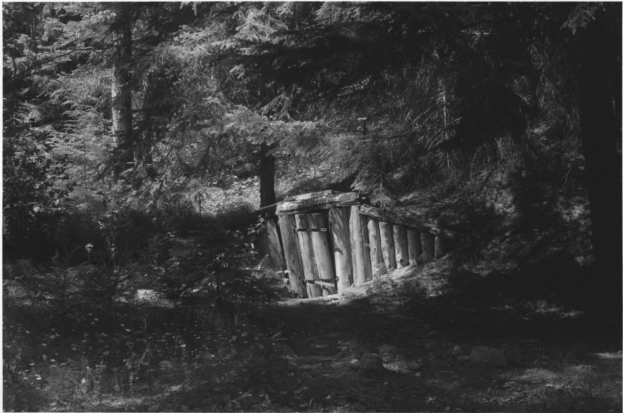
Septic pump house, Sherwood Lodge Glacier National Park, Flathead County, Montana Photograph No. 5
