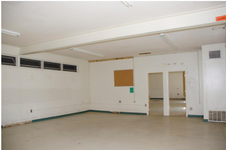
Photo 36: Interior of junior high, looking south at classroom
