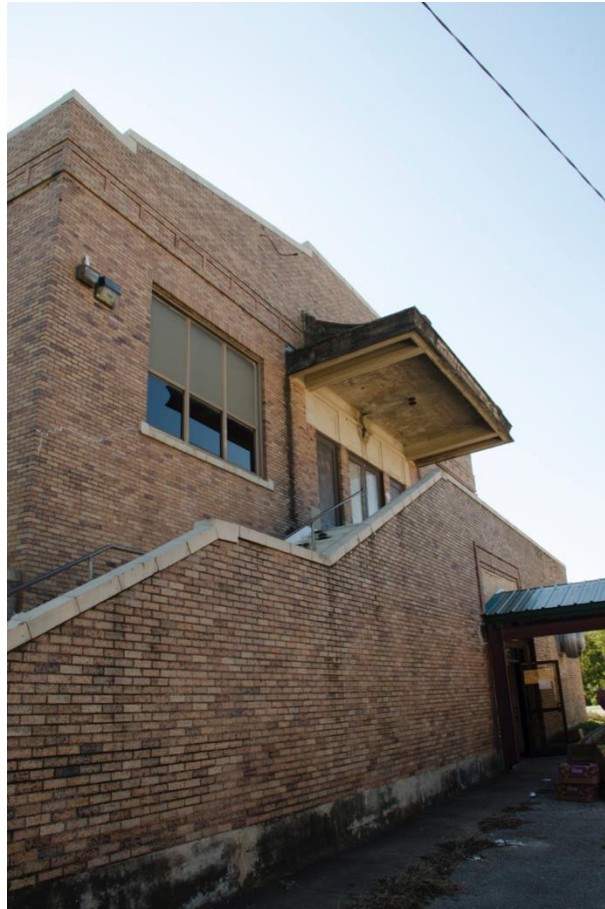
Photo 8: North elevation of auditorium, looking southwest
