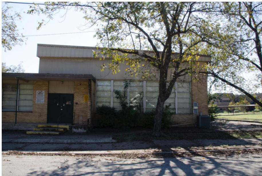
Photo 30: North elevation of junior high, looking south
