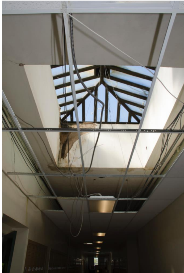
Photo 20: Second floor, detail of skylight, looking west
