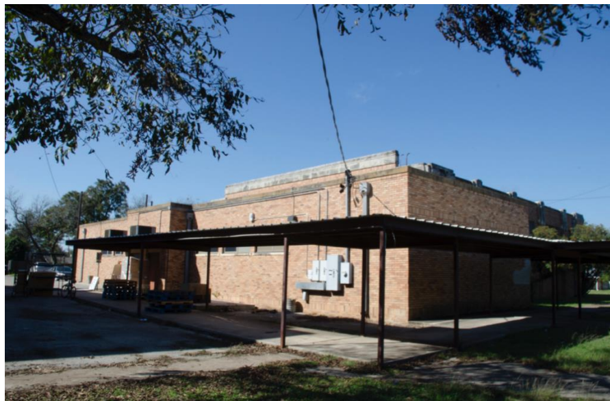
Photo 26: South elevation of gymnasium, looking northwest
