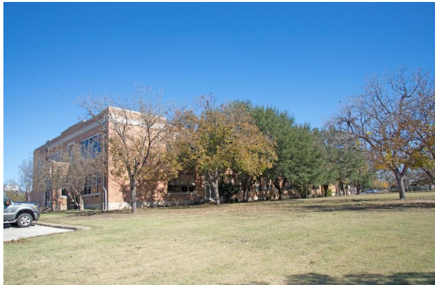
Photo 3: South and west elevation, looking northeast
