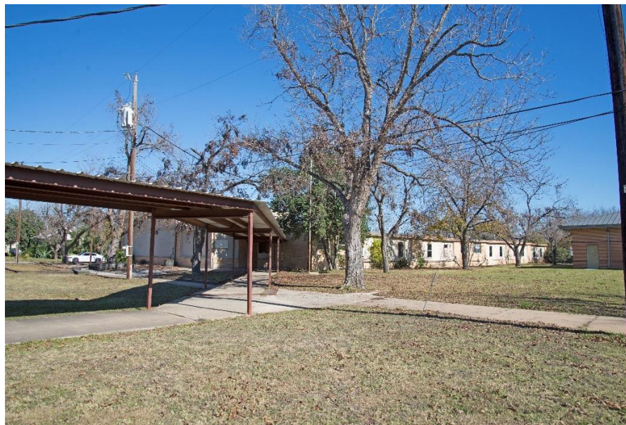
Photo 33: South elevation of junior high, looking northeast
