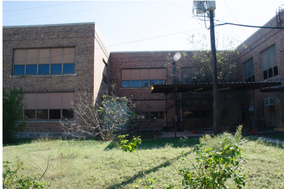
Photo 7: North elevation, looking south
