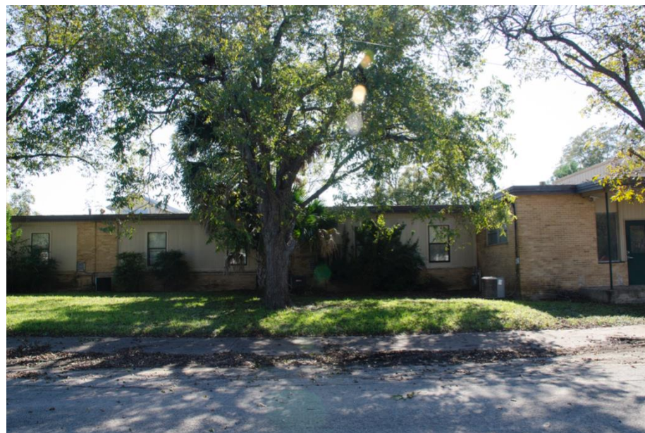
Photo 31: North elevation of junior high, looking south
