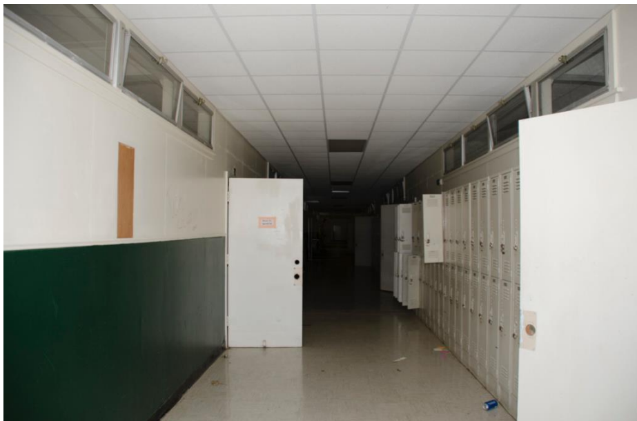
Photo 37: Interior of junior high, looking east
