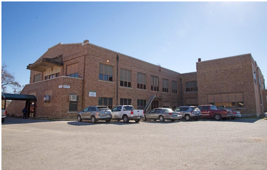
Photo 11: North and west elevation of auditorium, and partial north elevation of high school looking south
