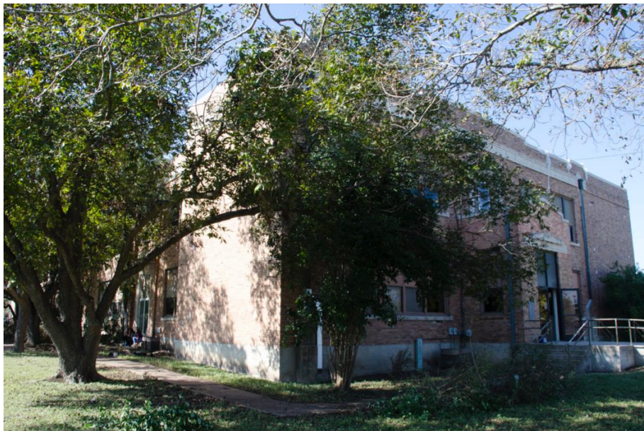
Photo 6: East and south elevations, looking northwest
