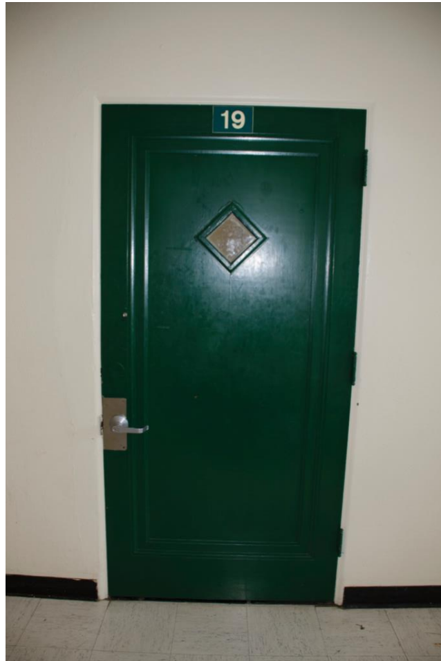
Photo 18: Second floor, detail of door, looking north
