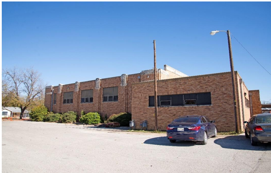
Photo 24: West elevation of gymnasium, looking east
