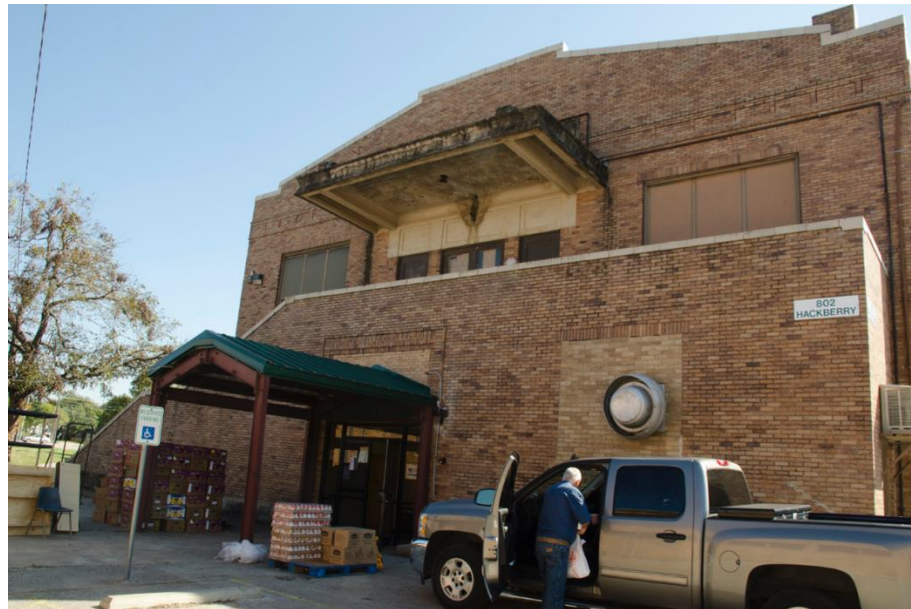
Photo 9: North elevation of auditorium, looking south
