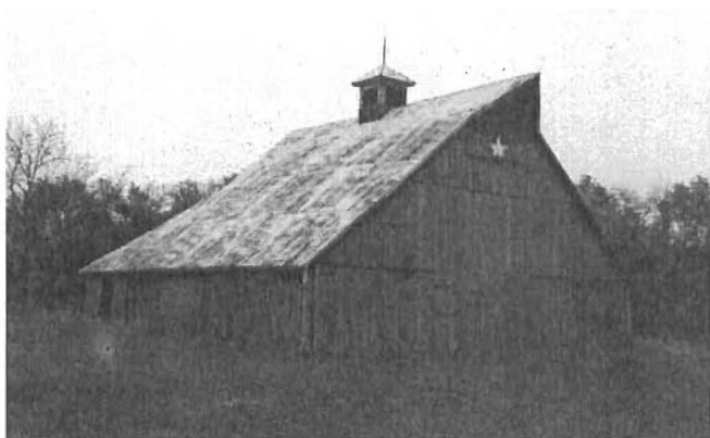
Figure 50: Midwest Prairie Barn in Coffey County. Brenda Spencer.
