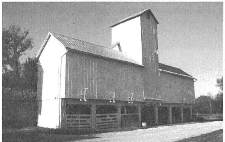
Figure 54: Granary (on-farm grain elevator) in Pottawatomie County. Brenda Spencer.
