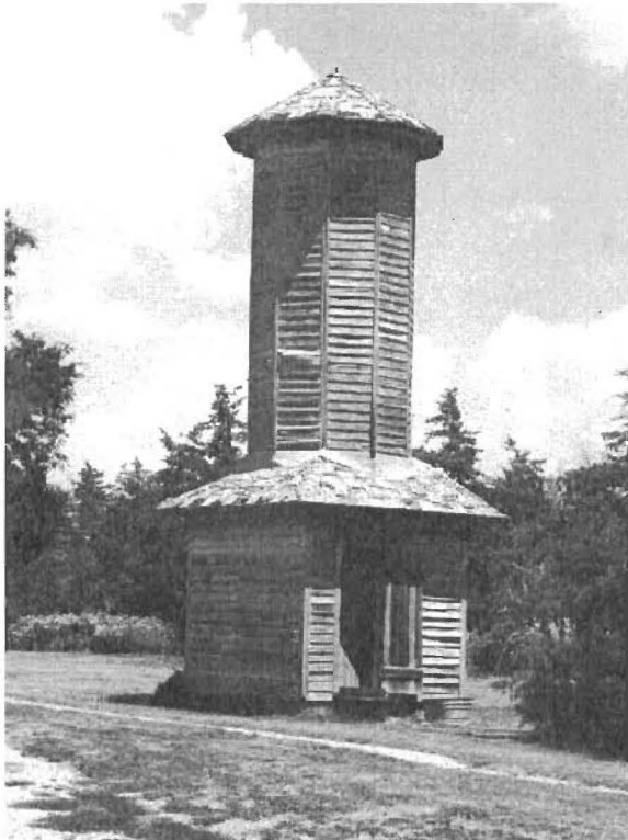
Figure 62: Tankhouse in Decatur County. Brenda Spencer.
