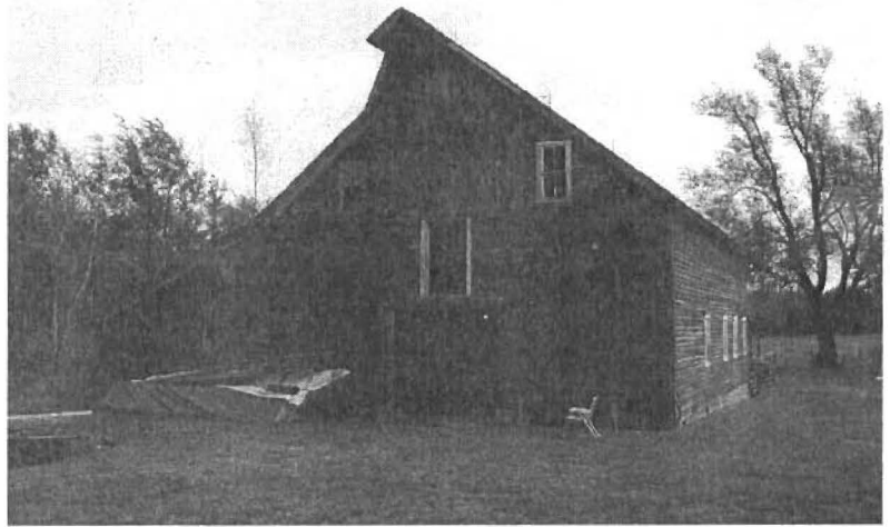
Figure 42: Gable-Roof Barn in Marion County. Brenda Spencer.
