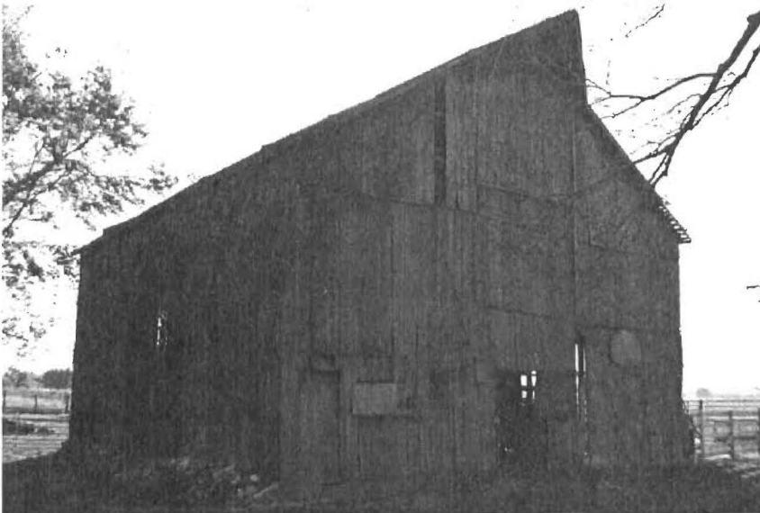
Figure 41: Gable-Roof Barn in Anderson County. Susan Ford.
