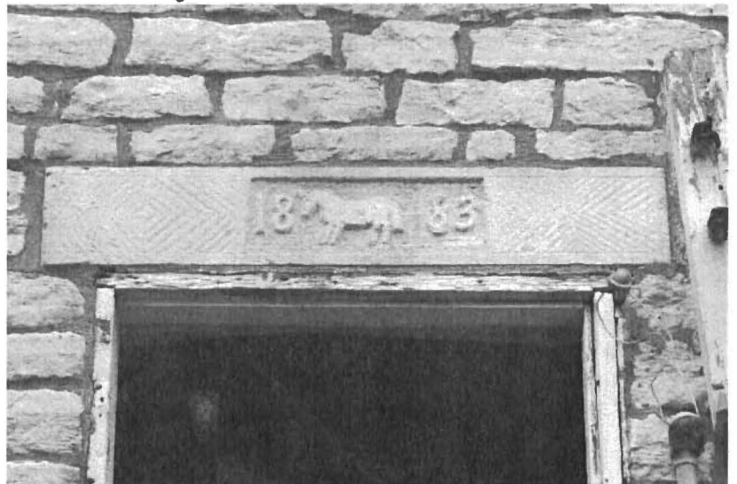
Figure 31: Intricate stonework in doorway of barn. Brenda Spencer.
