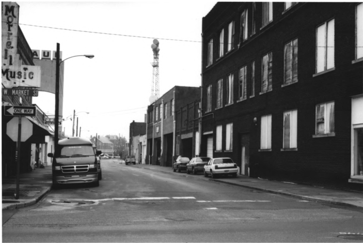
JOHNSON CITY WAREHOUSE & COMMERCE - HISTORIC DISTRICT WASHINGTON COUNTY TN 5 OF 8
