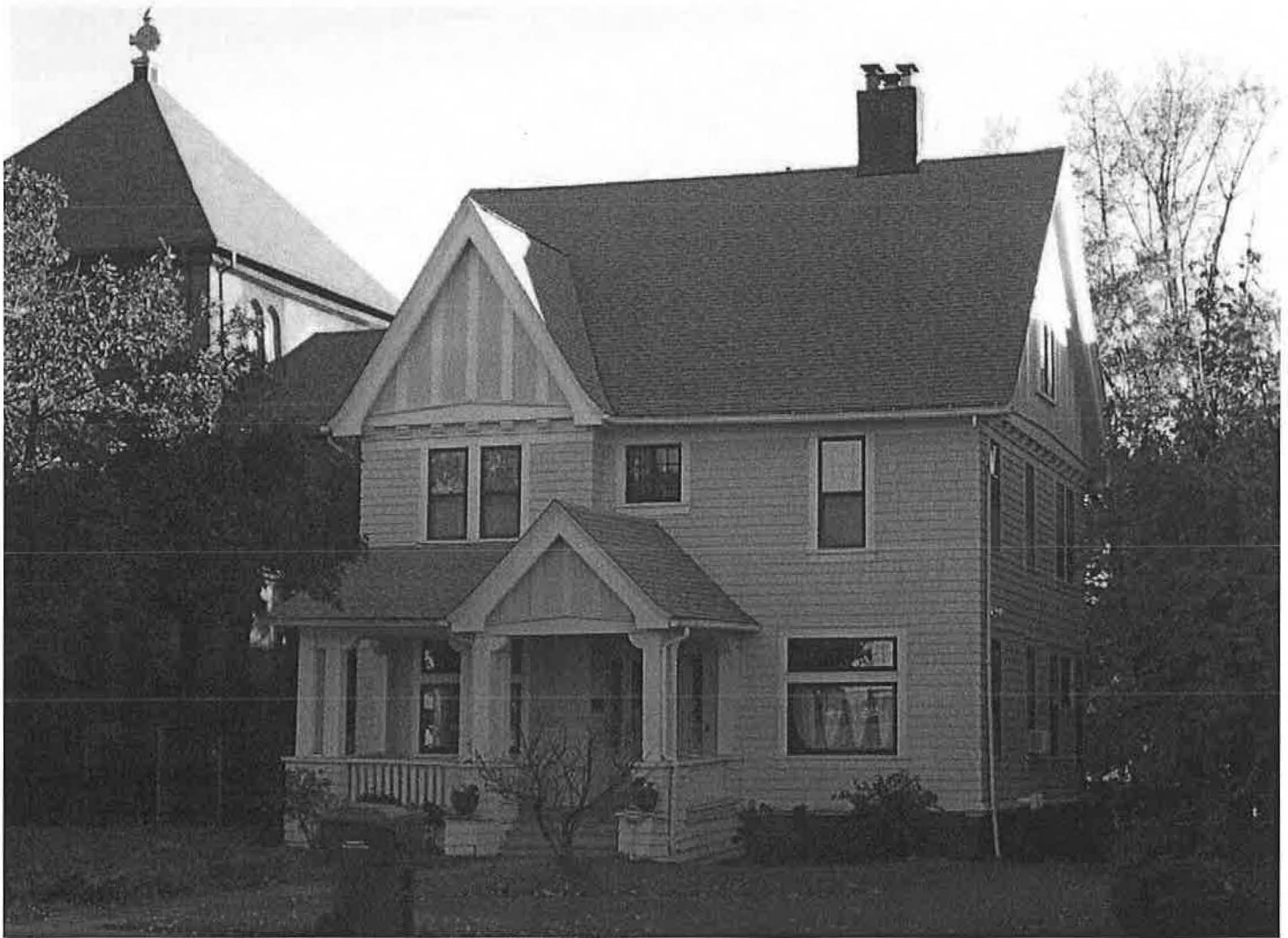
North (front) and west (side) elevations of 573 Farmington Avenue, 1904, showing façade, roof, porch, and window details.
