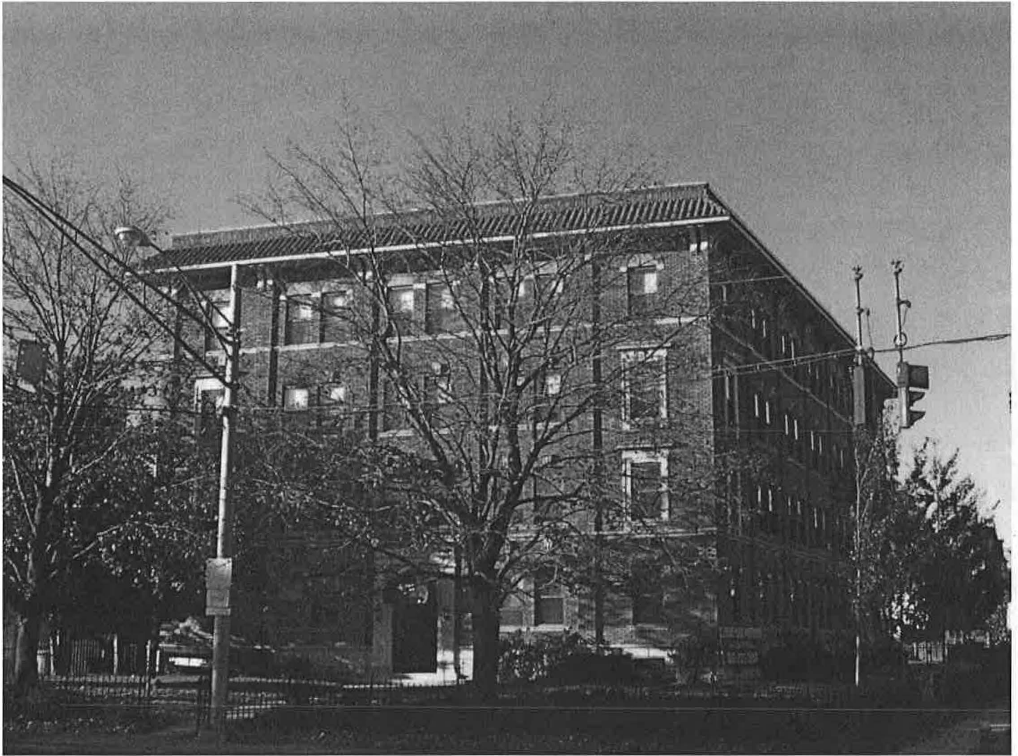
South (front) and east (side) elevations of 476-478 Farmington Avenue, 1917, showing façade, roof, entry, and window details.
