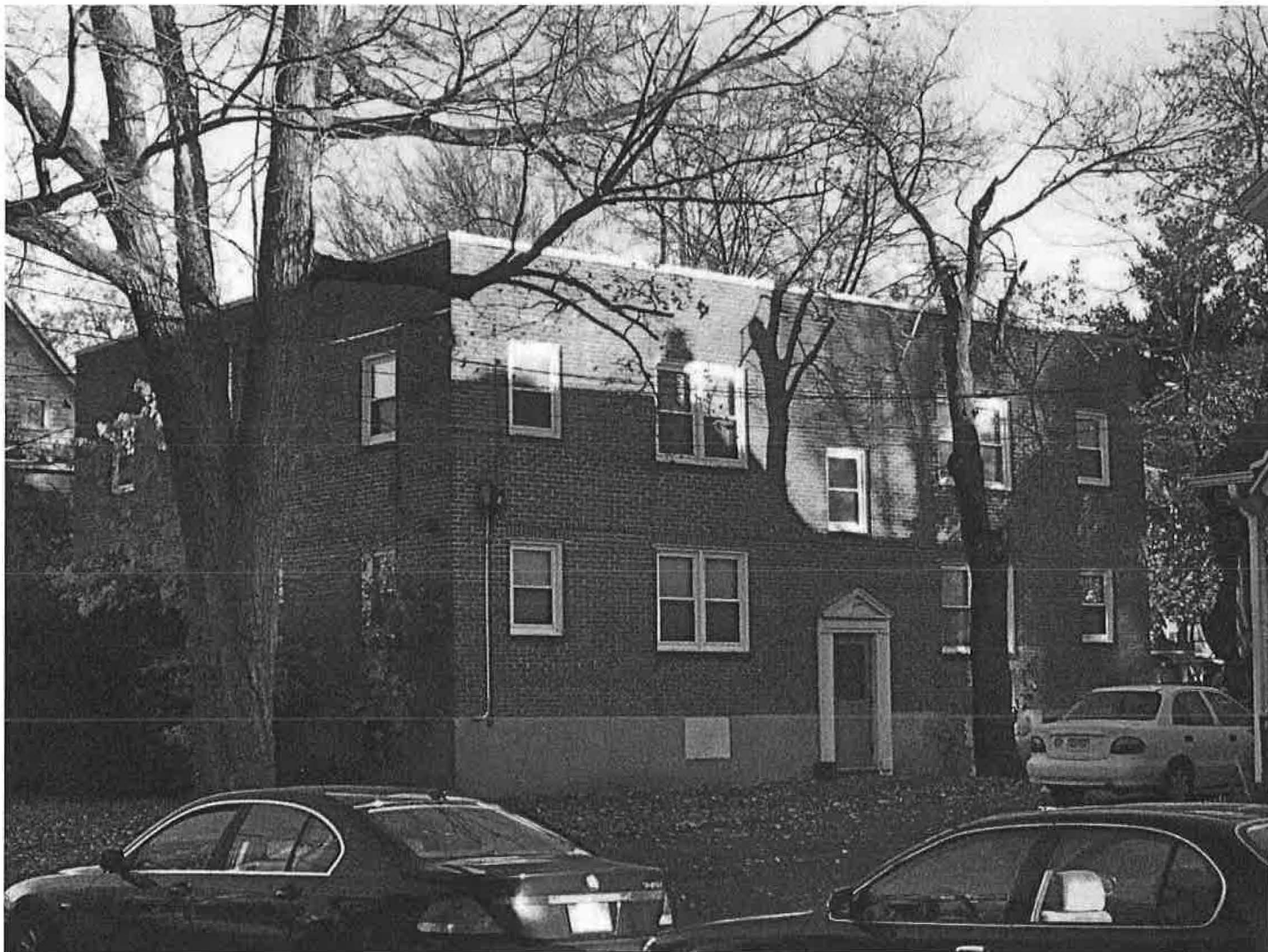
West (front) and north (side) elevations of 5 Gray Street, 1954, showing façade, roof, entry, and window details.
