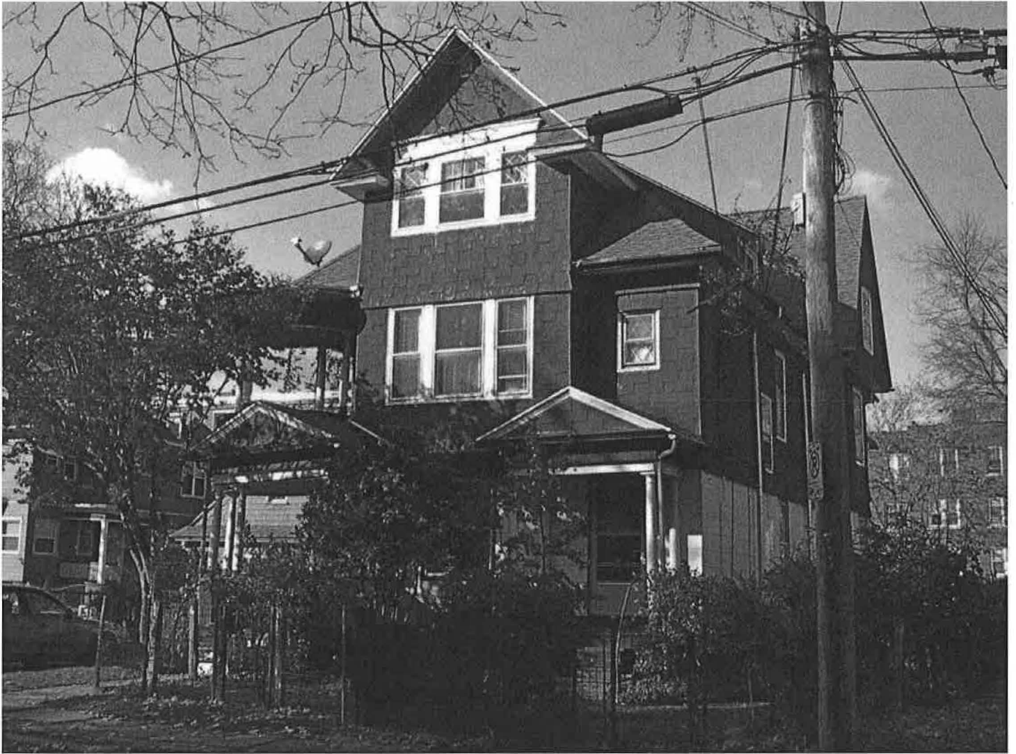
South (front) and east (side) elevations of 14-16 Fales Street, 1899, showing façade, roof, porch, and window details.
