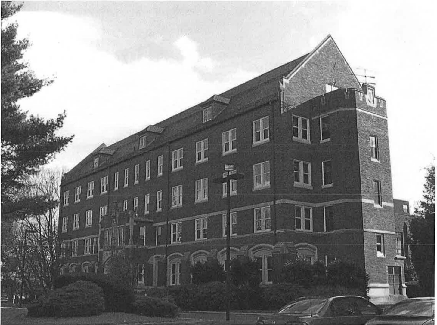
North (front) and west (side) elevations of 170 Sisson Avenue, 1930, showing façade, roof, entry, and window details.
