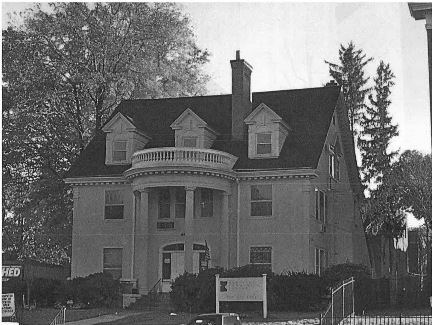
North (front) and west (side) elevations of 461 Farmington Avenue, 1907, showing façade, roof, porch, and window details.
