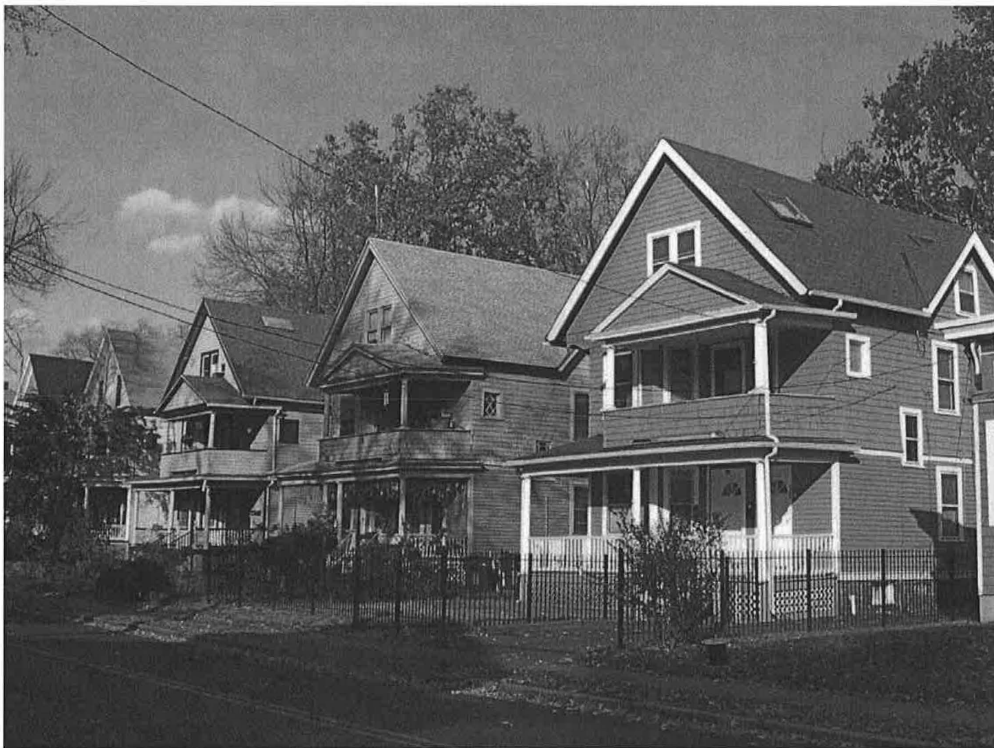
West (front) and south (side) elevations of 190-192, 194-196, 198-200, 202-204, and 206-208 South Whitney Street; 1907, 1907, 1907, 1905, and 1905; showing façade, roof, porch, and window details. Camera facing northeast. Photograph 12 of 37.
