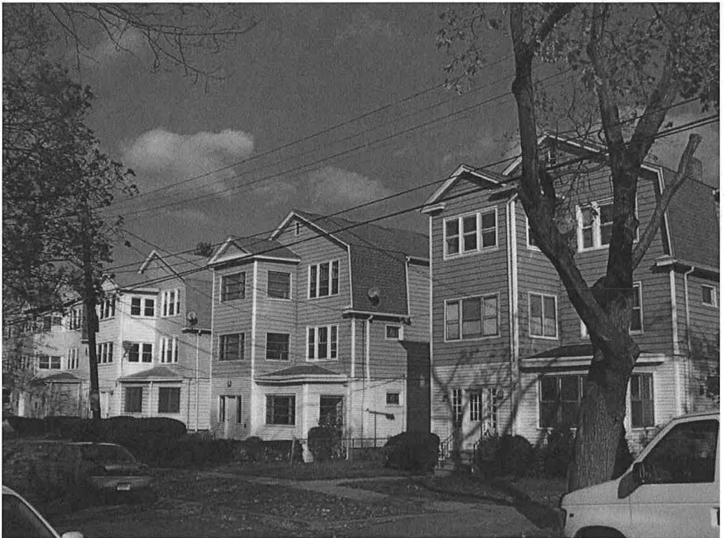
West (front) and south (side) elevations of 120-122, 124-126, 128-130, 132-134 Evergreen Avenue; 1925, 1926, 1926, and 1926; showing façade, roof, porch, and window details. Camera facing northeast. Photograph 16 of 37.
