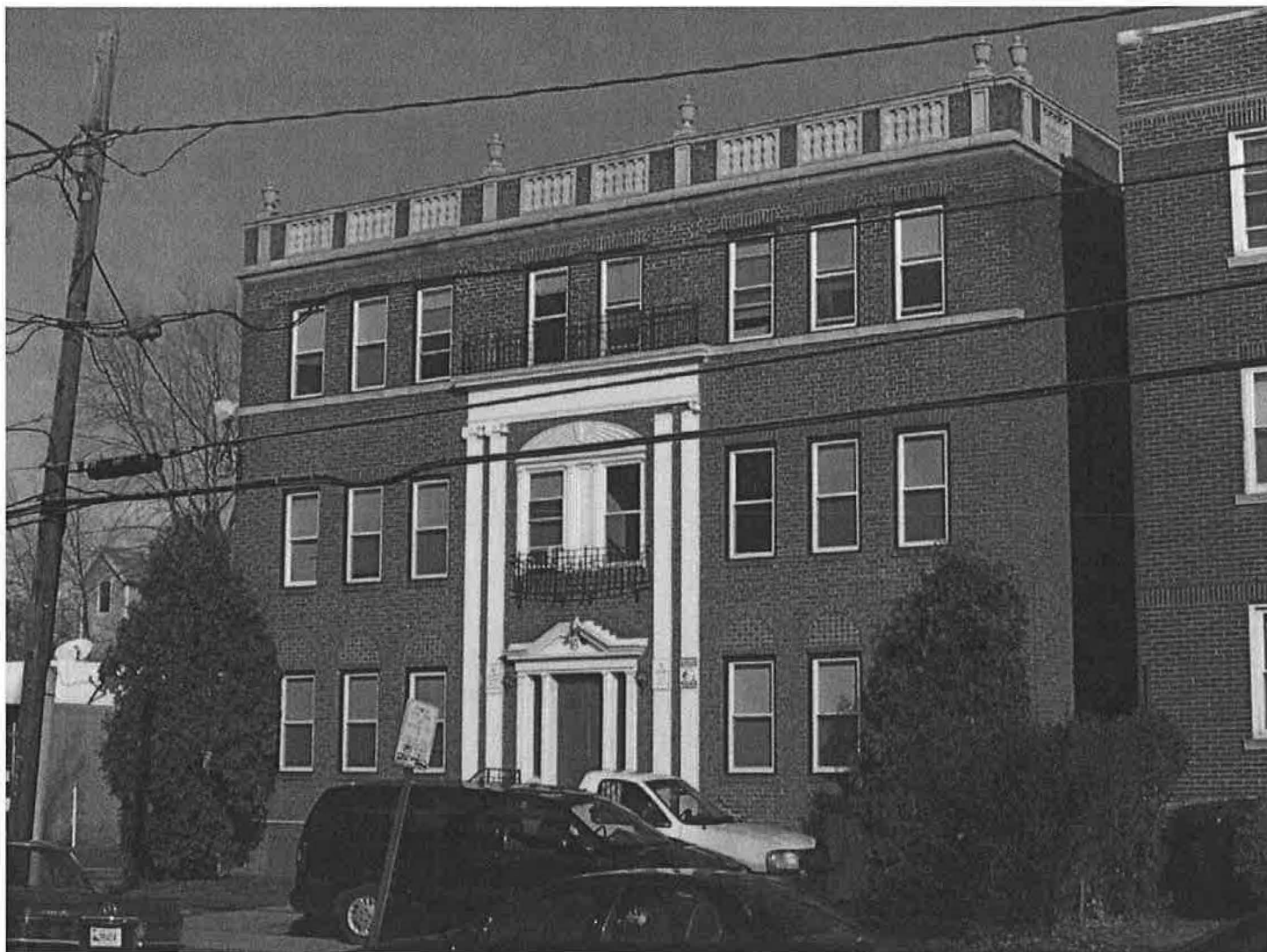
West (front) and south (side) elevations of 16 Evergreen Avenue, 1927, showing façade, roof, entry, and window details.
