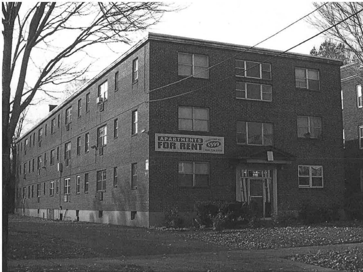
East (front) and south (side) elevations of 21 Evergreen Avenue, 1958, showing façade, roof, entry, and window details.
