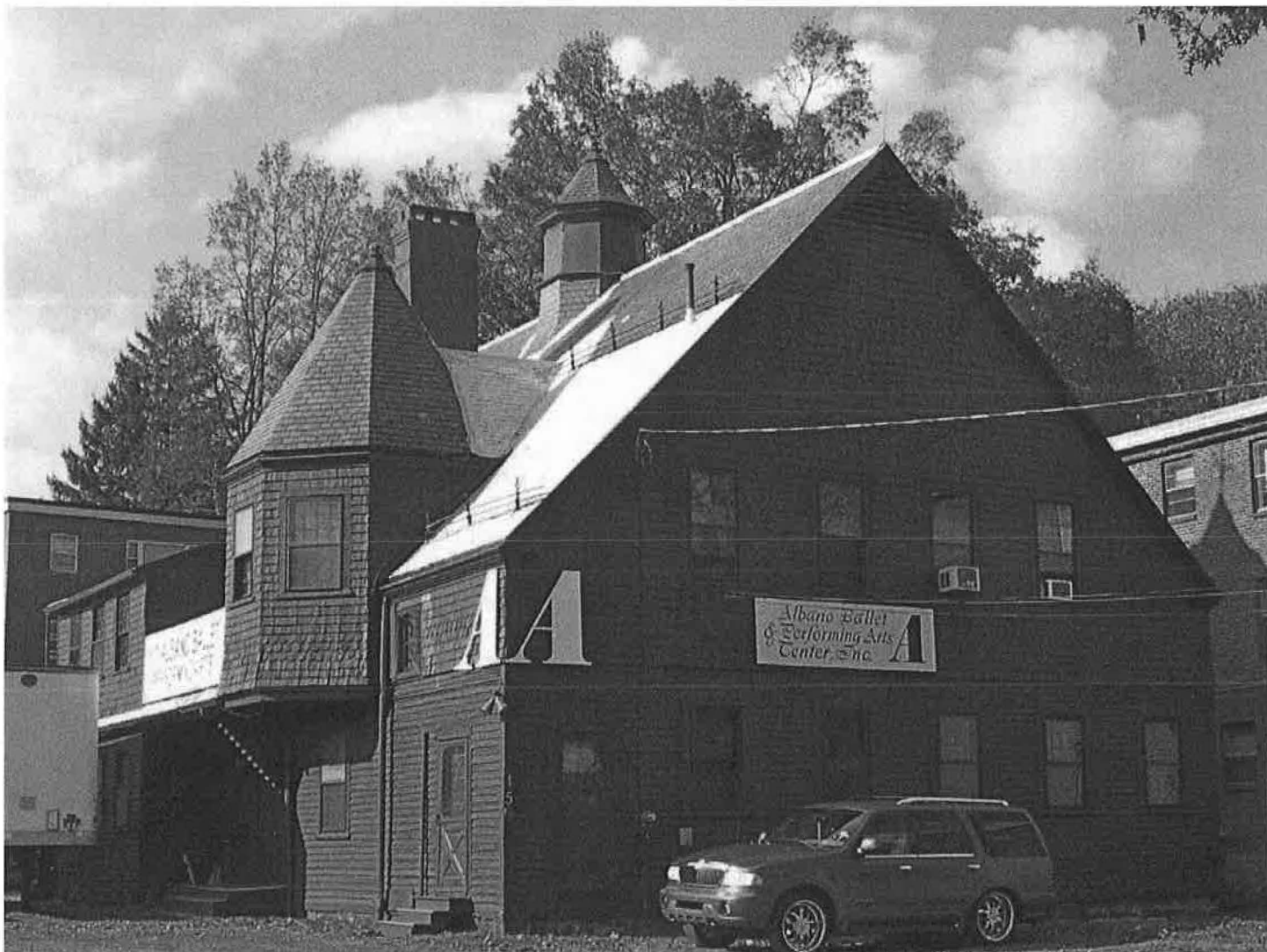
South (front) and east (side) elevations of 15 Girard Avenue, 1888, showing façade, roof, turret, and window details.
