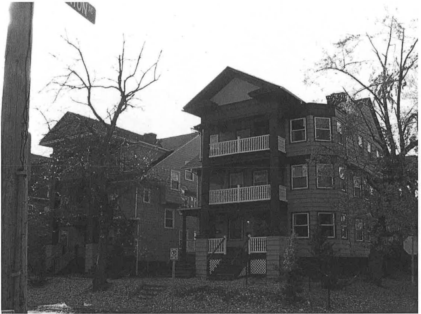
East (front) and north (side) elevations of 163-165 and 167-169 Sisson Avenue, 1915, showing façade, roof, porch, and window details. Camera facing southwest. Photograph 18 of 37.
