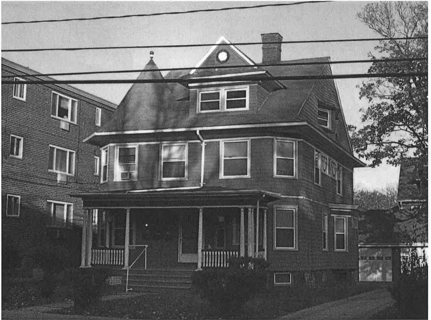
West (front) and south (side) elevations of 34 Evergreen Avenue, 1900, showing façade, roof, porch, and window details.
