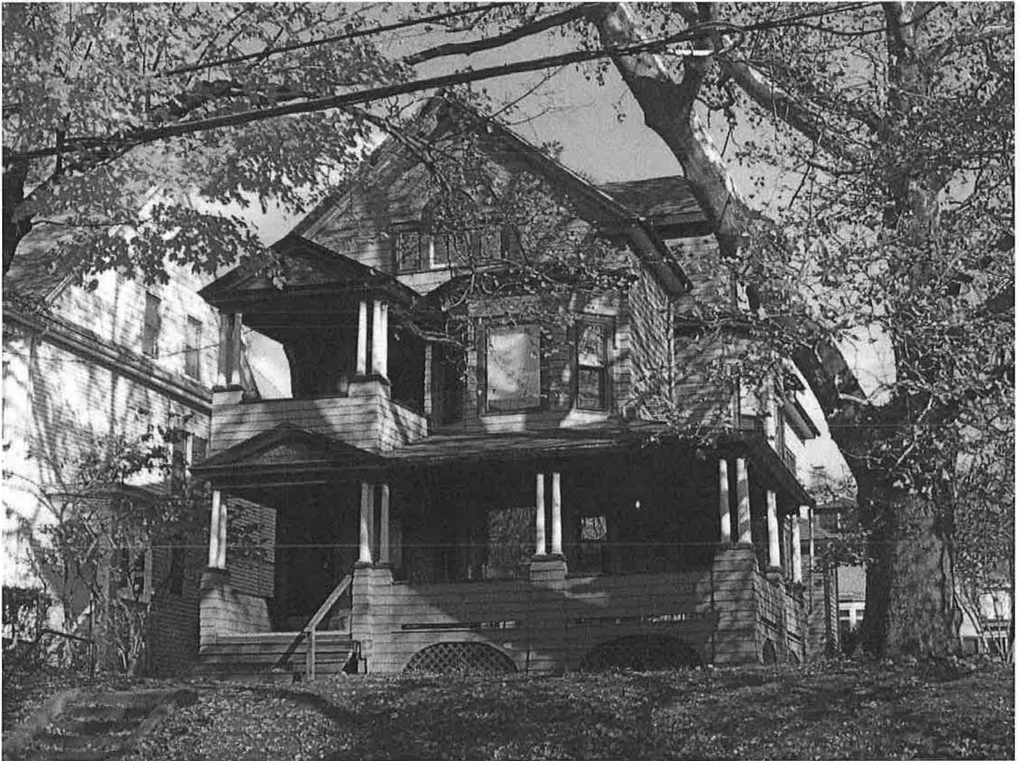
West (front) and south (side) elevations of 94-96 Evergreen Avenue, 1908, showing façade, roof, porch, and window details. Camera facing northeast. Photograph 11 of 37.
