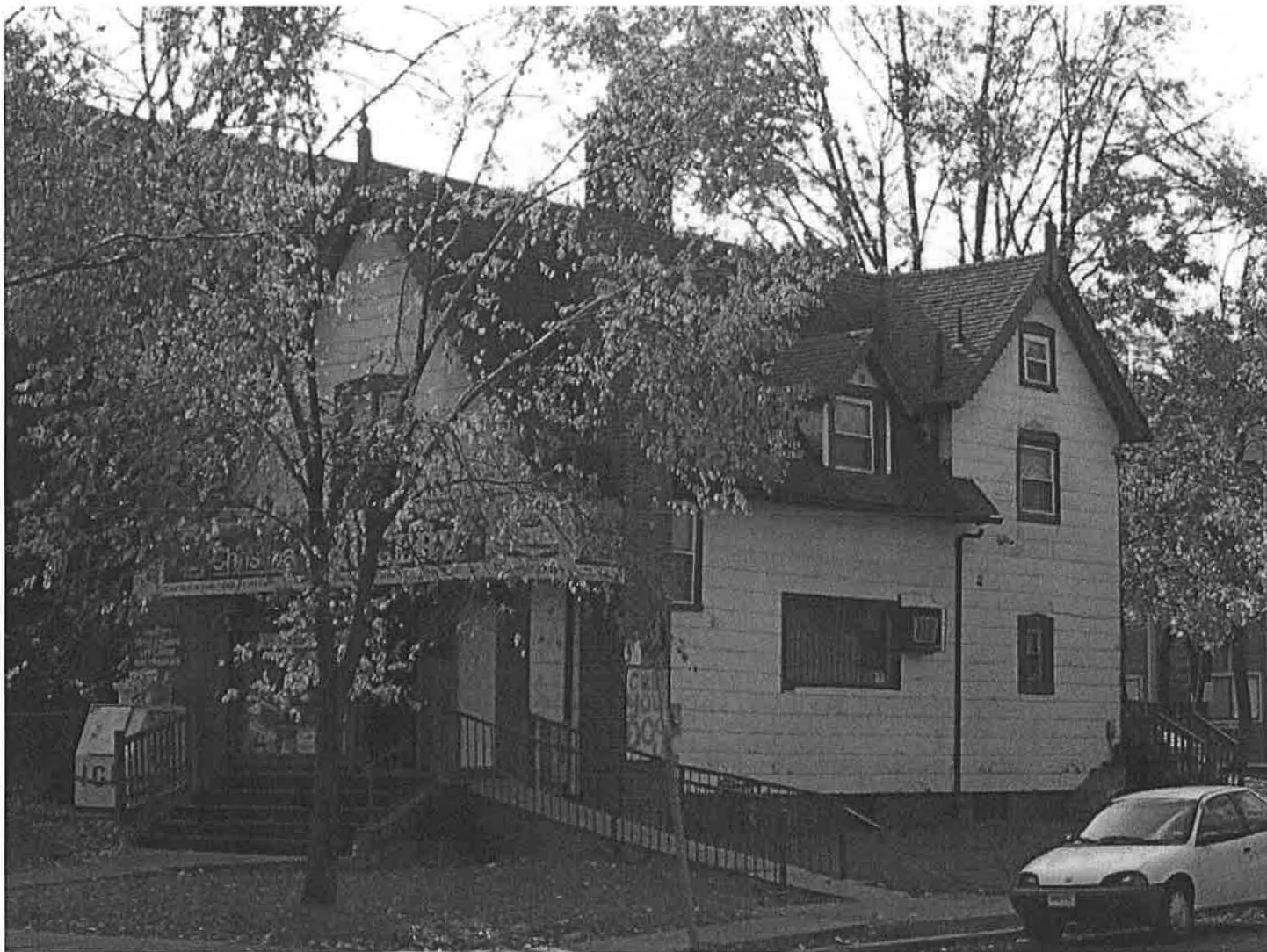
East (front) and north (side) elevations of 227 Sisson Avenue, c. 1890, showing façade, roof, porch, and window details.
