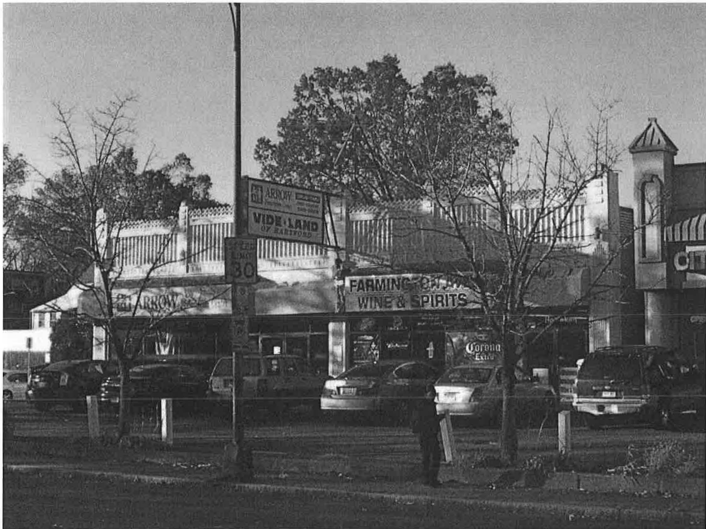
South (front) and east (side) elevations of 500-506 Farmington Avenue, 1933, showing façade, roof, parapet, and window details.
