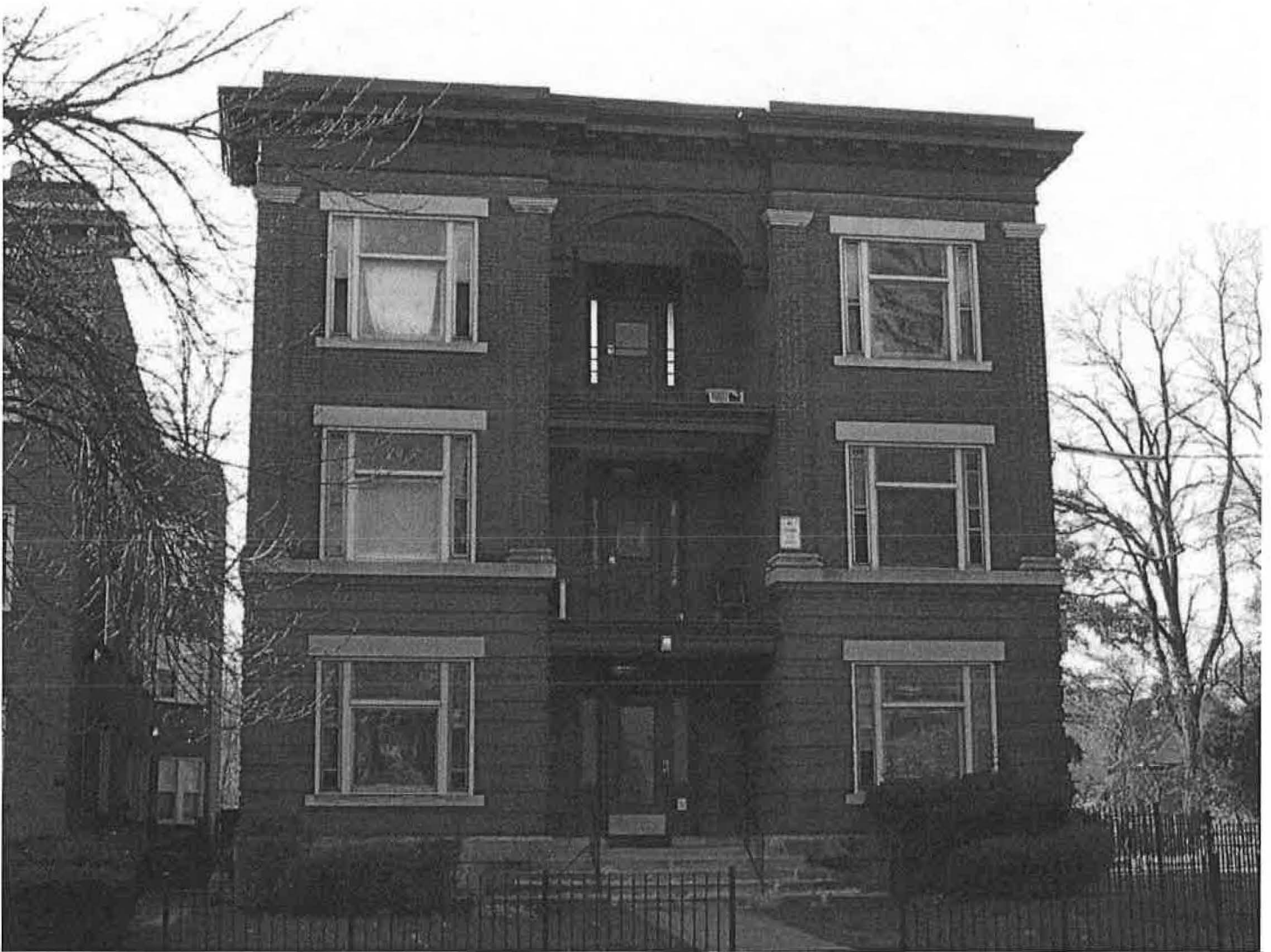
East (front) elevation of 53-55 Evergreen Avenue, 1908, showing façade, roof, porch, and window details. Camera facing west. Photograph 21 of 37.
