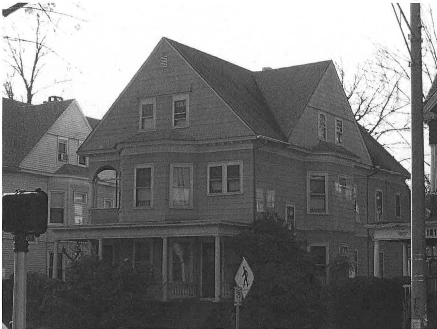
East (front) and north (side) elevations of 177-179 Sisson Avenue, 1904, showing façade, roof, porch, and window details.
