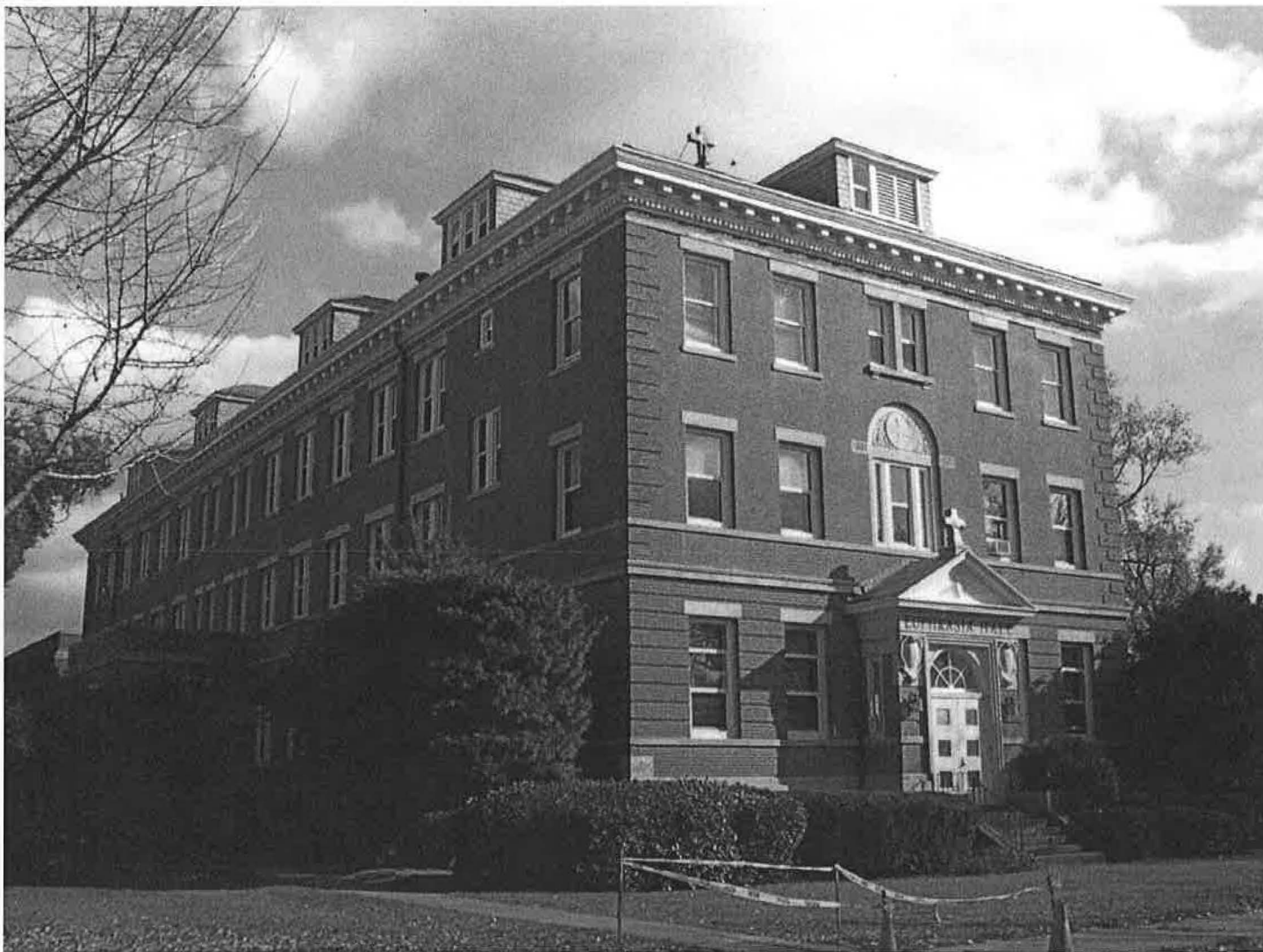
West (front) and north (side) elevations of 170 Sisson Avenue, 1905, showing façade, roof, entry, and window details.
