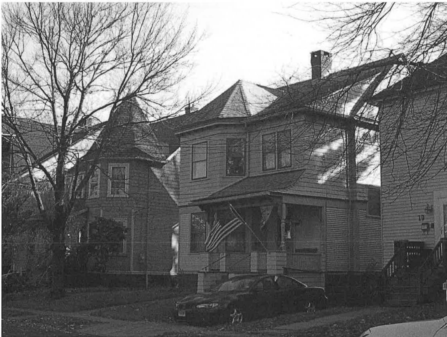
North (front) and west (side) elevations of 15 and 17 Warrenton Avenue, 1898 and 1905, showing façade, roof, porch, and window details. Camera facing southeast. Photograph 9 of 37.
