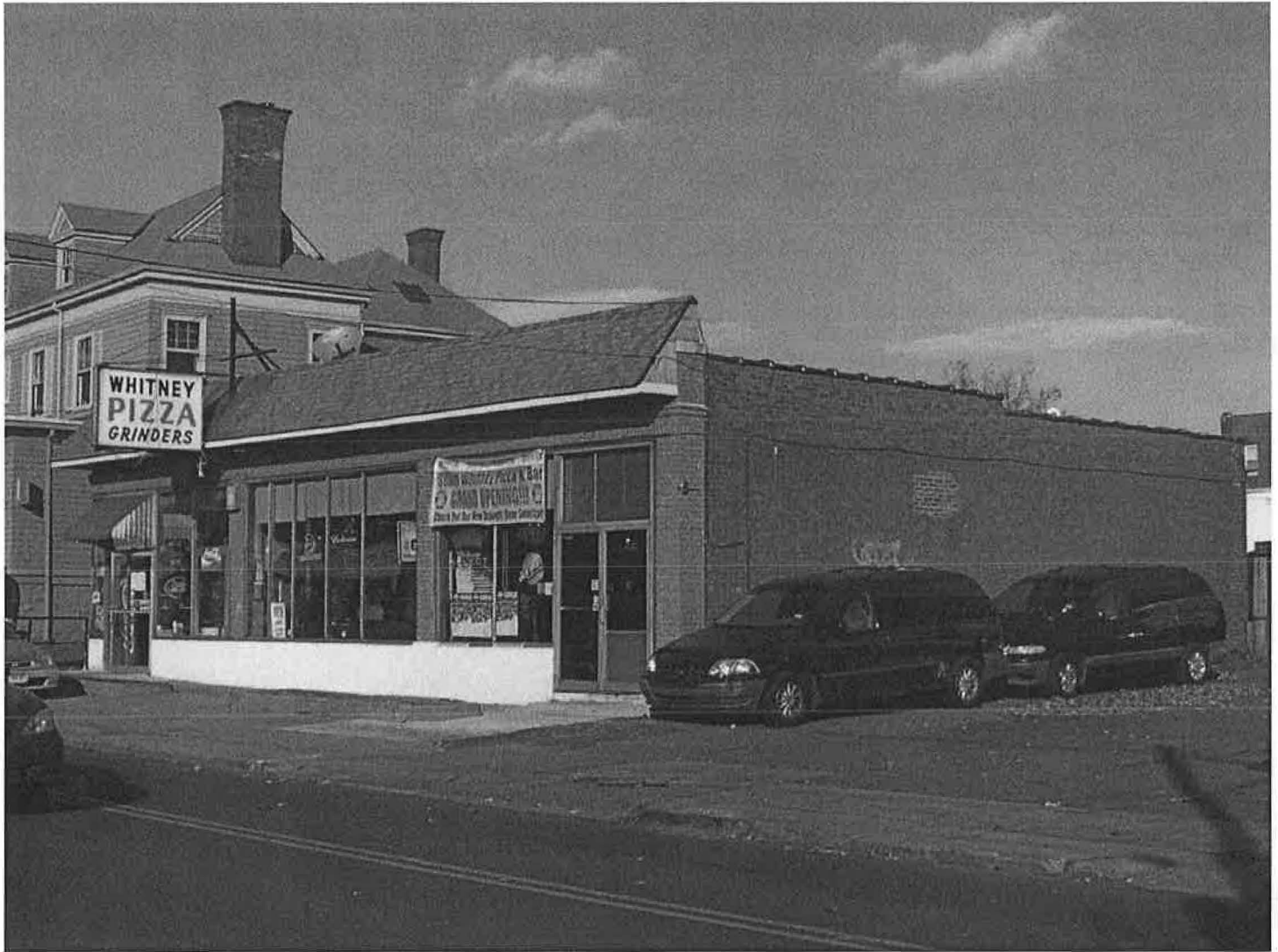
West (front) and south (side) elevations of 262-264 South Whitney Street, 1926, showing façade, roof, porch, and window details.
