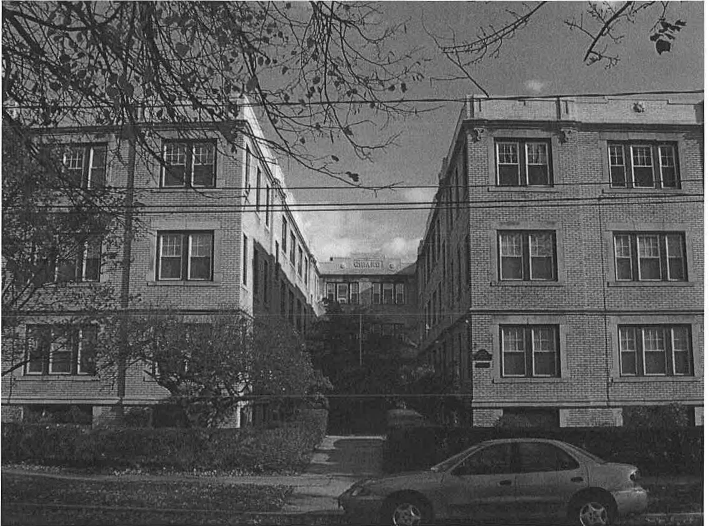
West (front) elevation of 16-26 Girard Avenue, 1920, showing façade, roof, entry, and window details. Camera facing east. Photograph 25 of 37.
