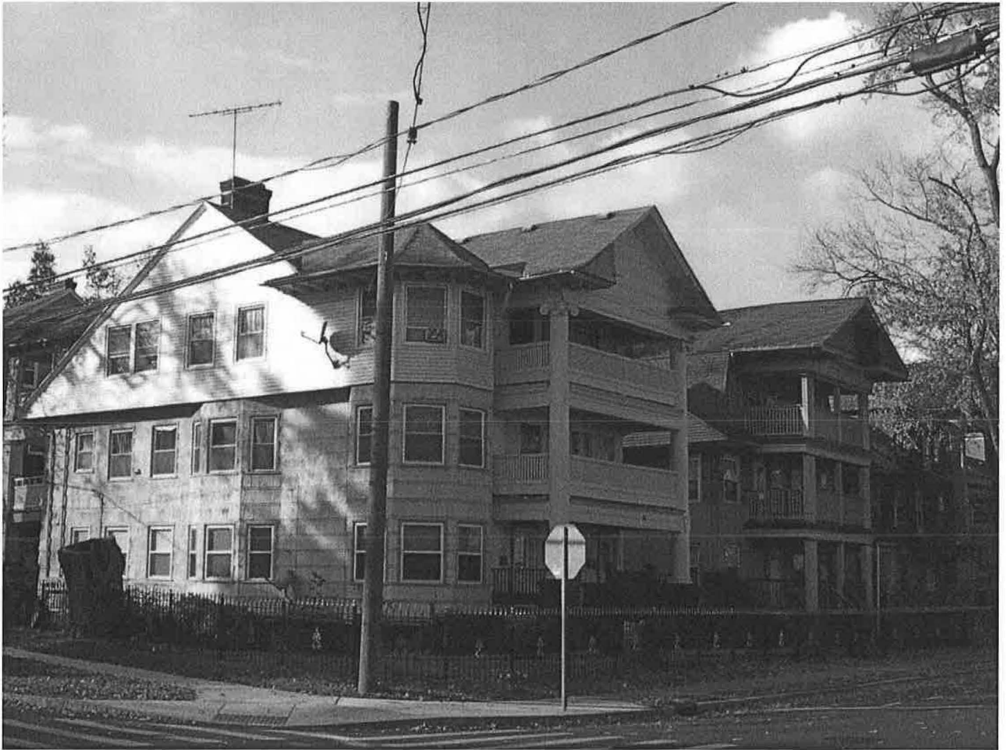
East (front) and south (side) elevations of 183-185 and 187-187 South Whitney Street, 1914, showing façade, roof, porch, and window details. Camera facing northwest. Photograph 17 of 37.
