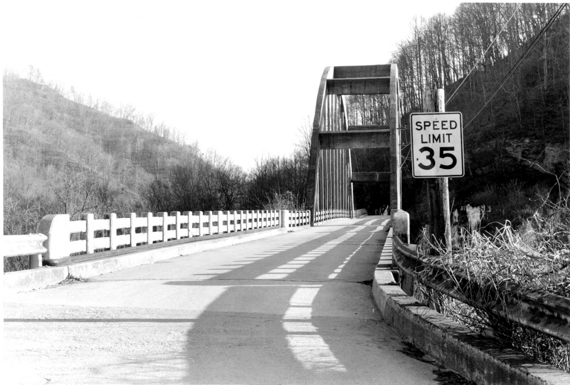
Town Branch Bridge Prestonsburg MS Floyd Co., KY
