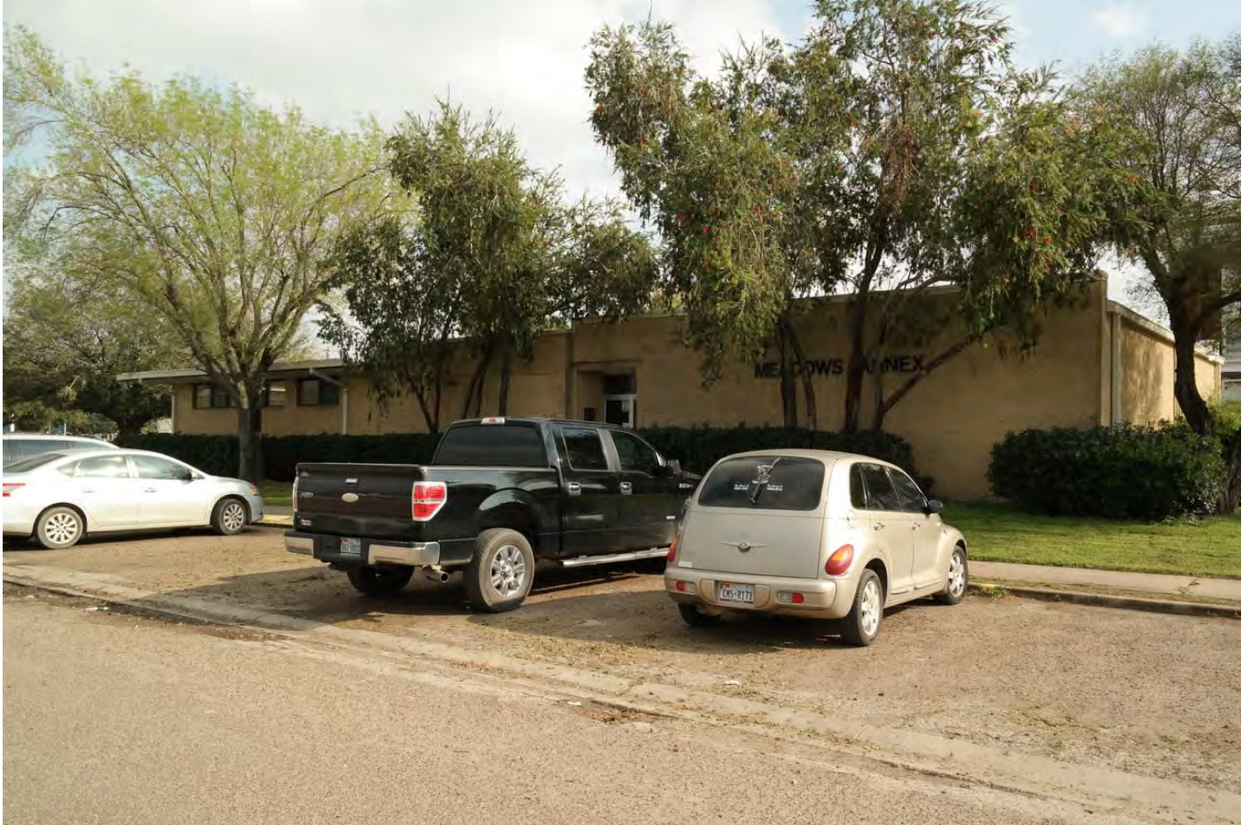
Photo 13 1950 Willacy County Library (contributing), north elevation
