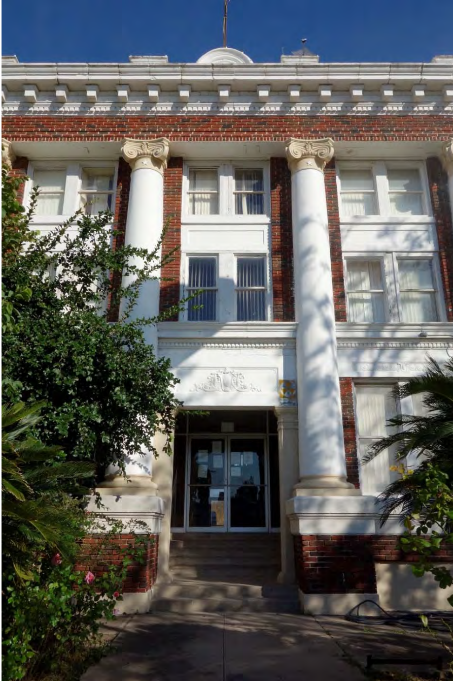
Photo 2: South Elevation, entry detail
