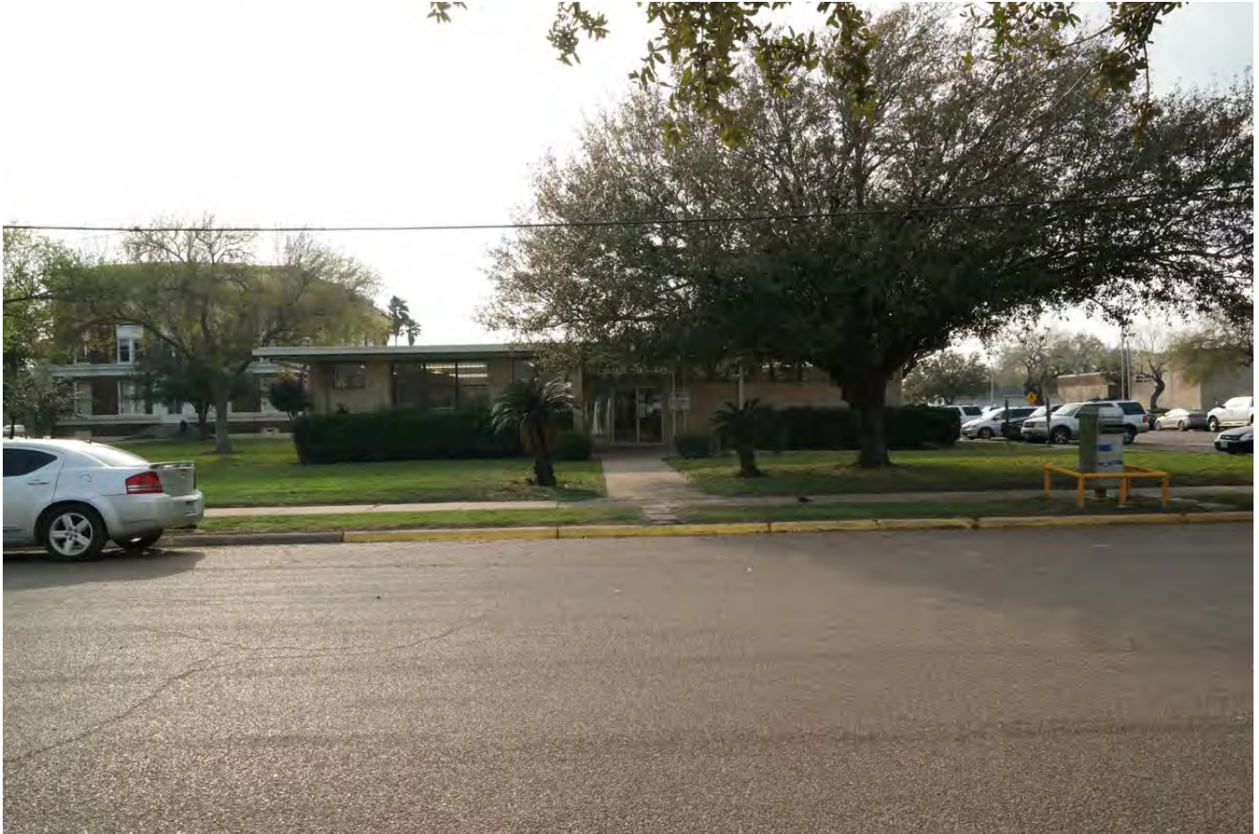
Photo 14 1950 Willacy County Library (contributing), east elevation
