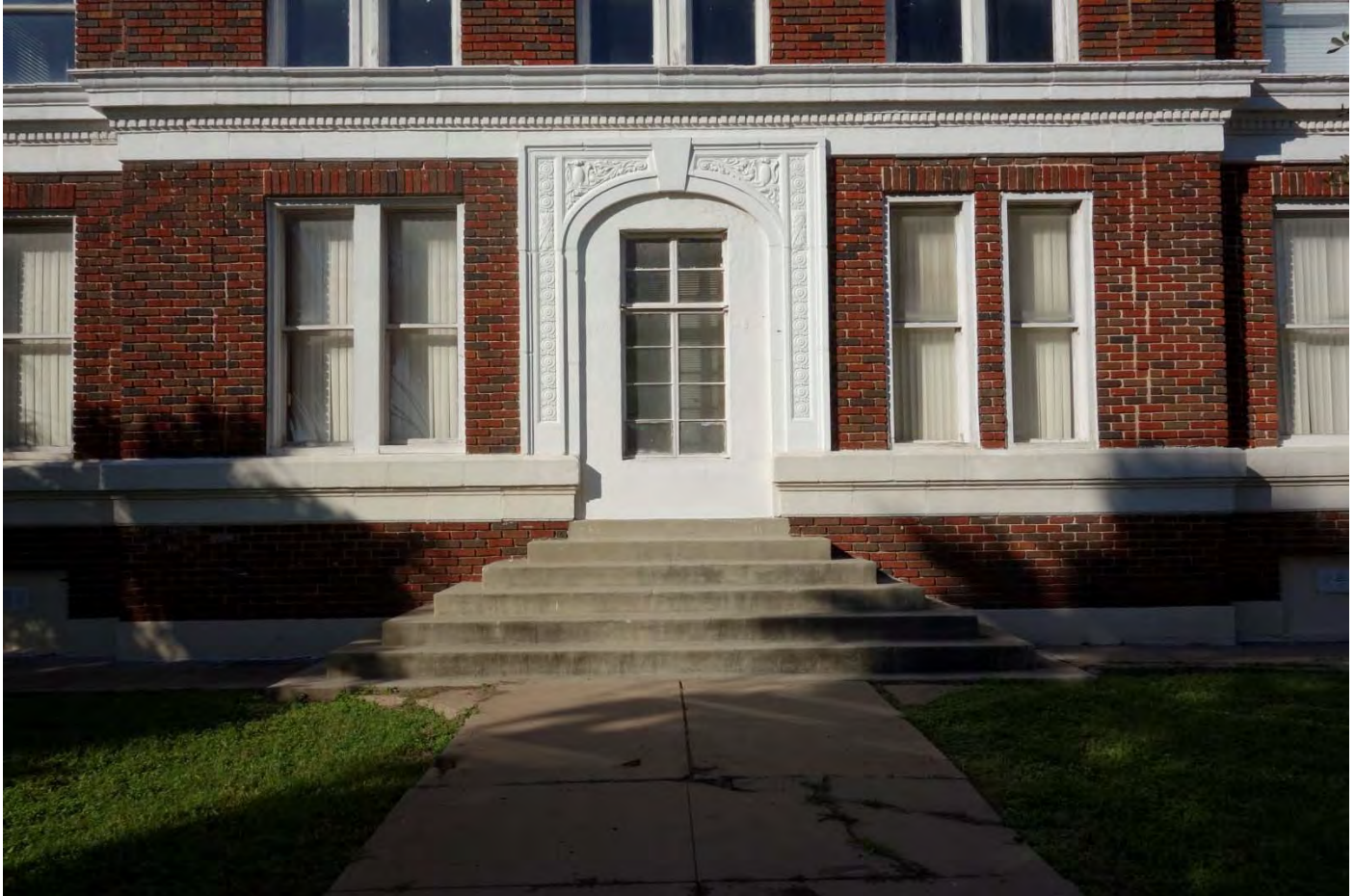
Photo 4: East Elevation, entry detail
