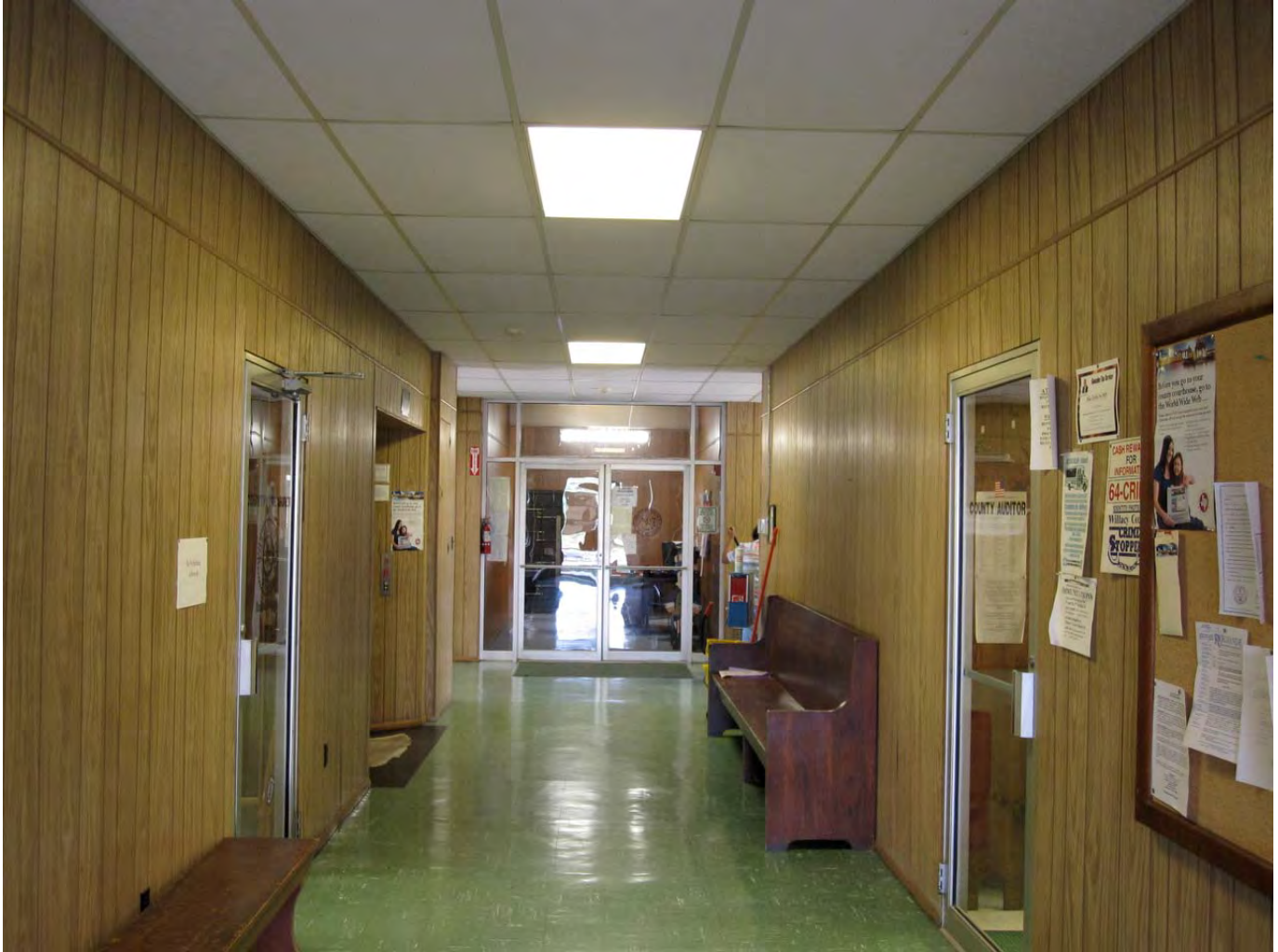
Photo 9: First floor corridor
