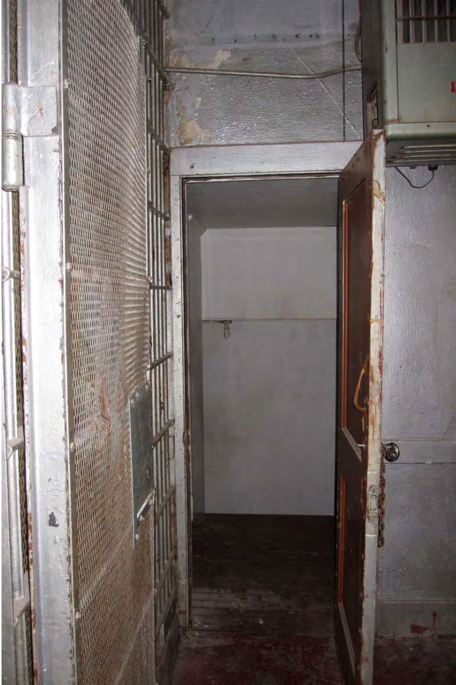
Photo 11: Third floor corridor
