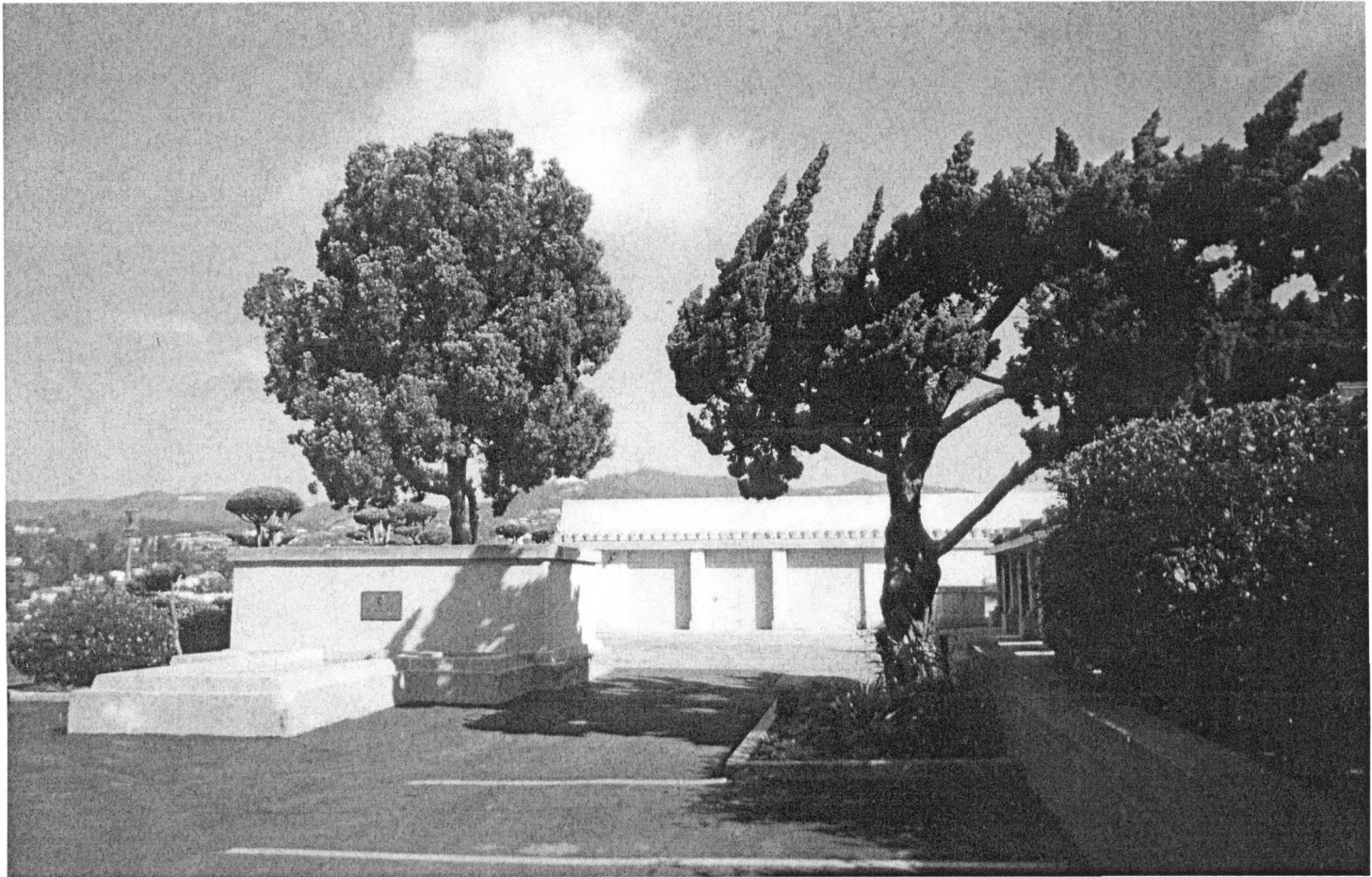
Exterior view, motor court and garage, looking north. Thomas Koester, photographer, 15 Mar. 2006.
