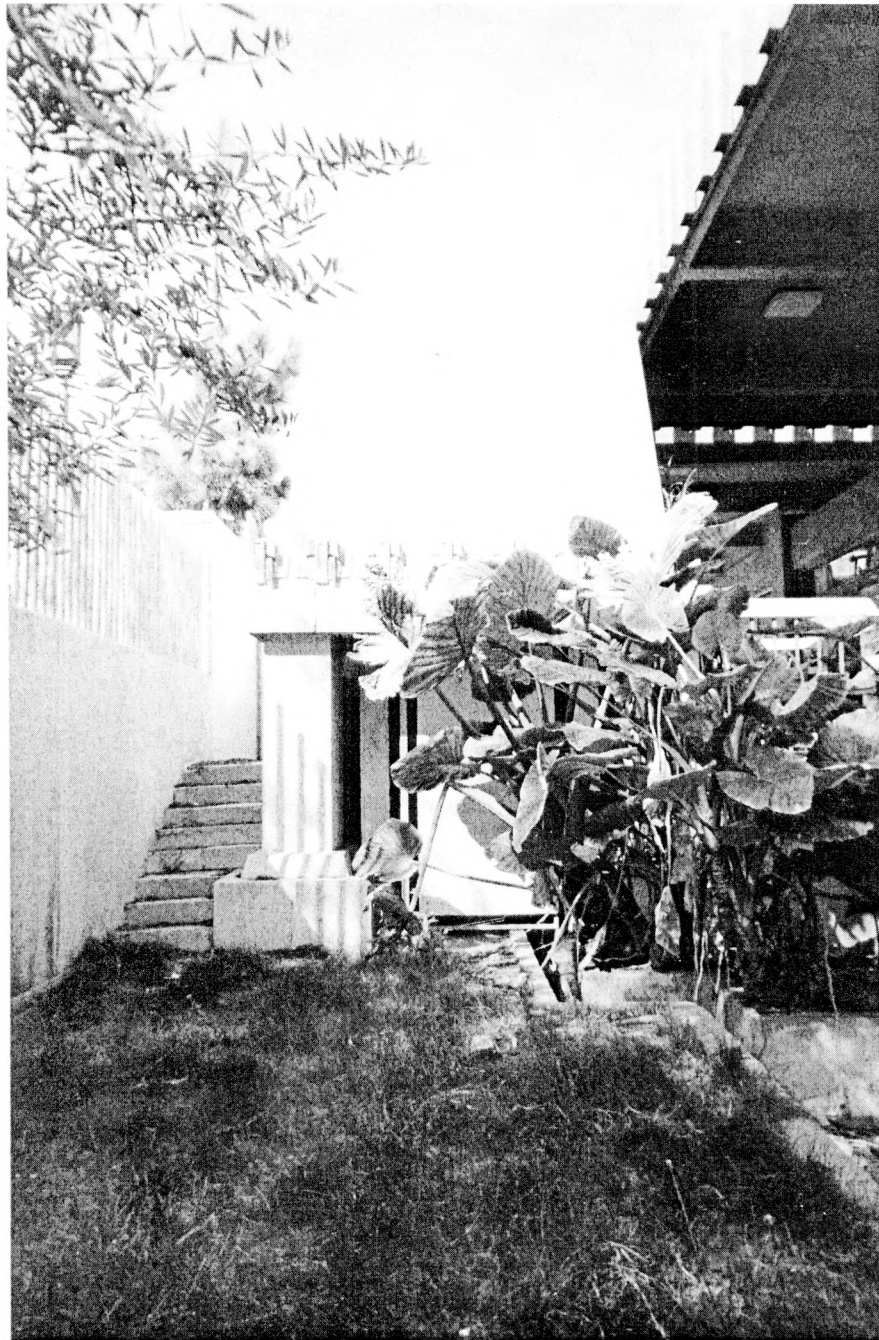
Spring house, south elevation. Thomas Koester, photographer, 15 Mar. 2006.
