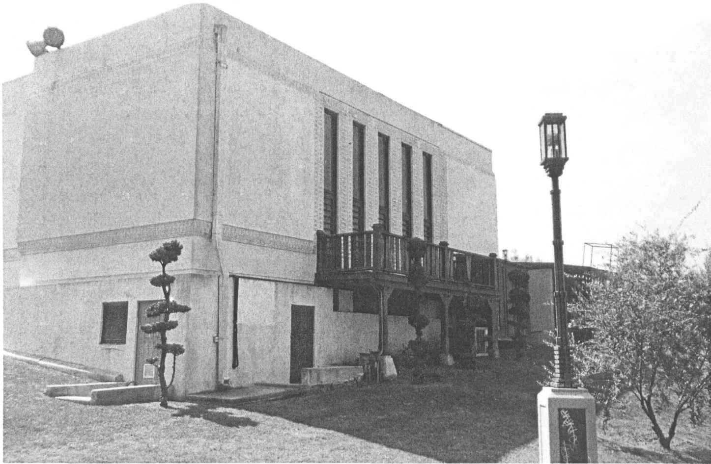
Residence "A", exterior view, looking southwest. Thomas Koester, photographer, 15 Mar. 2006.
