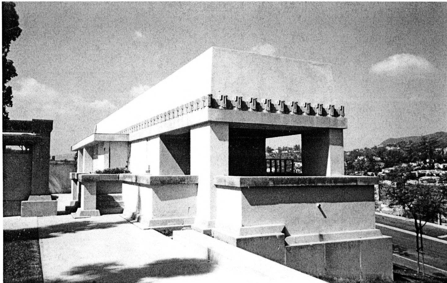
Exterior view, garage, looking northwest. Thomas Koester, photographer, 15 Mar. 2006.
