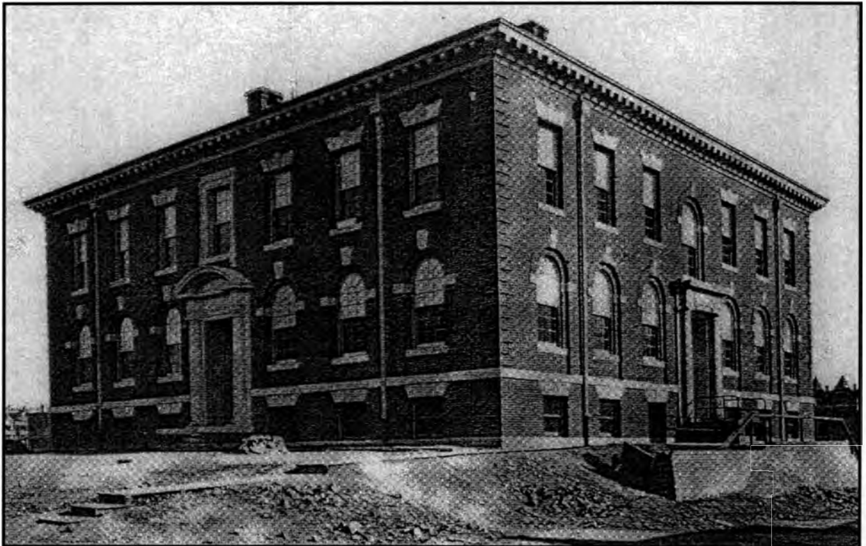
1904 View of Nathaniel Parker Gage School (From D.C. Historic Preservation Office Vertical Files, Gage School)
