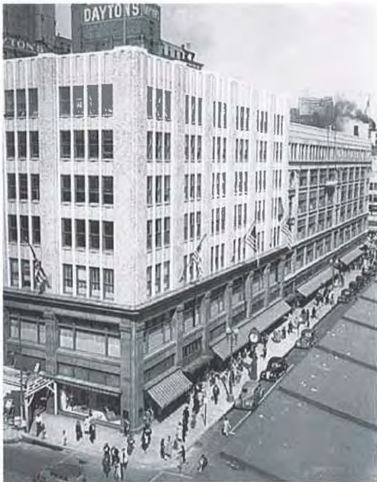
Figure R. Dayton's Department Store, 1937. Photo courtesy of the Minnesota Historical Society.
