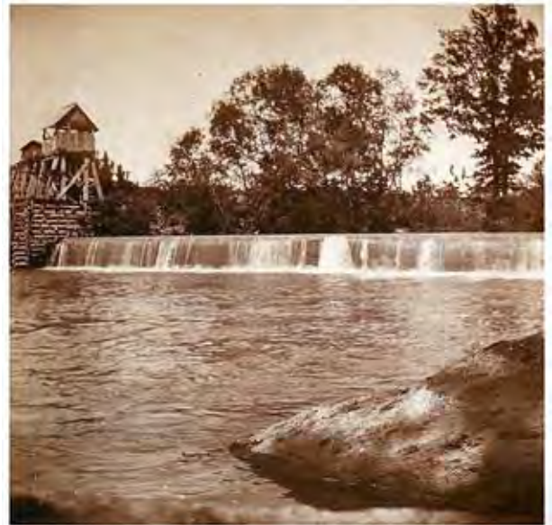
Ca. 1950 photo of the dam for the Hardison Mill along the Duck River
