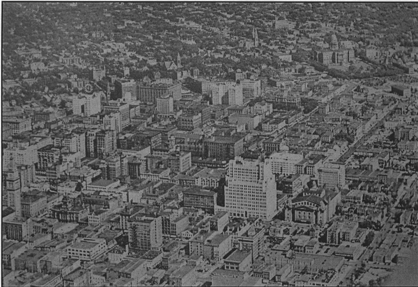
Figure 6. The height, mass, light buff color, and stepped design of the Telephone Building (lower center) made it a landmark on the Downtown Denver skyline. SOURCE: The Monitor , September 1929, 28.
