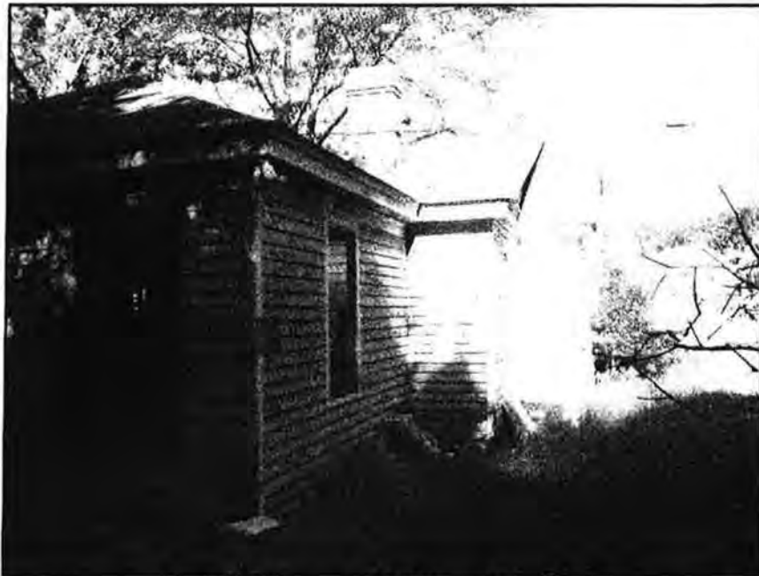
Figure 14: Plummer T. Hall House, facing West.
