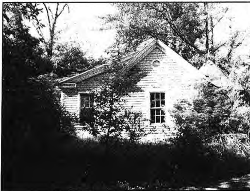
Figure 13: Plummer T. Hall House, facing South.
