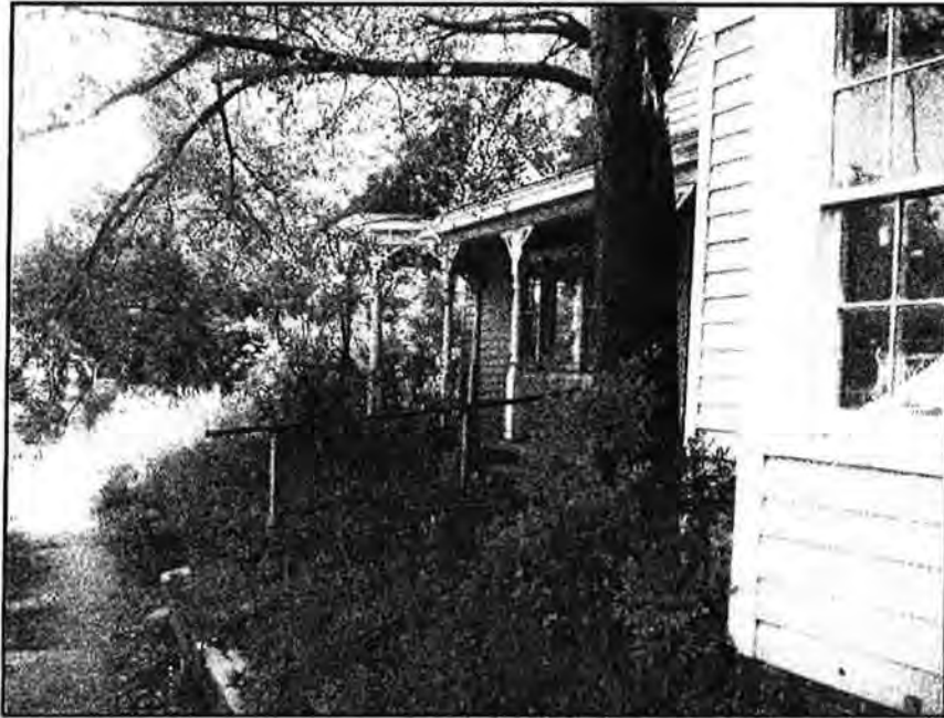
Figure 16: Front of Plummer T. Hall House, facing North-Northeast.
