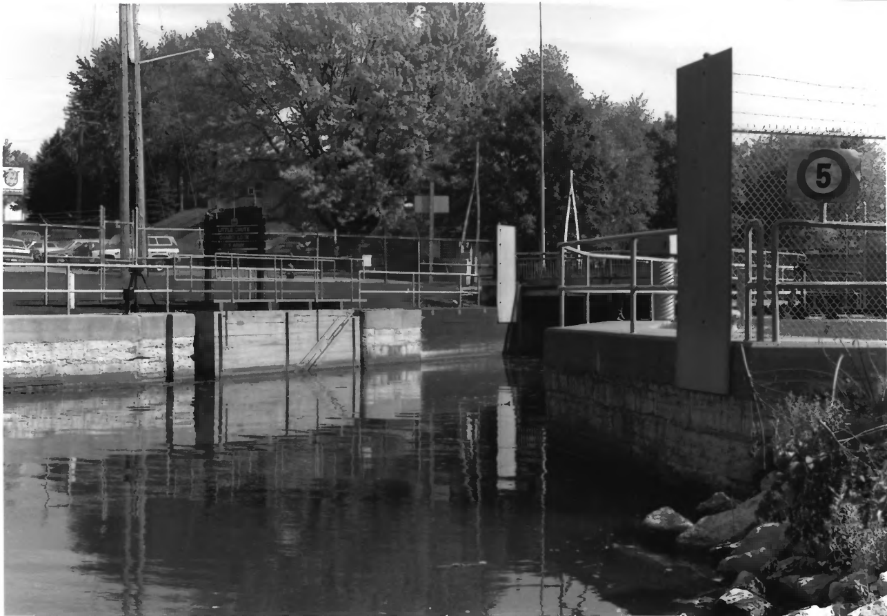
Little Chute Locks Hist Dist, Little Chute, Outagamie County, Photo # 2 of 10
