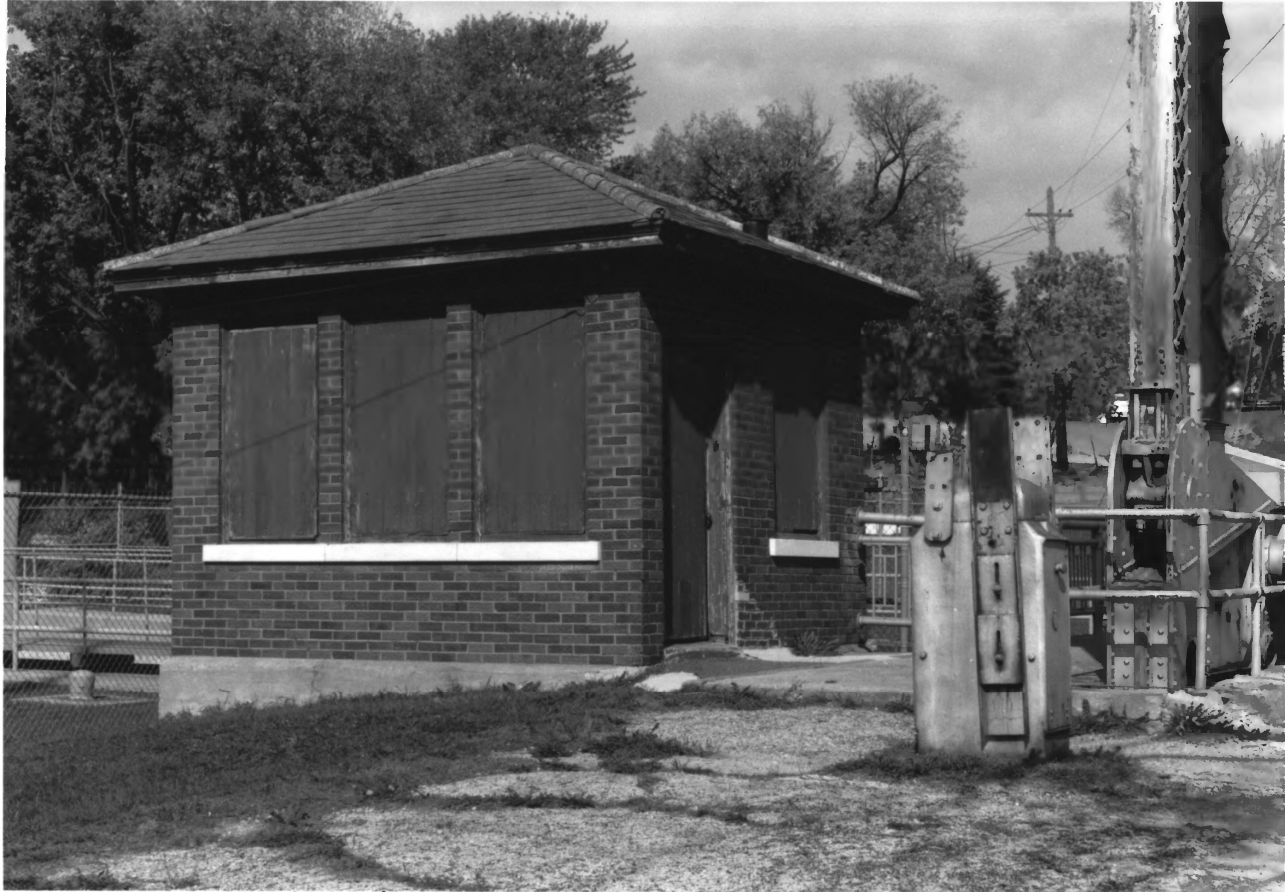
Little Chute Locks Hist Dist, Little Chute, Ooutasawrie County, Photo # 3 of 10
