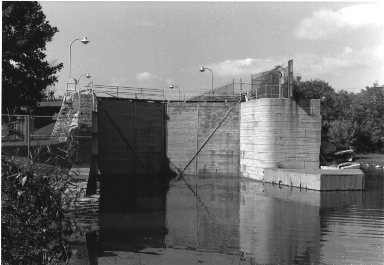
Little Chute Locks Hist Dist, Little Chute, Outagamie County, Photo #6 of 10
