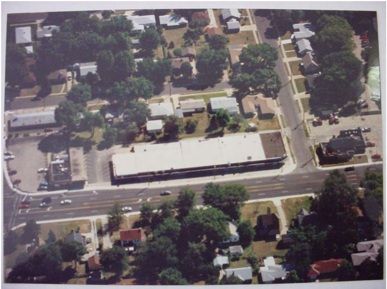
Aerial view after the 1993 road widening. (Left is north)
