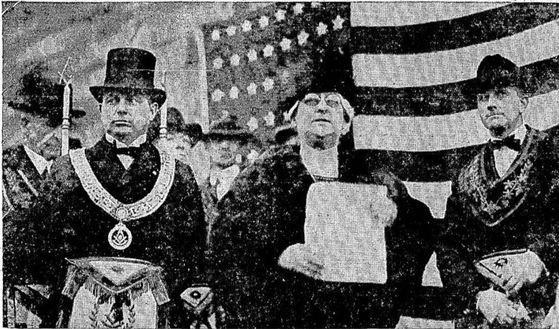
CORNERSTONE OF D. A. R. HOME IS LAID —Members of Rainier Chapter, Daughters of the American Revolution, witnessed the fulfillment of their dream to erect a chapter home in Seattle when the cornerstone of their memorial home at Harvard Avenue and Roy Street was laid yesterday. The ceremony of putting the stone in place was conducted by the Grand Lodge of Washington, Free and Accepted Masons, in the presence of officers and members of the chapter and their friends. A copper box containing records of the chapter and newspaper articles on the construction of the memorial was placed in the stone before it was set in place by Robert C. McCroskey, most worshipful master of the grand lodge. The address of the day was delivered by Mrs. David W. Bowen, regent of Rainier Chapter. In this photograph, left to right, are Mr. McCroskey, Mrs. Bowen and Walter F. Meier, senior grand warden. (See news columns.)
