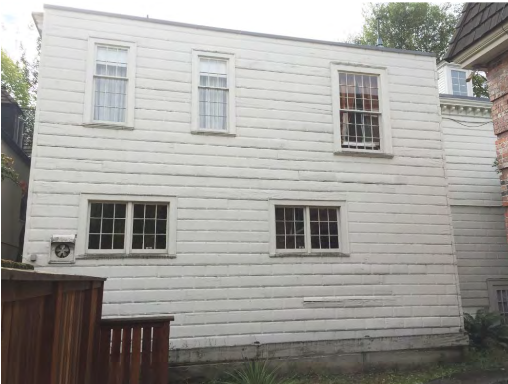
7 of 20 – Rear / North Façade Northeast corner showing kitchen extension (1927).
