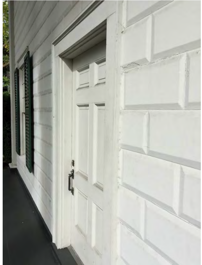
5 of 20 – Detail of entry door and siding.
