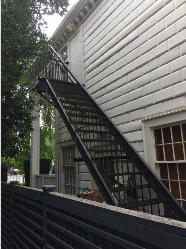
6 of 20 – West façade showing second floor fire escape.
