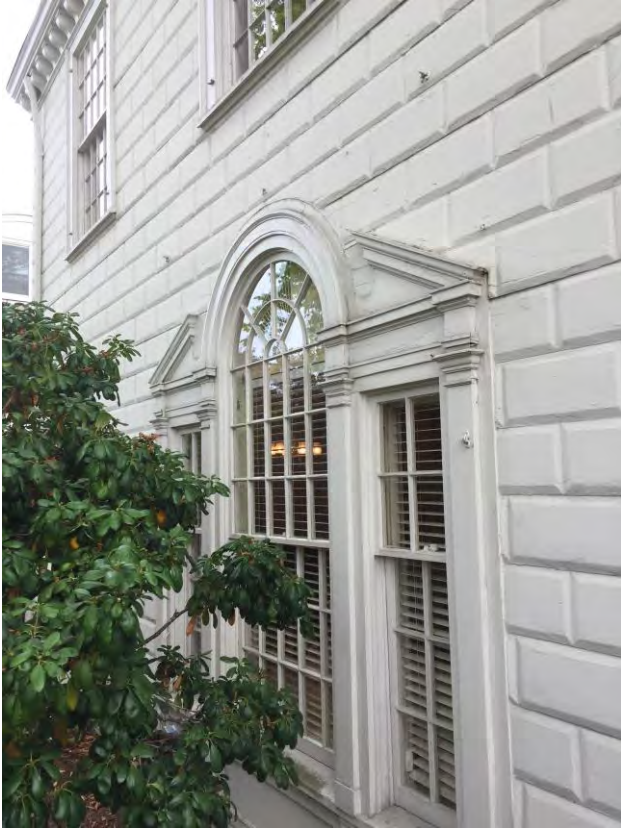
8 of 20 – Detail of Palladian style window on West elevation.
