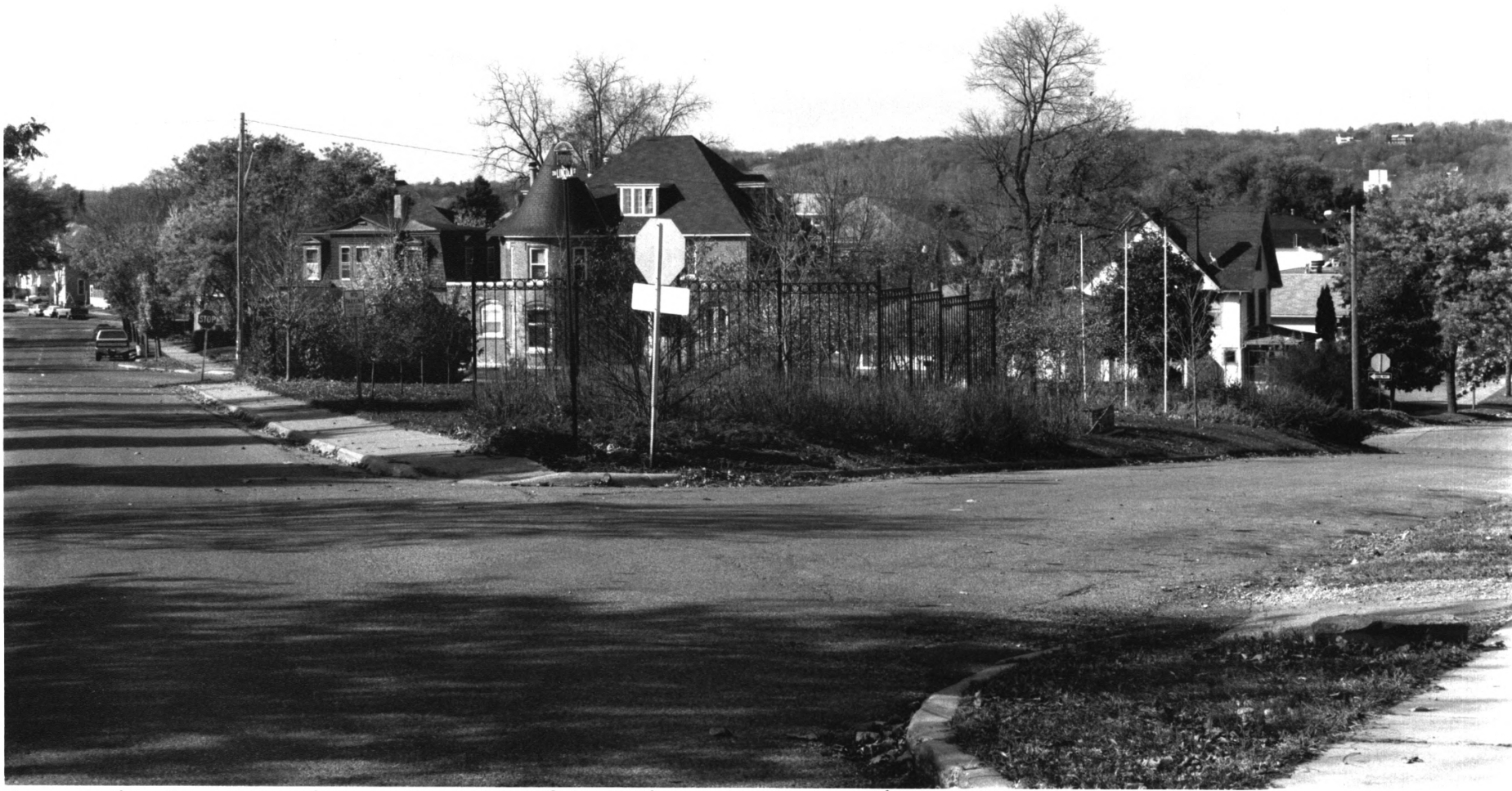
Street Scape Lincoln St. 200 Block, Lincoln Park Lincoln Park Residential Historic District Blue Earth Co., mn 011773-3
