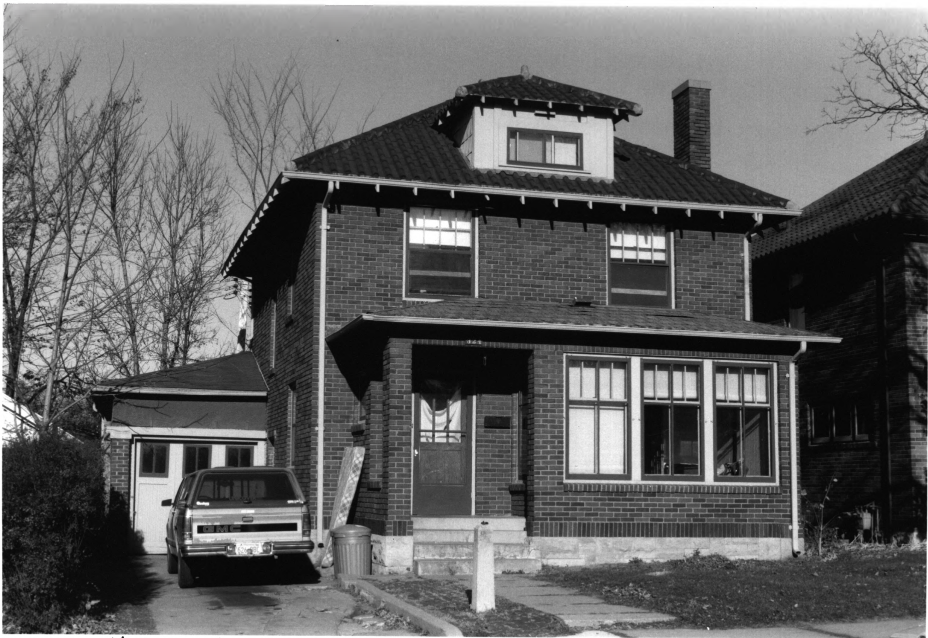
Gendler House, #128 Lincoln Park Residential Historic District Blue Earth Co., MN 011787-9
