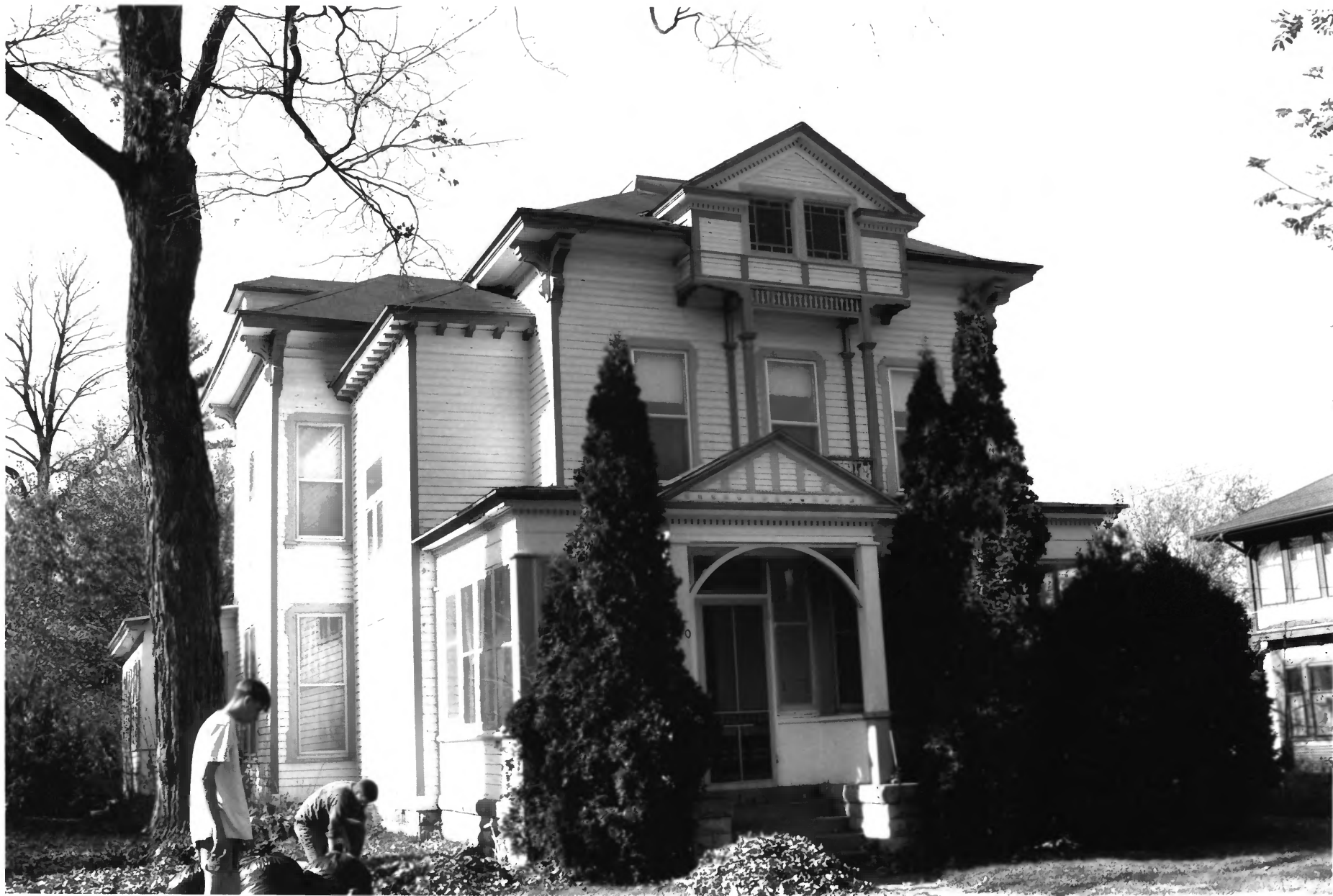
Noe House, #85 Lincoln Park Residential Historic District Blue Earth Co., MN 011777-19
