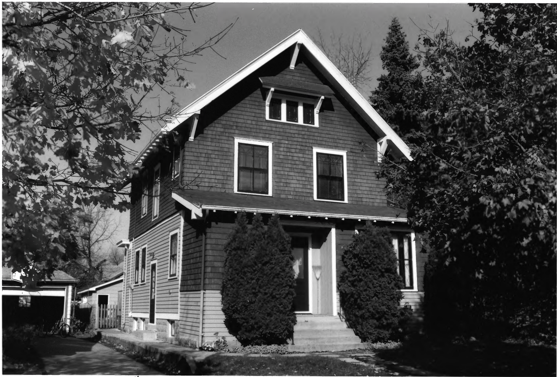
McGovern House, #192 Lincoln Park Residential Historic District Blue Earth Co., MN 011768-16
