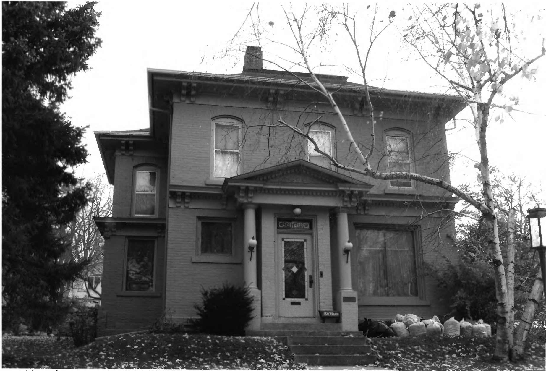
Little House, # 132 Lincoln Park Residential Historic District Blue Earth Co., MN 011770-15
