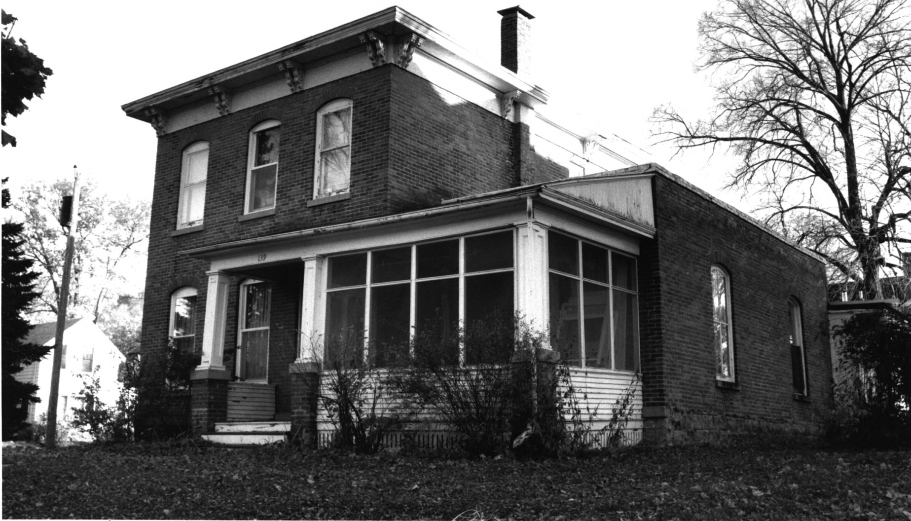
Durkee/Veigel House, #181 Lincoln Park Residential Historic District Blue Earth Co., MN 011793-15
