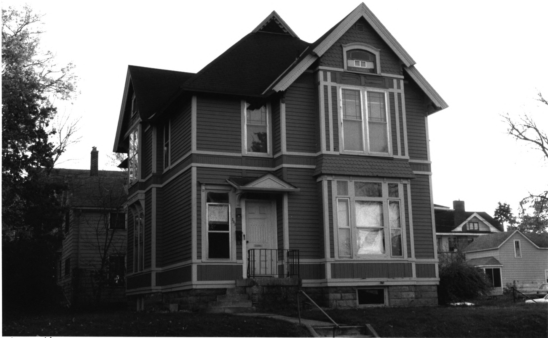
Hart House, #182 Lincoln Park Residential Historic District Blue Earth Co., MN 011760-14
