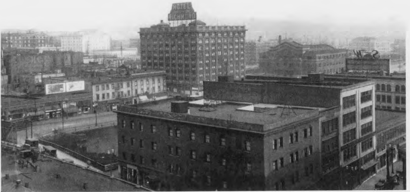
New Richmond Hotel in background (center) – 1932 Photo courtesy of University of Washington Special Collections
