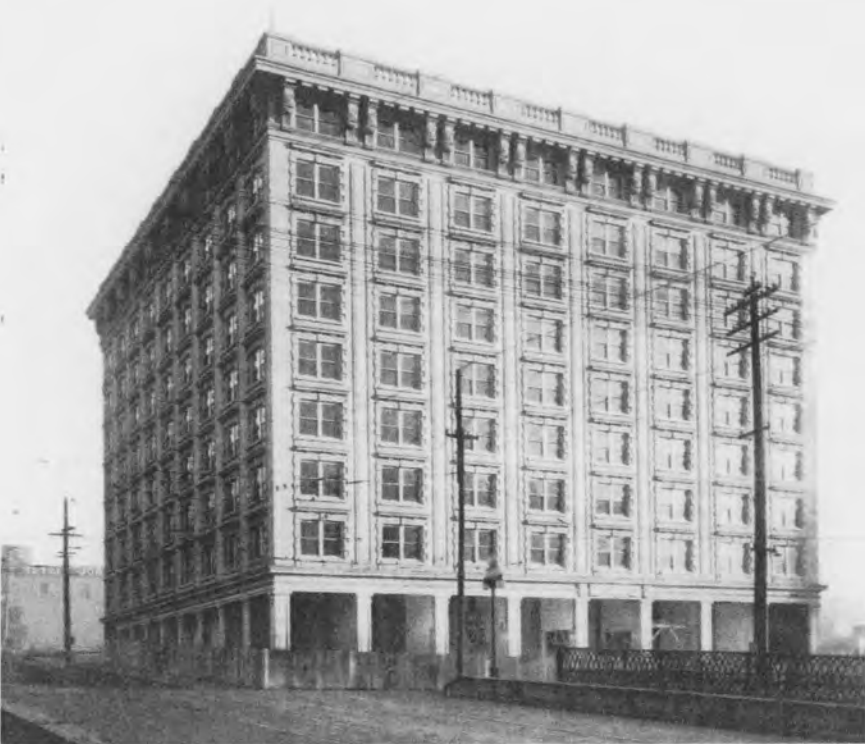
New Richmond Hotel under construction (note missing storefronts) – 1910
