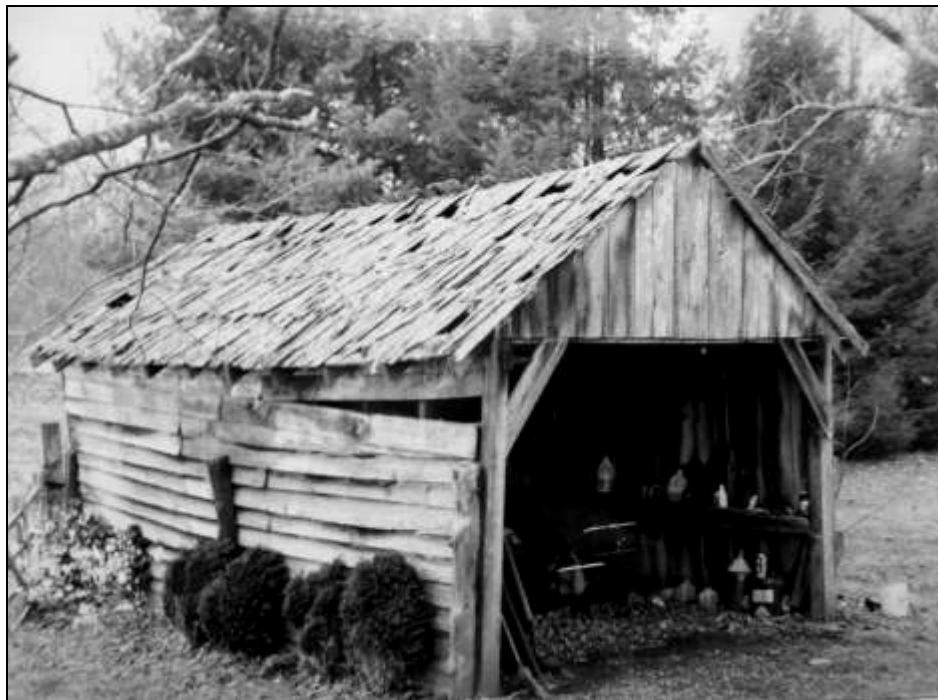
10. Early Twentieth-Century Garage Formerly Located In West Side Yard. Source: Susan Bull Ryan.
