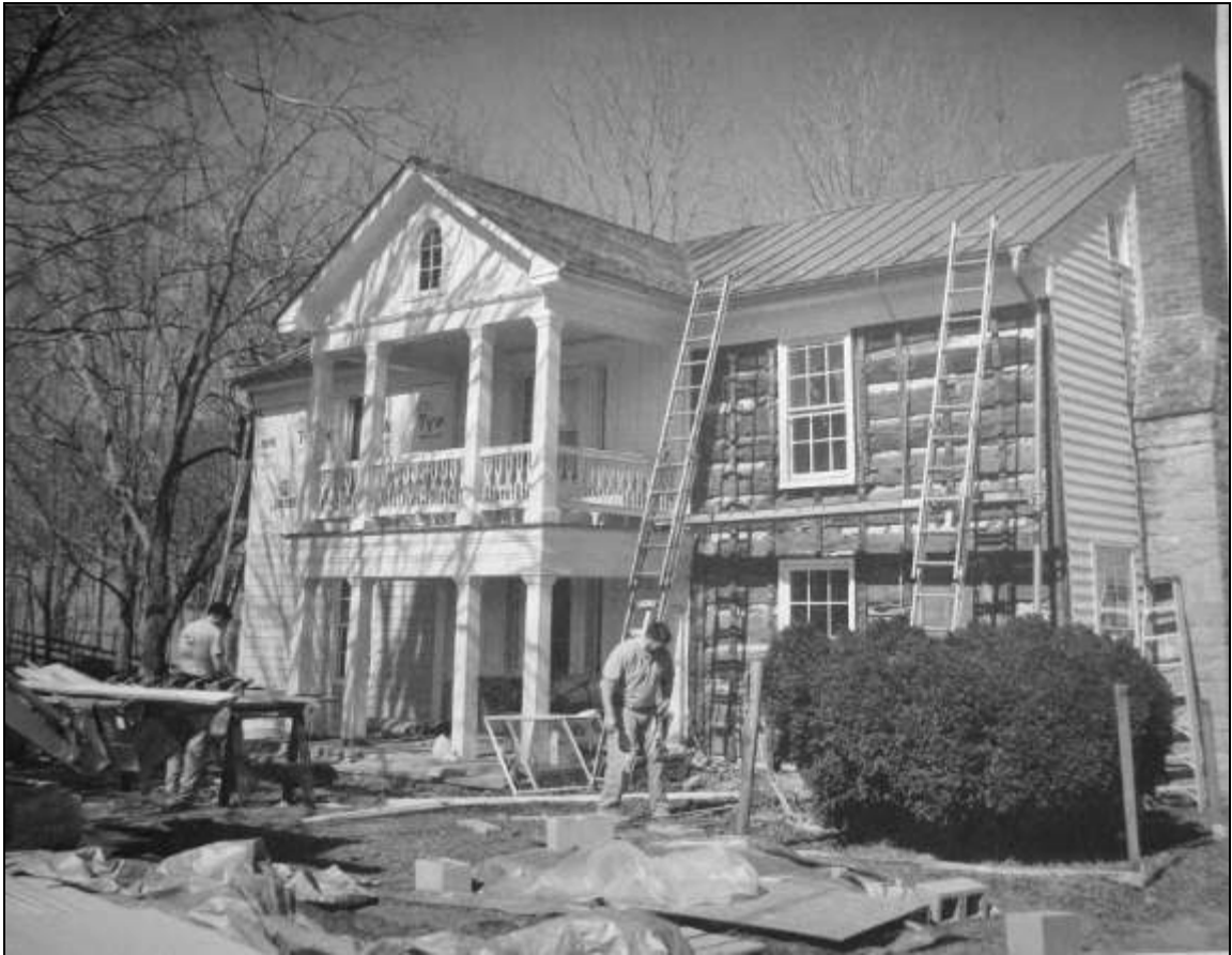
11. Slusser-Ryan House during Renovation Showing Log Construction of East Wing, Prior to 2011. Source: Susan Bull Ryan.
