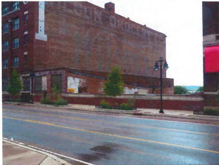
808 SW Washington (left) and now demolished 810 SW Washington (right).
