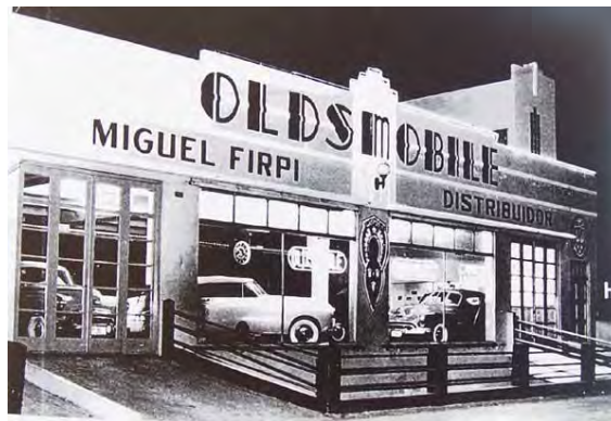
Figure 66. Oldsmobile Showroom, 1925, Puerta de Tierra Historic District, San Juan de Puerto Rico. 297
