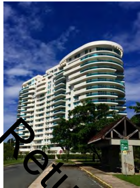
Figure 84. Condominio Millennium, Puerta de Tierra, San Juan de Puerto Rico, 1990s, Google, Public domain.
