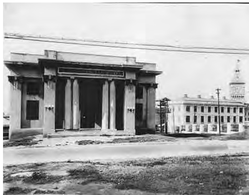
Figure 68. Masonic Lodge (destroyed), Puerta de Tierra Historic District, San Juan de Puerto Rico by Antonin Nechodoma, 1920s. 304
