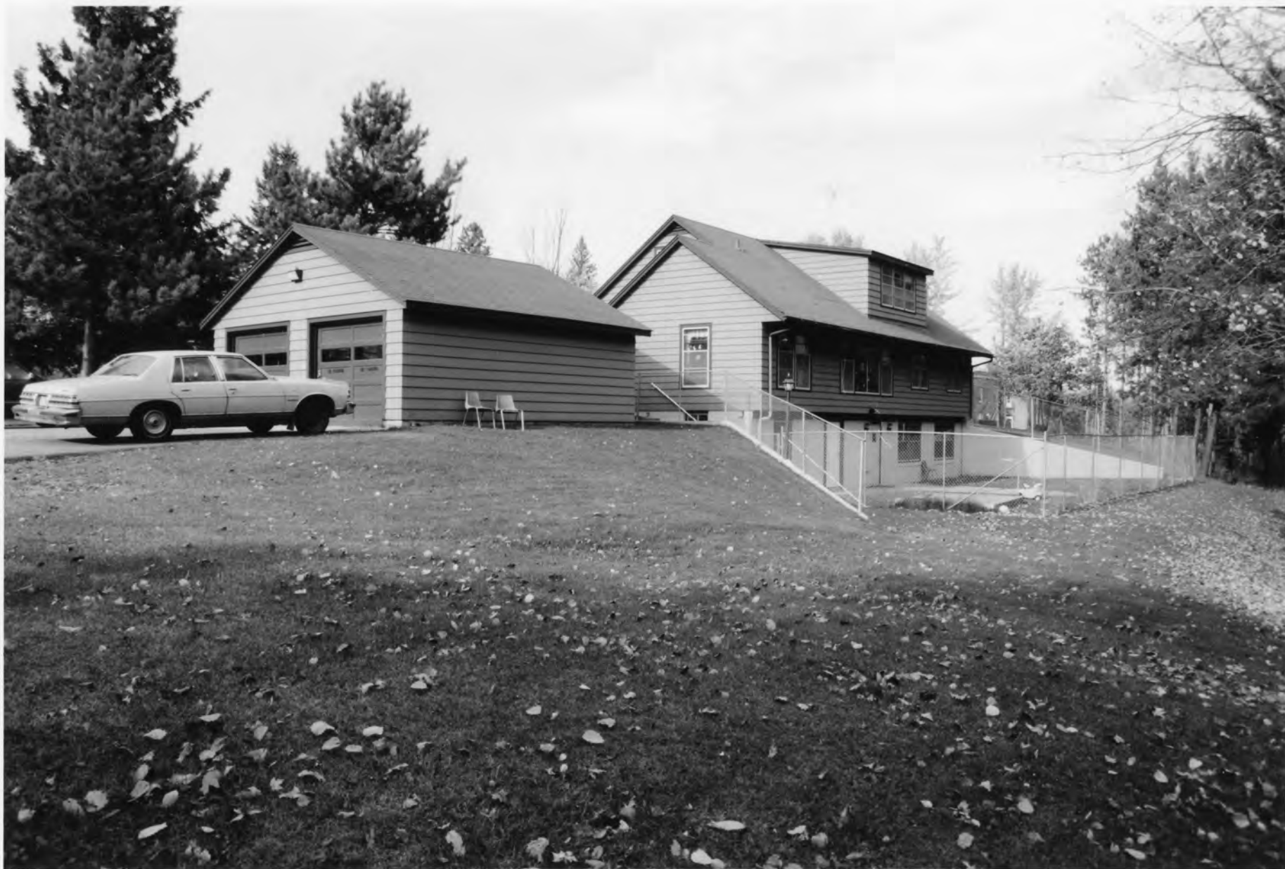
MINNESOTA STATE SANATORIUM FOR CONSUMPTIVES #19 SUPERINTENDENT'S RESIDENCE (NC) CASS CO., MN 012666-19
