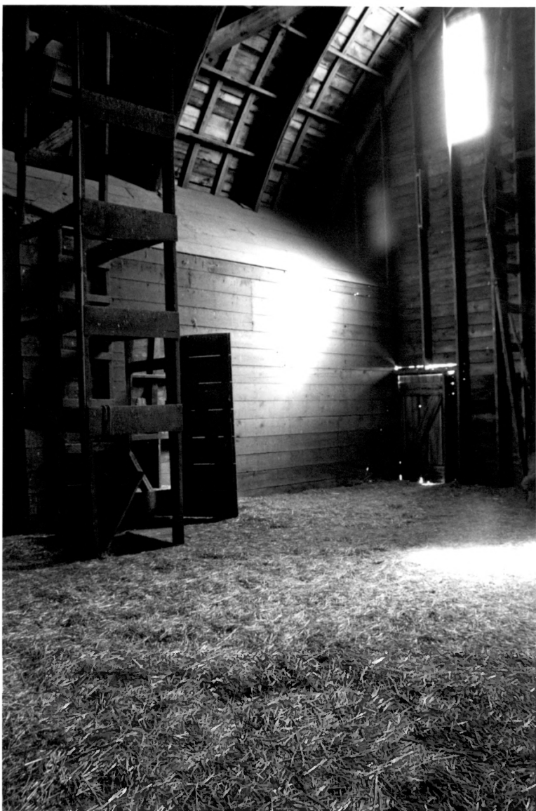
Herman F. Michael Gothic Arched-Roof Barn, Brookings Co., S. D., No. 3
