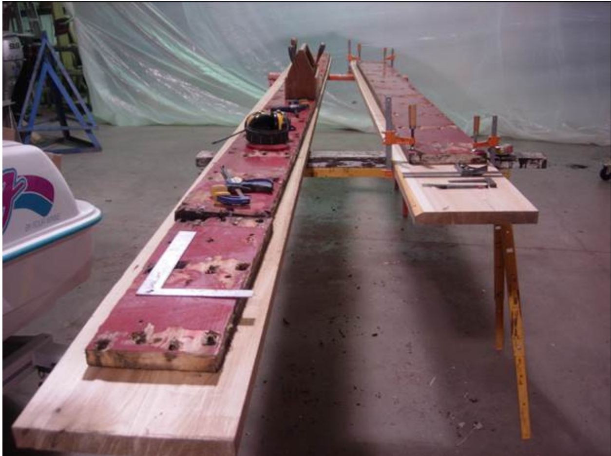
MT_GlacierCounty_Rising Wolf_0009, planking, showing restoration process.
