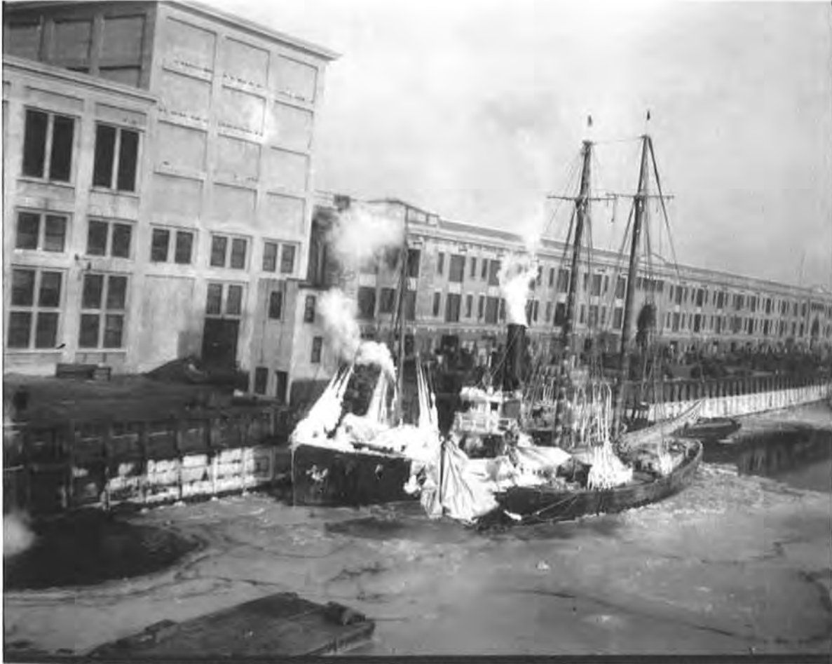
Figure 10. “Fish Pier in Winter,” Leslie Jones, ca. 1950. Boston Fish Pier East Building at right, cold storage building (no longer extant) at left (Boston Public Library, Leslie Jones Collection).
