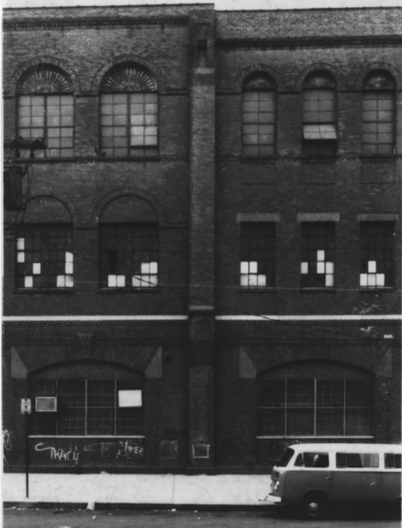
North side of PAVONIA Avenue, opposite
