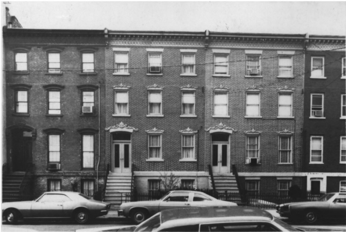
211 213 215 North side of Pavonia, opposite, between GROVE AND ERIE Streets
