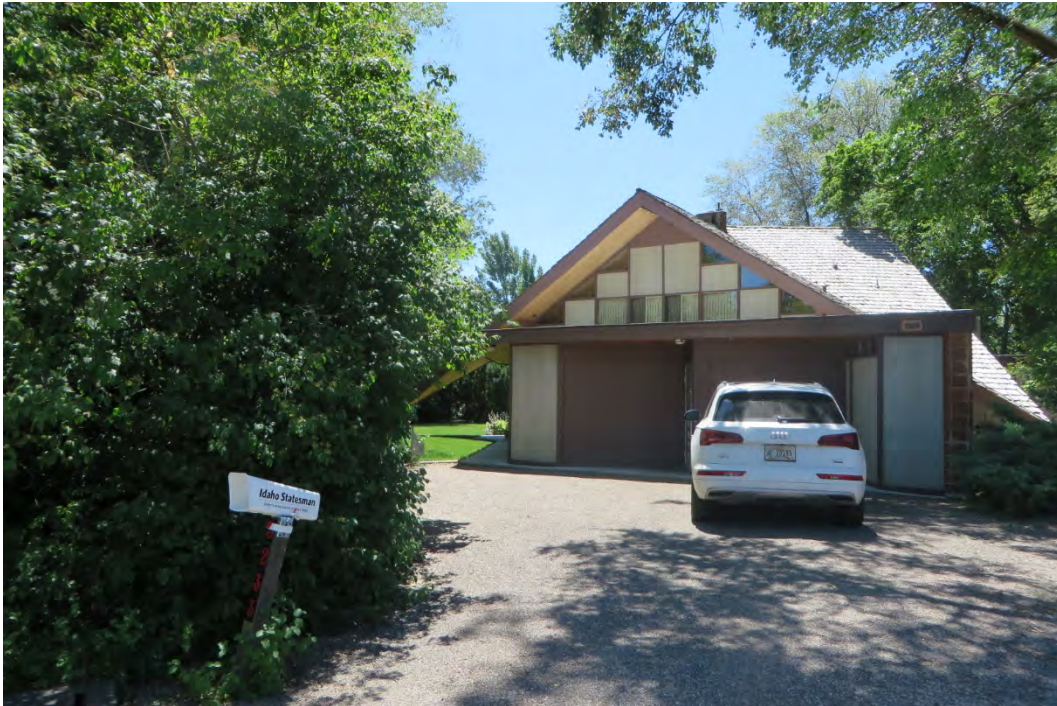
Photo 1 Phillips House, looking southwest, from driveway entrance on Edson Street.
