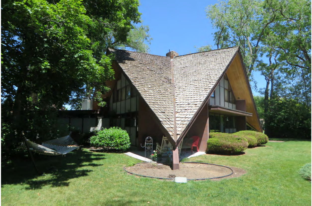
Photo 11 Dynamic Roof Structure with concrete footing, South Elevation with overhang, Northwest Elevation, partially obstructed Shop Addition, looking northeast.
