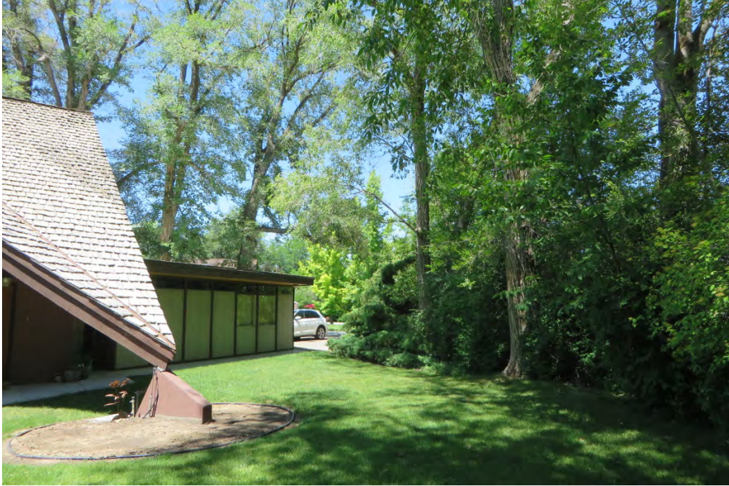
Photo 7 Accessory Dwelling Unit, partially visible main entrance, mature tree line along eastern property boundary, driveway to Edson Street, looking north/northeast.
