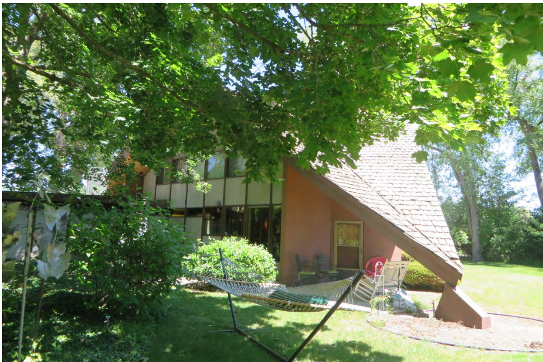
Photo 12 Northwest Elevation, partially obstructed Shop Addition, taken from west edge of property line, looking east.
