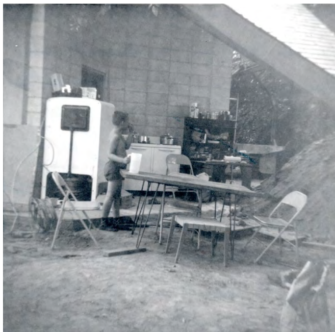
Figure 33 Photograph from 1958 Phillips House Construction c. 1958. 104
