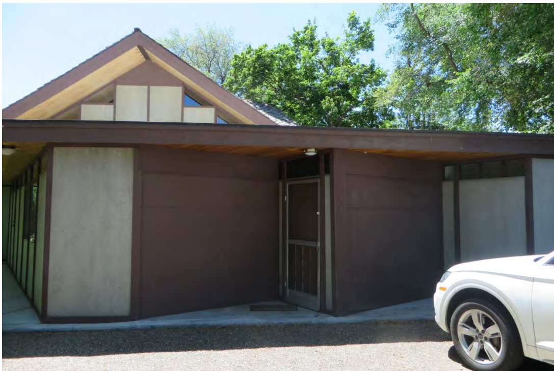
Photo 2 Accessory Dwelling Unit, and partial northeast elevation, looking southwest, from driveway.
