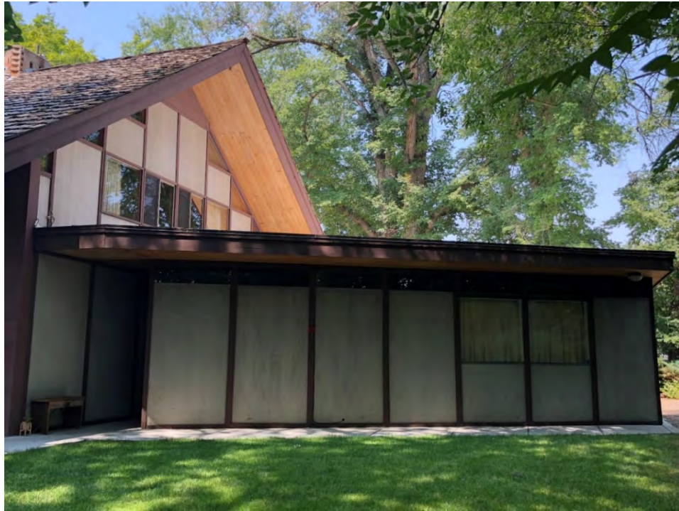
Photo5 Accessory Dwelling Unit, partially obstructed Northeast Elevation, and entrance to breezeway, looking west.
