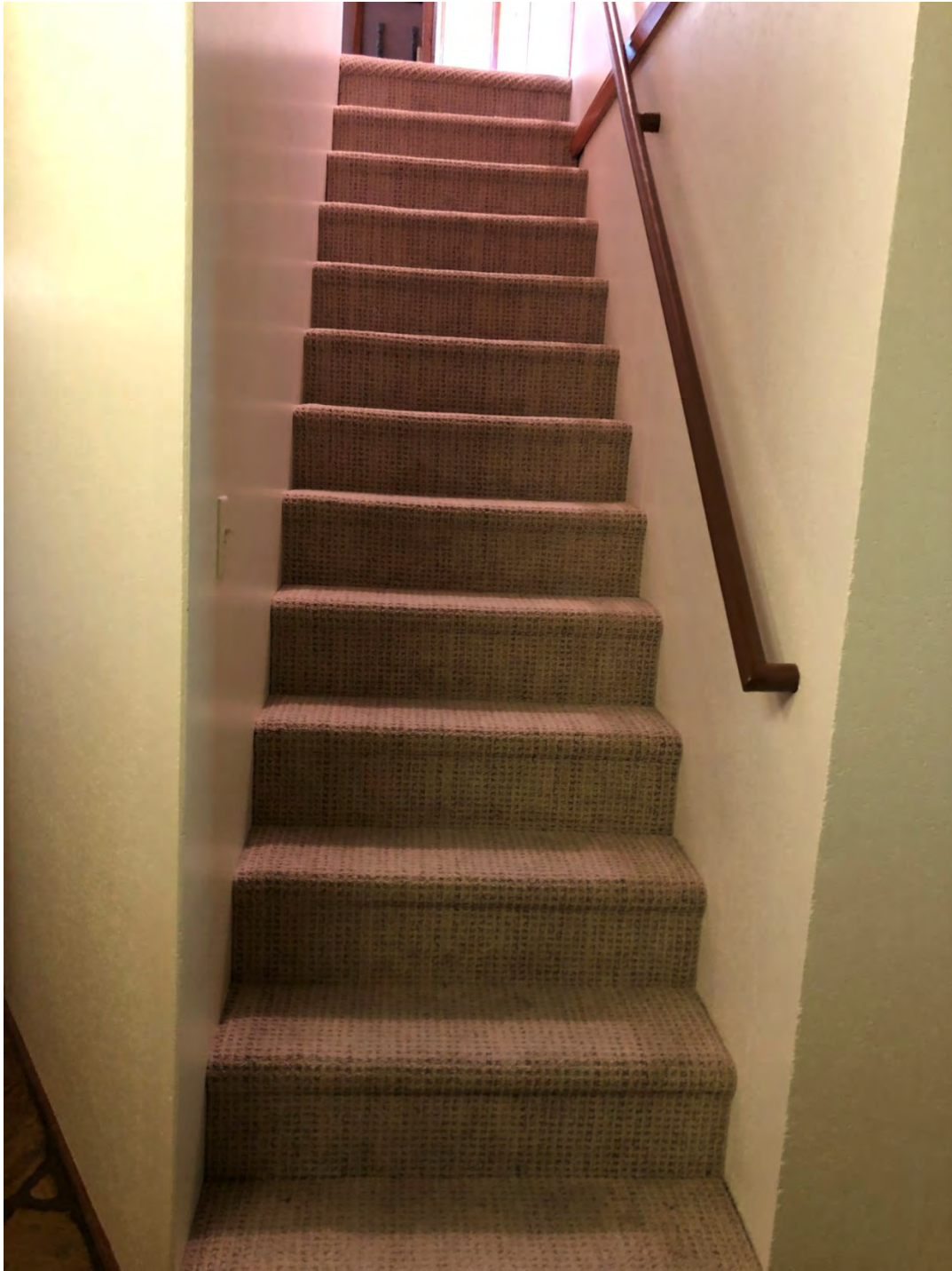
Photo 23 Stairs to second floor, looking southeast..
