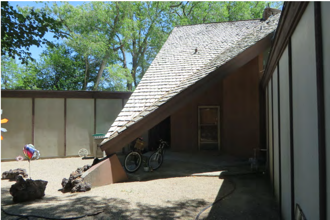
Photo 16 Northeast elevation of Shop Addition (right of frame), entrance to main floor kitchen, Dynamic roof structure and concrete footings, Zen Garden, and northwest elevation of Accessory Dwelling Unit (left of frame).
