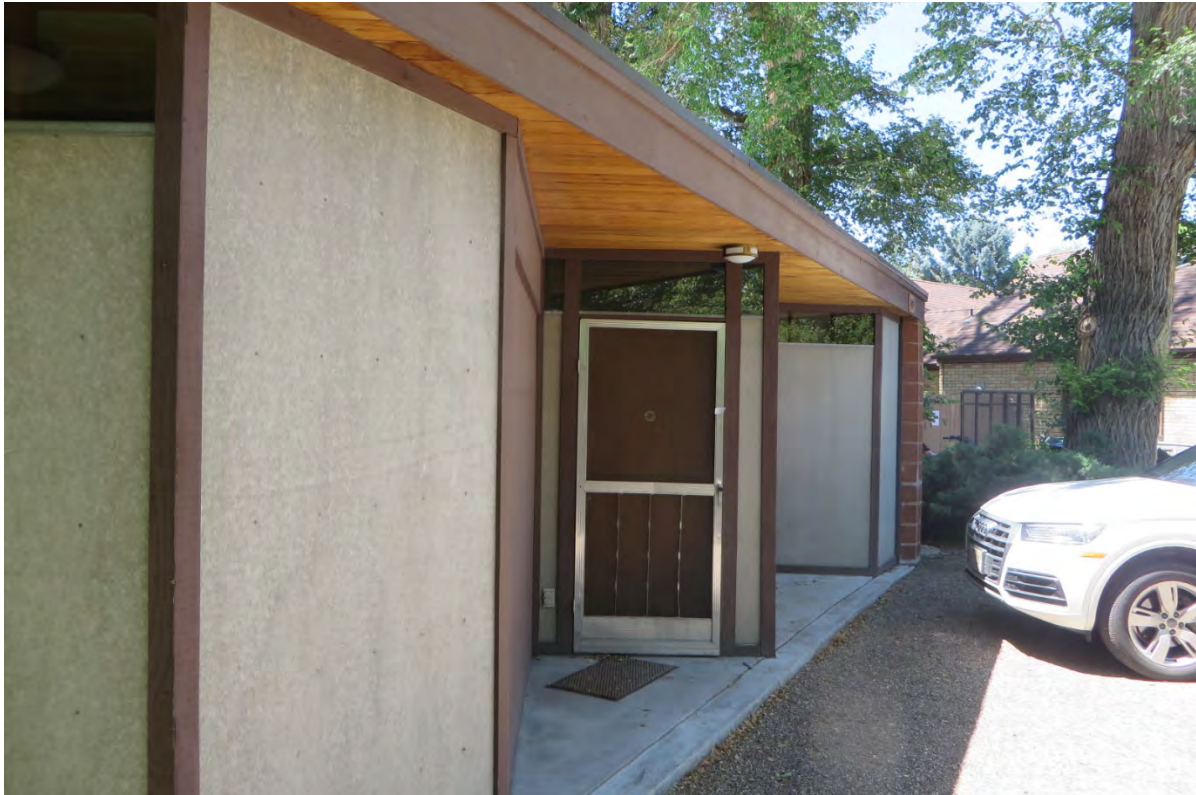
Photo 3 Accessory Dwelling Unit Front Entrance, looking northwest.
