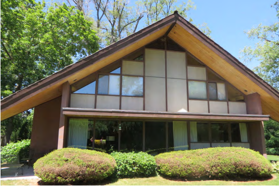
Photo 9 South Elevation, interior living room, and second floor bedrooms, looking north.
