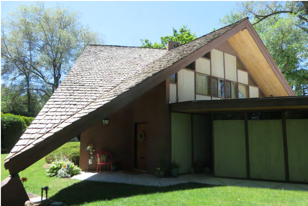
Photo 6 Accessory Dwelling Unit , Northeast Elevation, main entrance, entrance to breezeway. Dynamic roof structure and concrete footings in foreground. Looking southwest.
