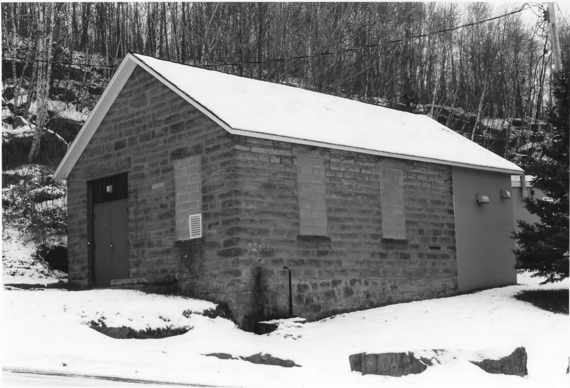
KETTLE RIVER SANDSTONE COMPANY QUARRY - Pumping station PINE CO., MINNESOTA 010681 #1/A
