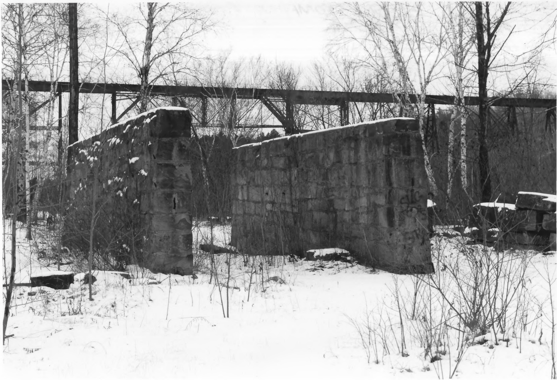
KETTLE RIVER SANDSTONE COMPANY QUARRY, STONE CRUSHER WALLS PINE CO., MINNESOTA 010681 #10/10A
