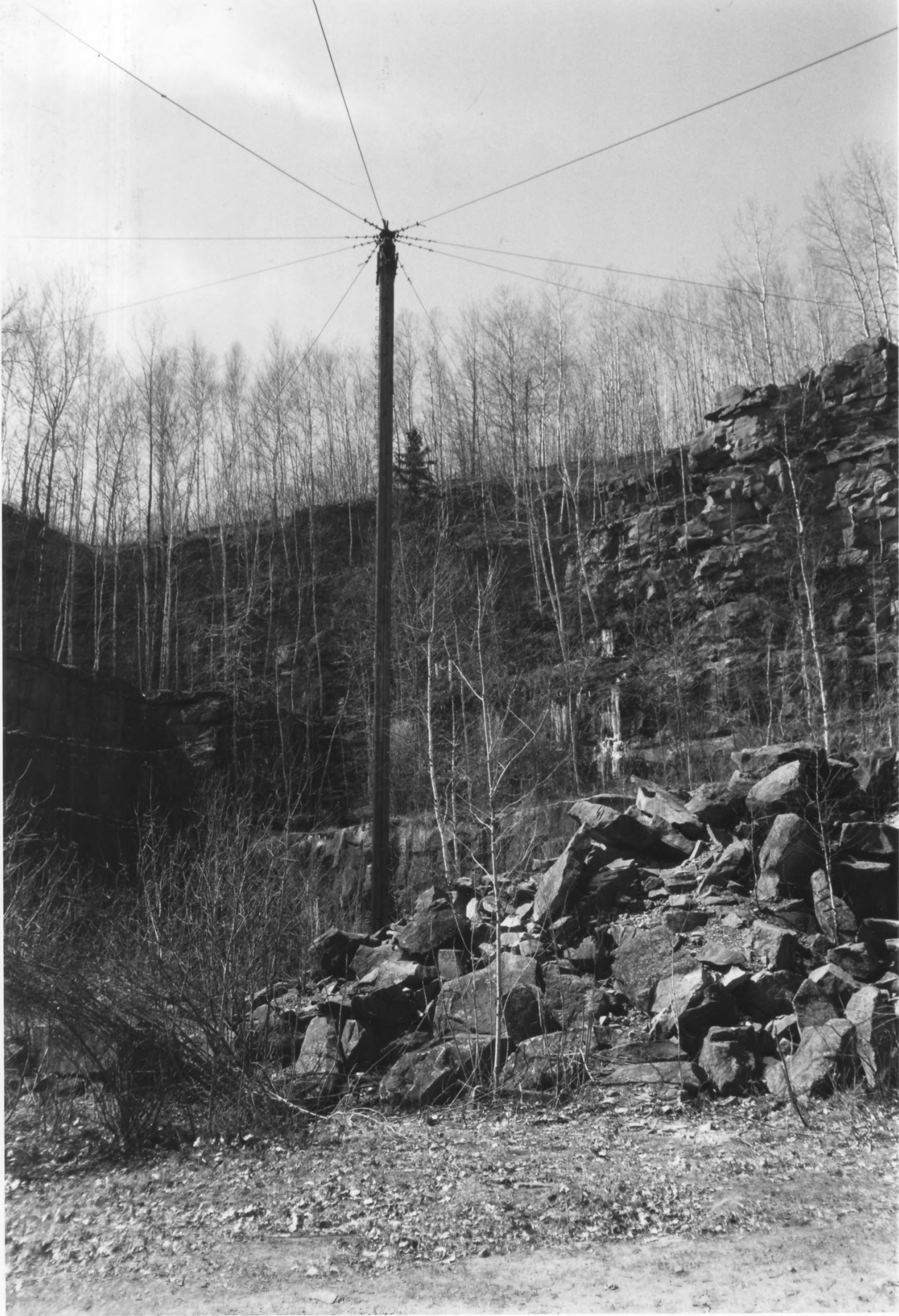
KETTLE RIVER SANDSTONE COMPANY QUARRY, DERRICK MAST PINE CO., MINNESOTA 010544 #19
