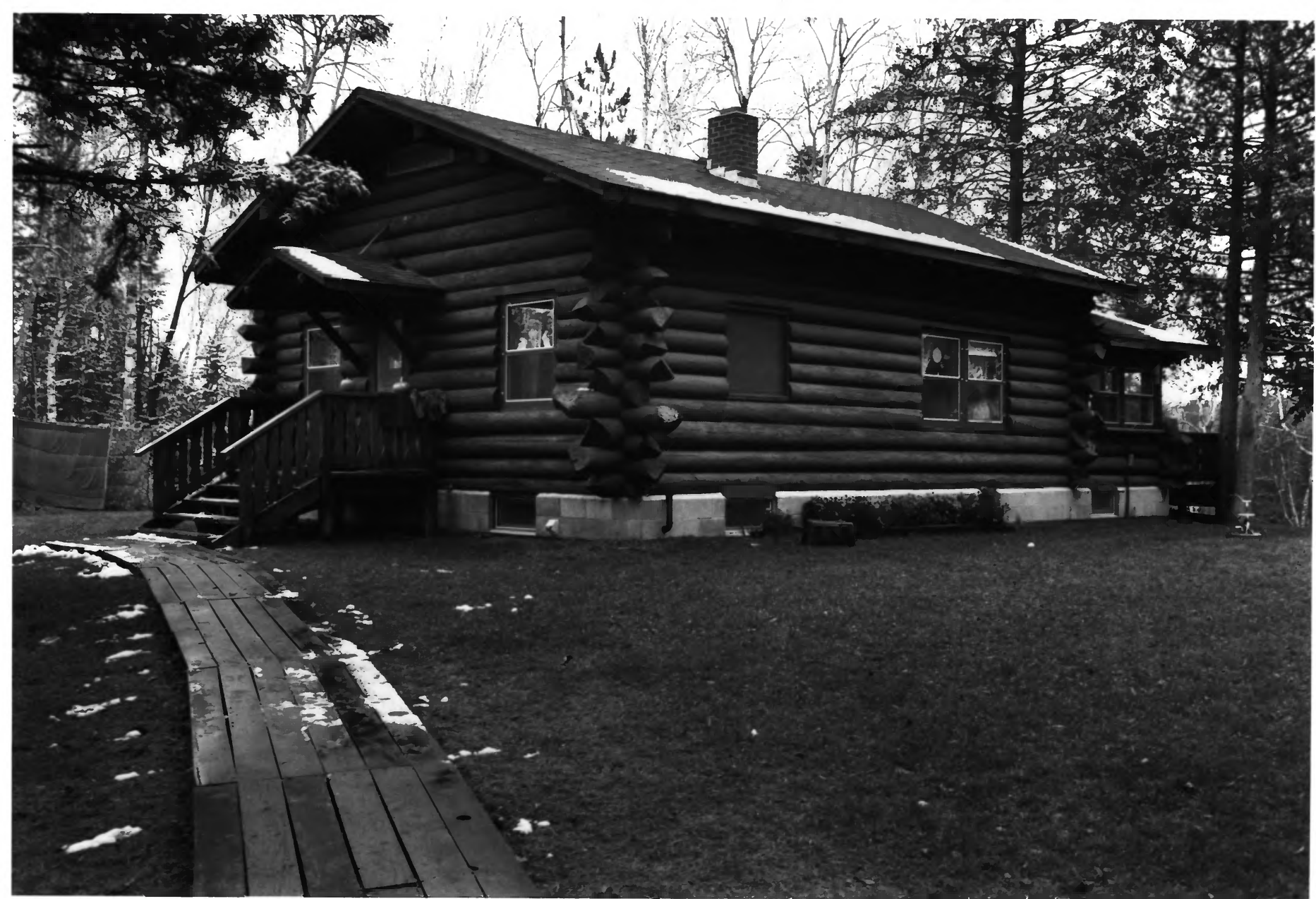
SCENIC STATE PARK - CCC / RUSTIC STYLE SERVICE YARD ITASCA CO., MN BLDG # 9 PHOTO I.D. 09120 # 10
