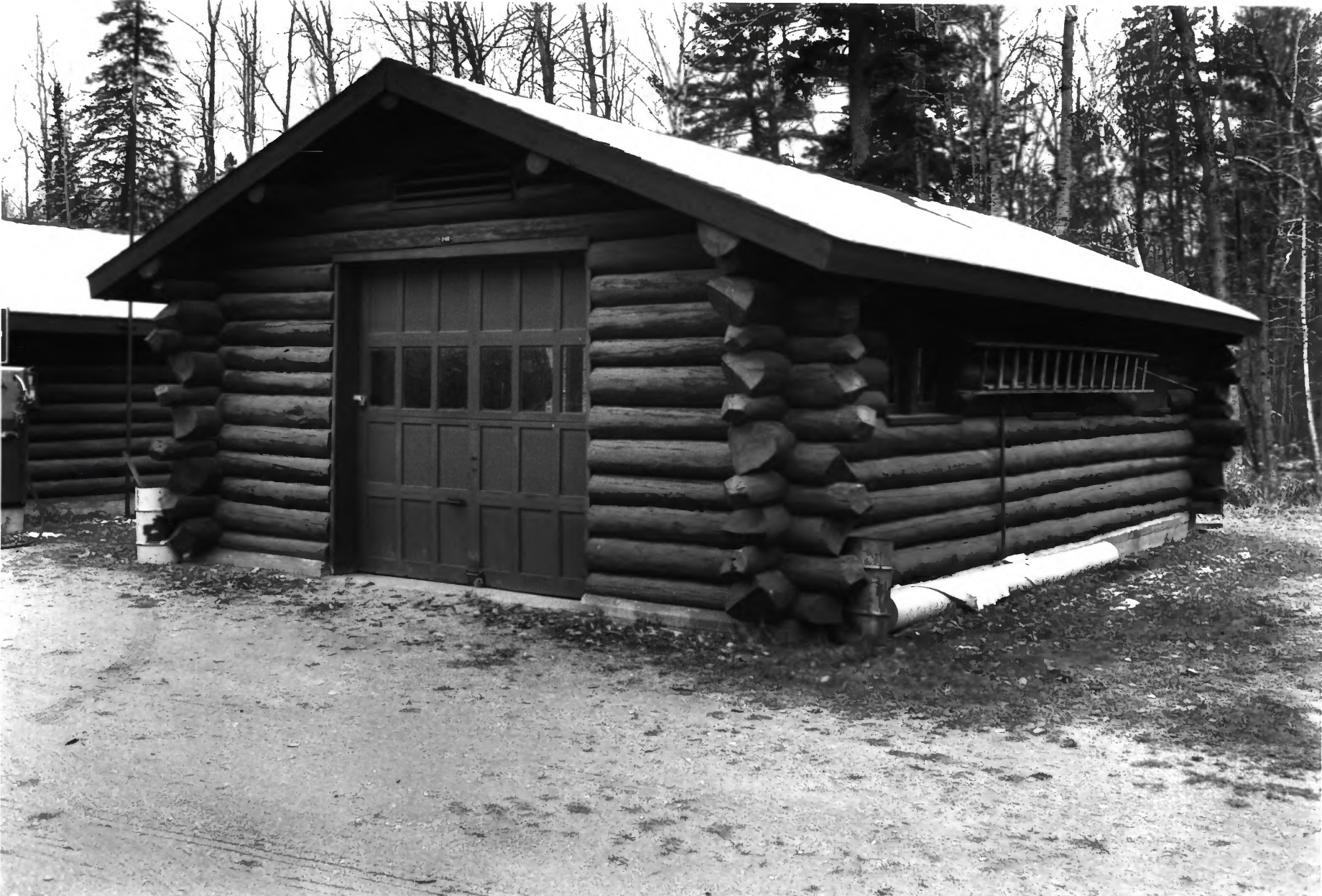
SCENIC STATE PARK - CCC / RUSTIC STYLE SERVICE YARD ITASCA CO., MN BLDG # 93 PHOTO I.D. 09120#4
