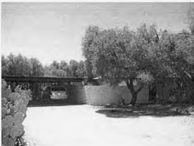
Photograph #3 View of east facade and carport looking southwest
