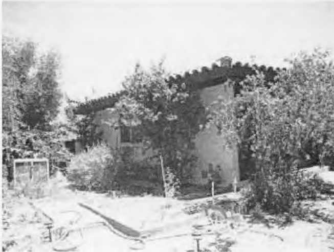
Photograph #5 View of west facade looking northeast
