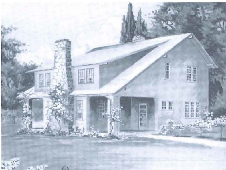
Fig. 9: Cement house No. 12, first published in the December 1911 issue of The Craftsman , features elements common to the style: ribbon windows, exposed rafter ends, two porches and an exterior wall chimney.
