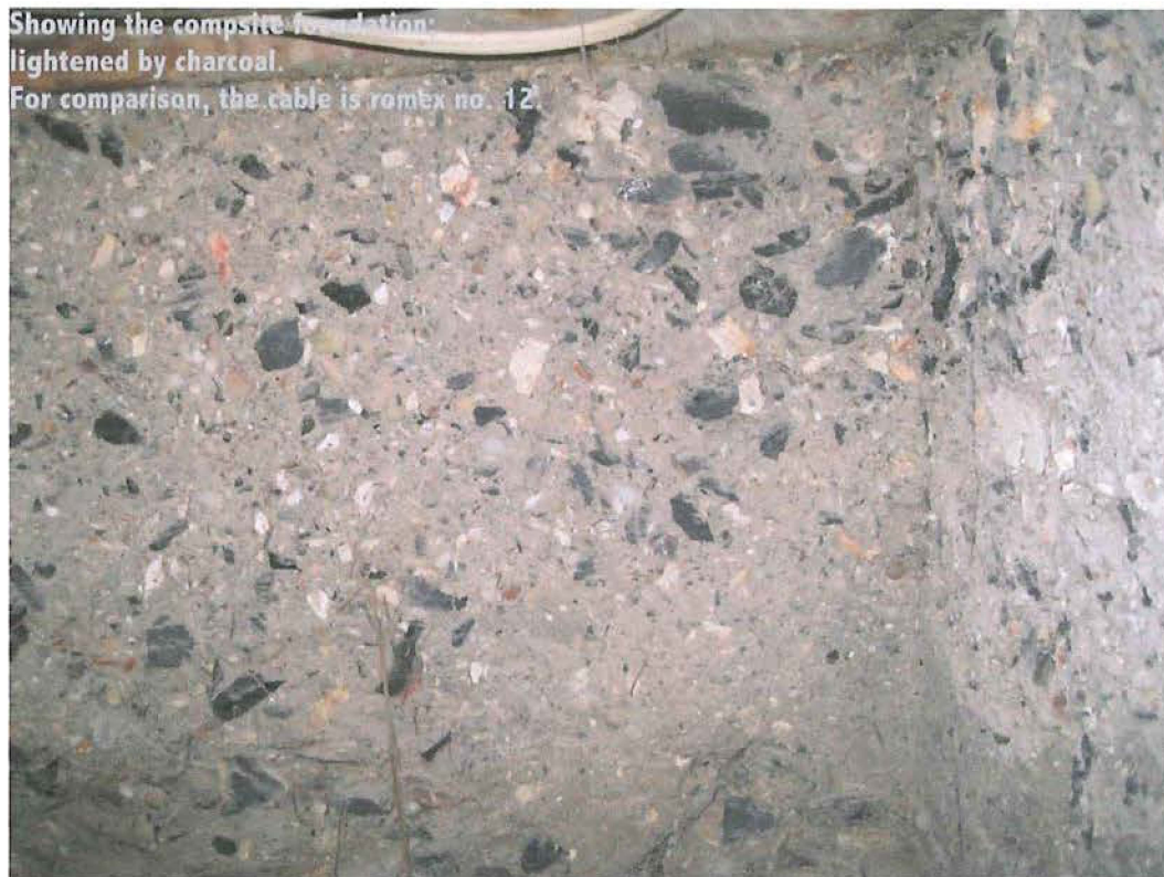
Fig. 7: lump coal as part of the aggregate in the foundation walls.
