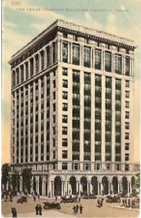
Figure 7. Texas Company Building, 1915, Houston, Texas Courtesy: Houston Metropolitan Research Center, Houston Public Library.
