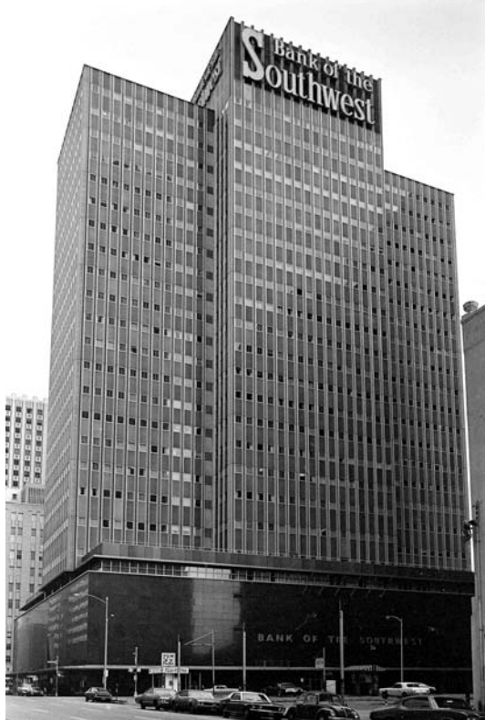
Figure 21. Bank of the Southwest Building (1956), Houston, Texas Courtesy Randy Pace postcard collection, Houston, Texas
