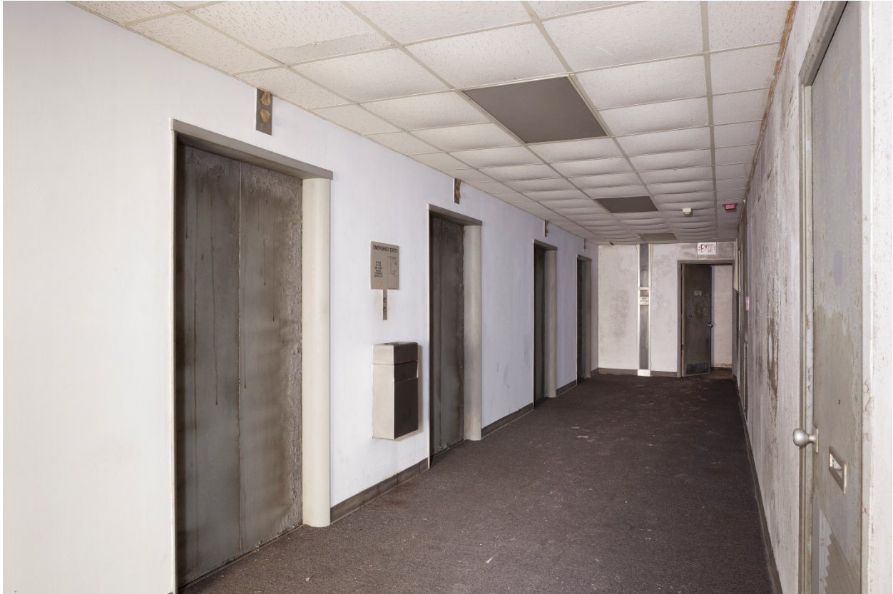
Photo #11 (TX_HarrisCounty_MelroseBuilding_photo_0011) Typical upper floor elevator lobby, camera facing north
