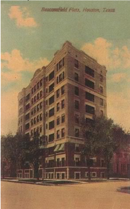
Figure 4. The Beaconsfield, 1910, 1700 Main, Houston, Texas Courtesy: www.houstonarchitecture.com
