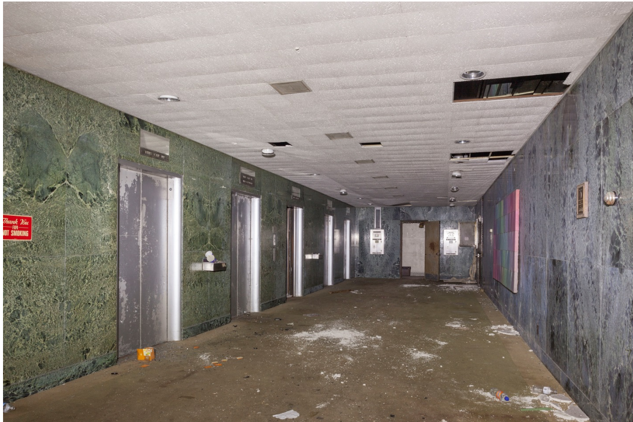
Photo #5 (TX_HarrisCounty_MelroseBuilding_photo_0005) Ground floor elevator lobby, camera facing north
