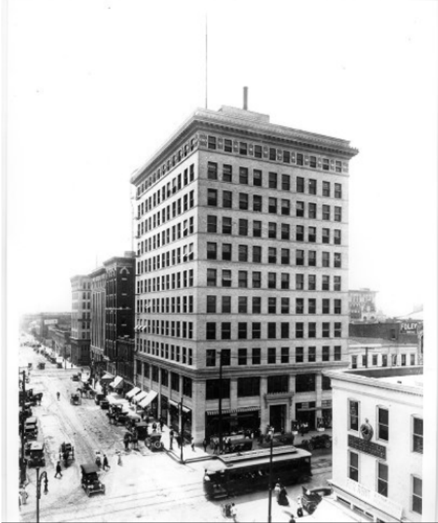
Figure 5. Scanlan Building, 1920, 405 Fannin, Houston, Texas Courtesy: Houston Metropolitan Research Center, Houston Public Library
