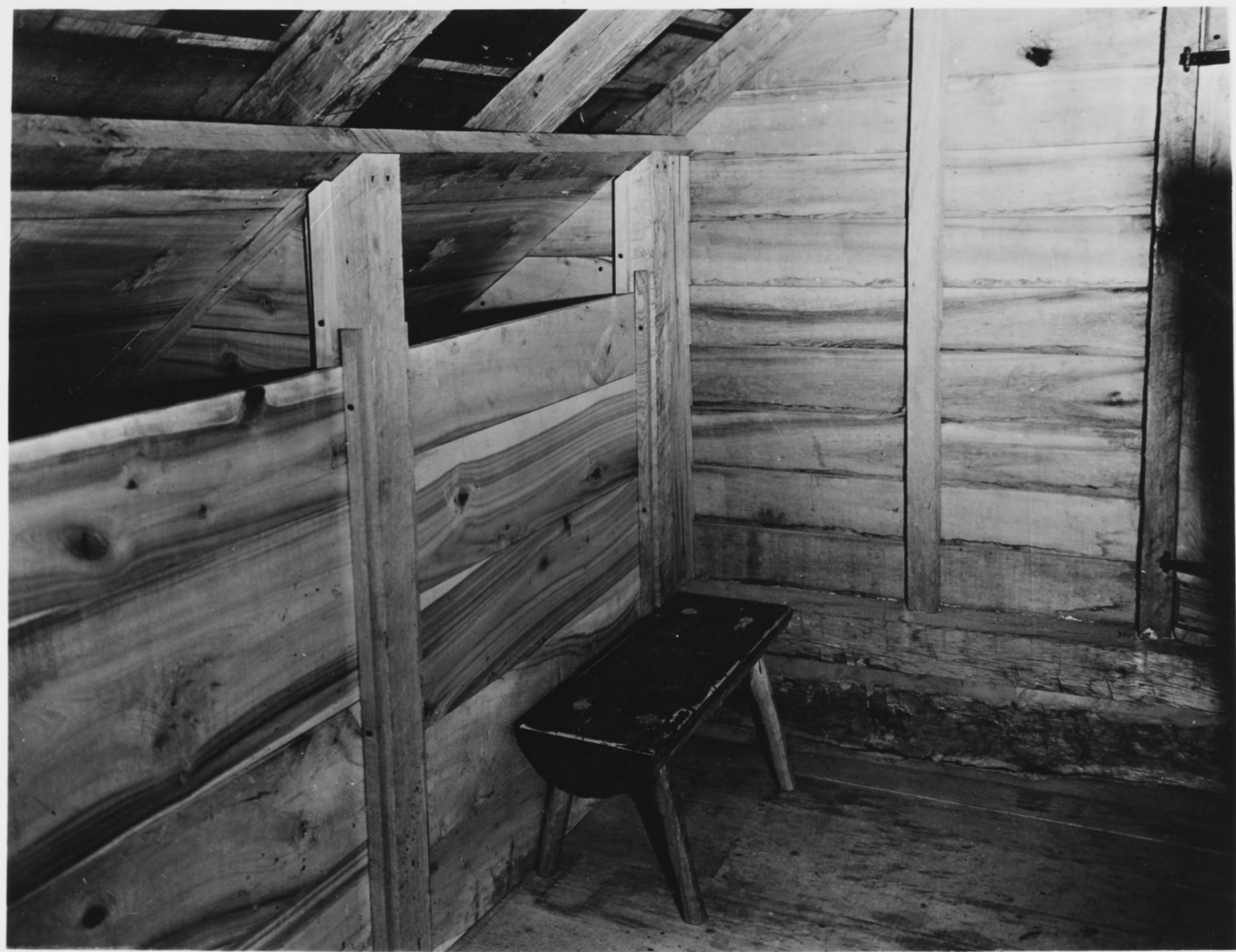
Corner of Third Floor of Mill. Storage Bins and Bench.
