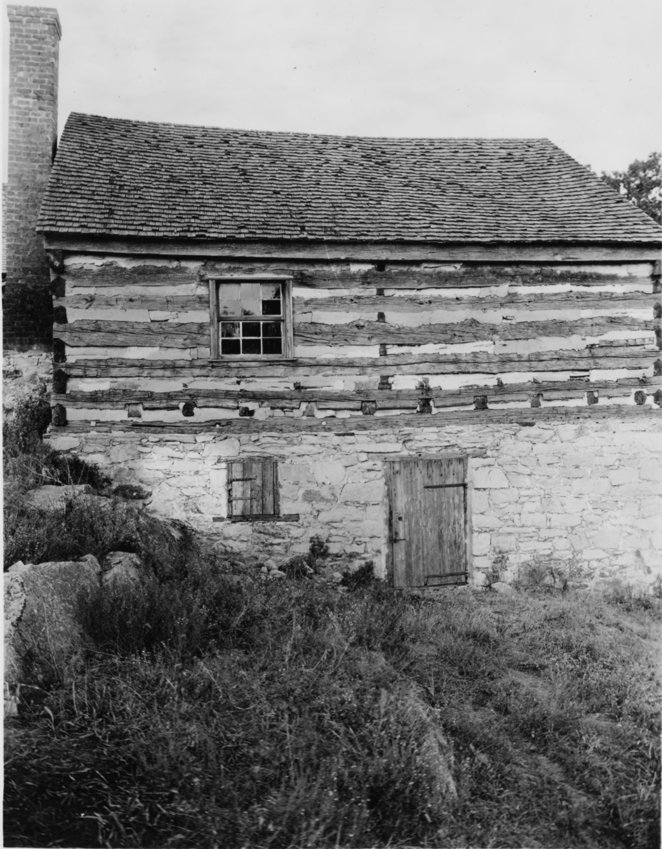
Side of Blacksmith Shop looking toward the House. The Door and Window in Stone Foundation were straightened and repaired in September 1938.
