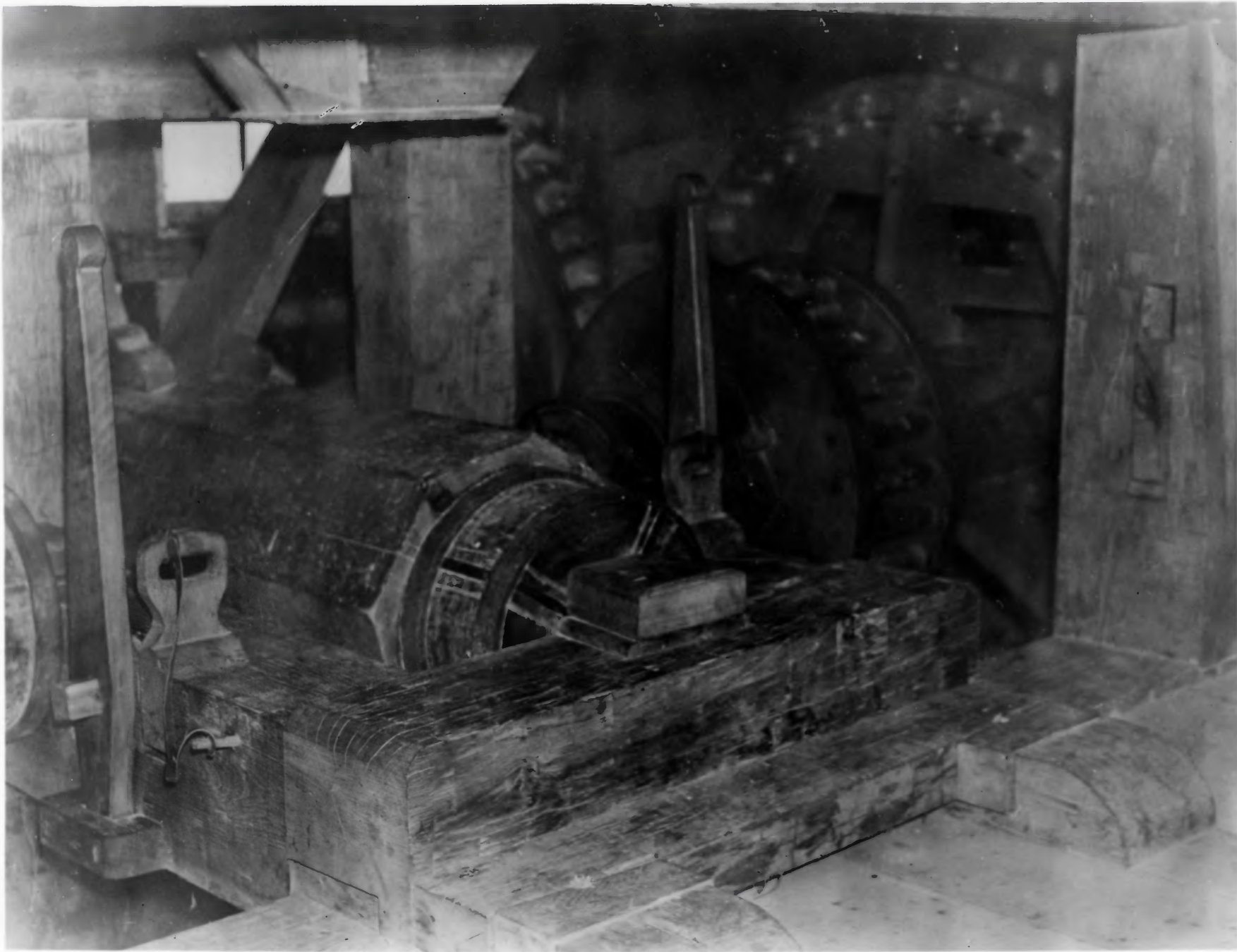
6. First Floor of Mill, showing Main Shaft and Corn Burr Machinery in motion. Note Levers for throwing Machinery in and out of gear.
