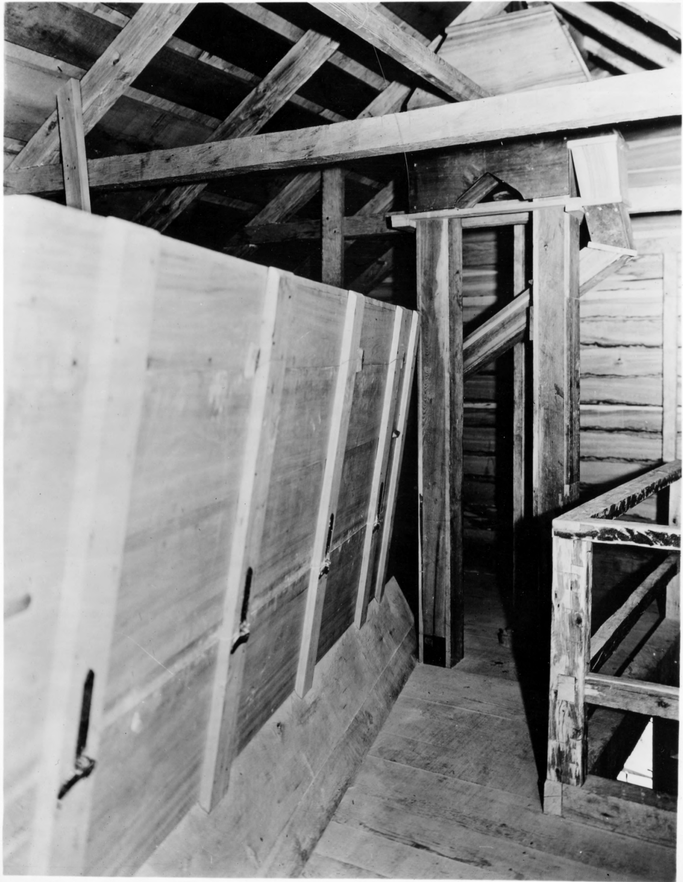
View of Interior of Mill Building, Third Floor. Bolting Chest with Door closed, Elevators and Chute.
