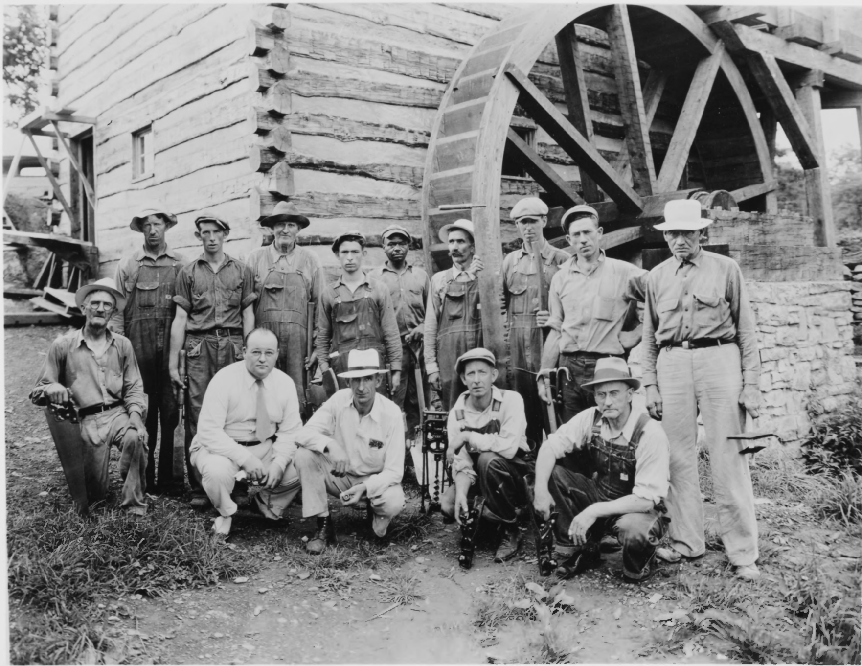
H. A. Kellar with Foreman, A. L. Oviatt, and a picked group of workmen, skilled in working with wood, stone, and iron, who did the most difficult parts of the restoration of the Race, Mill, Mill Machinery and Slave Cabin.
