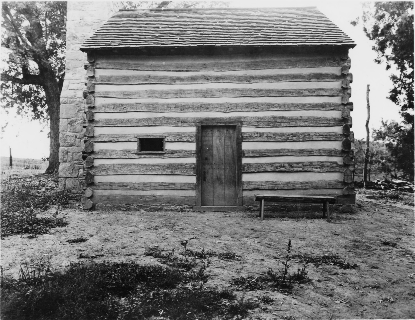
Exterior of Slave Cabin, east side, showing Entrance to lower floor. Note side view of stone chimney.
