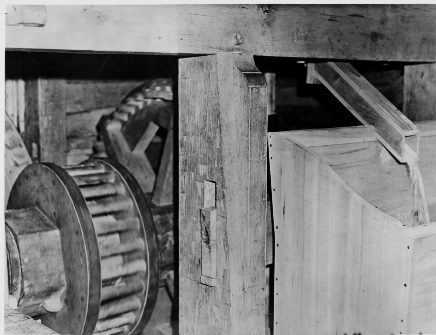
View of First Floor of Mill Building.
