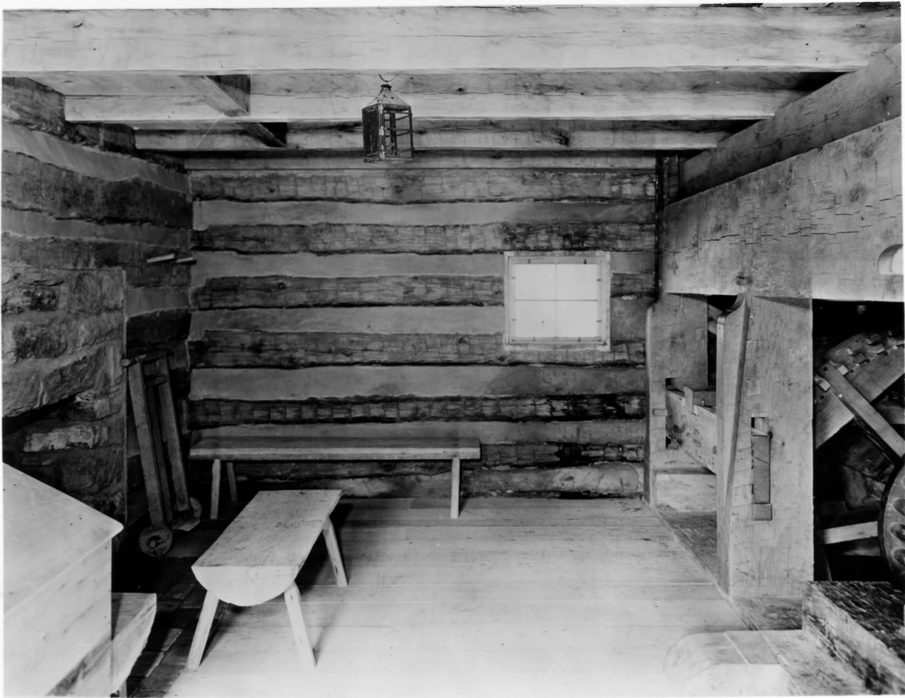
View of Interior of the Mill Building. Part of First Floor. Note Bran Bin on left and Mill Machinery on the right.
