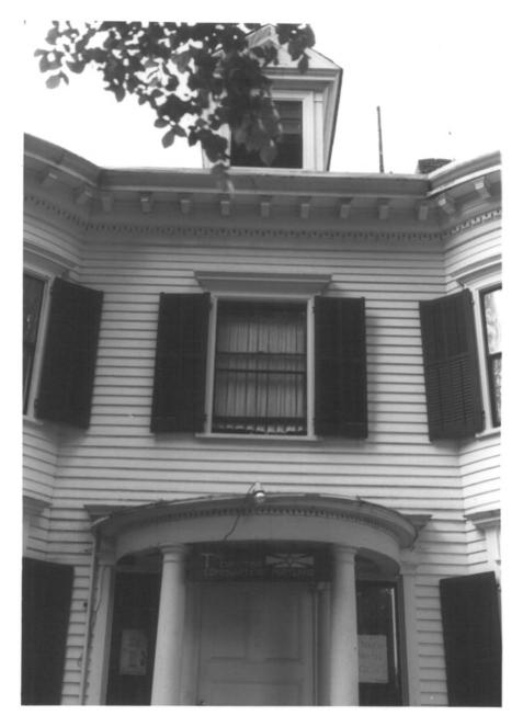
3 of 18 Detail of central bay of facade showing loss of balustrade from bowed portico.
