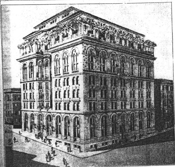
ELEVATION OF THE NEW Y. W. C. A. BUILDING IN COURSE OF CONSTRUCTION.
