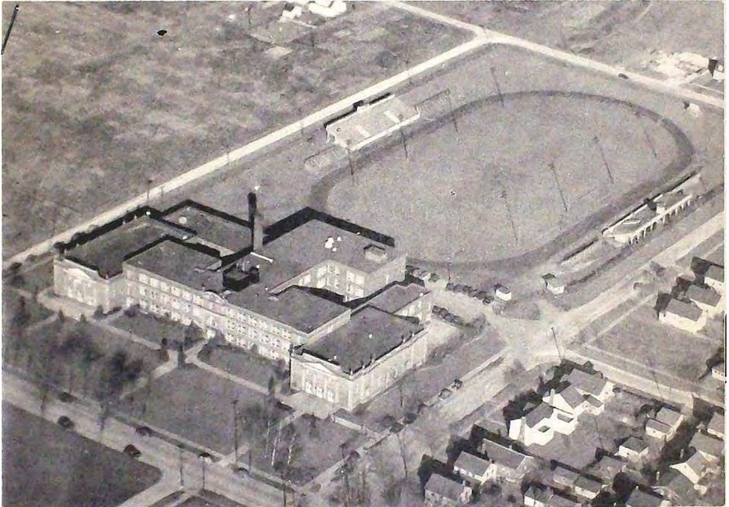
Payne High School, c. 1940, showing the school and athletic fields. Note also the vacant land to the north and east of the school. Available at nthistory.com .
