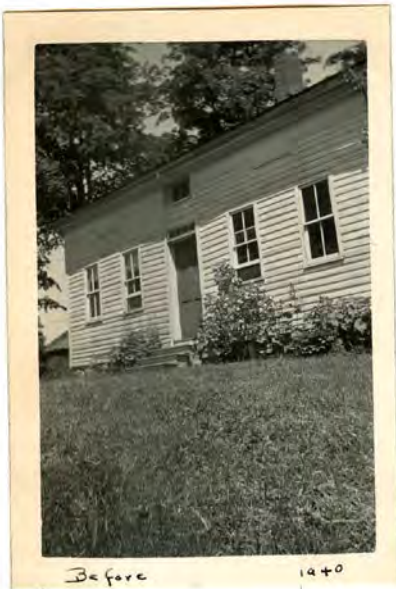
Description: View of south facade before the 1940s, before the Sornborger sisters did renovations. Notice the two-over-two windows.
