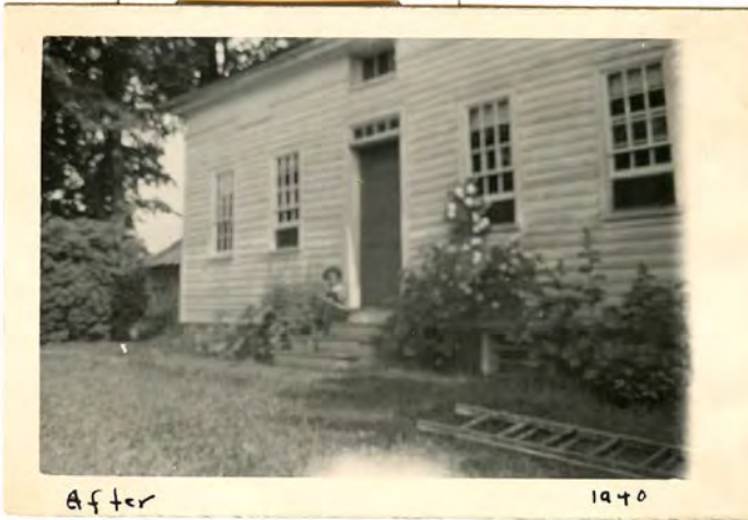
Description: View of south facade after the renovations in the 1940s. Notice the nine-over-six windows.
