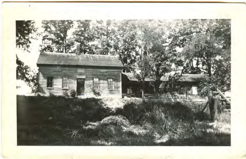
Description: View of south facade showing the house in disrepair
