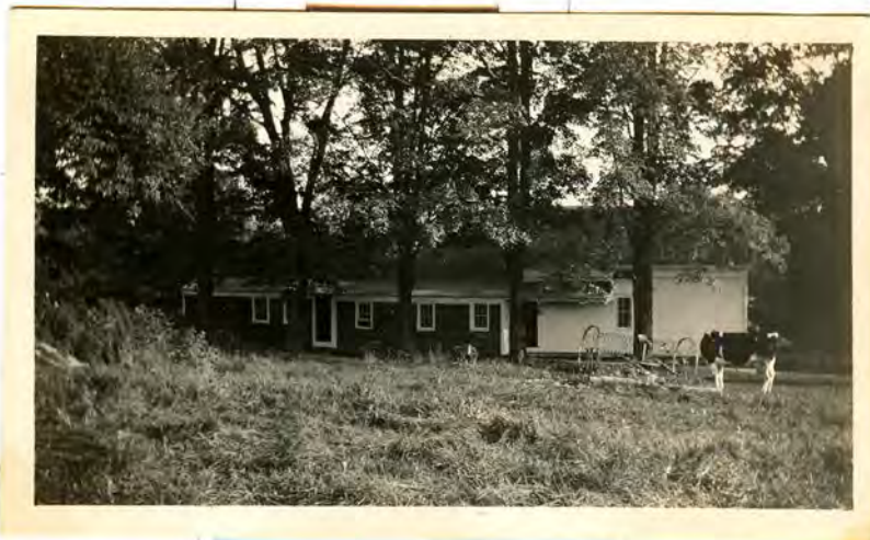
Description: View of the north facade after painting
