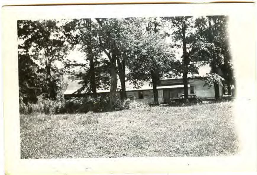
Description: View of the north facade before painting
