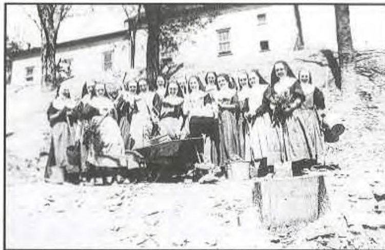
Constructing the Terrace Garden, 1930s
